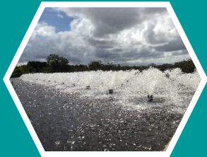
112 FILTRATION PLANTS with 136 intakes
