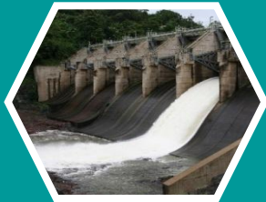
8 DAMS Owned by PRASA
