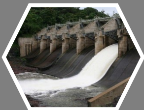
8 DAMS Owned by PRASA
