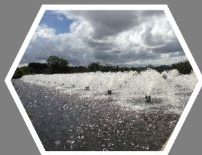
112 FILTRATION PLANTS with 138 intakes
