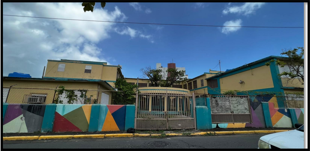
South View of the Property
