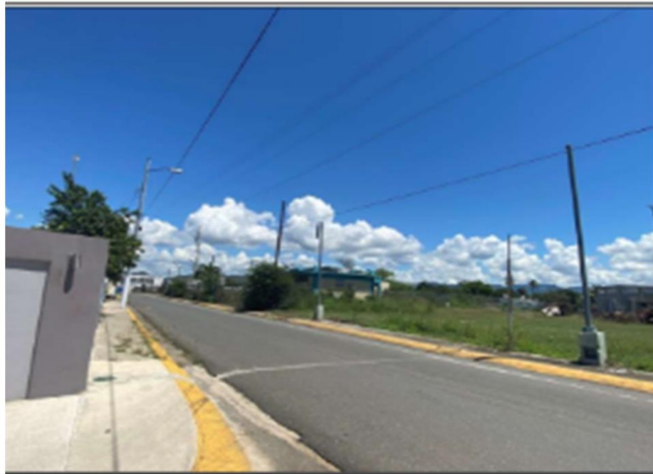
View west along Street 1. Subject at right side of street.
