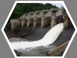
8 DAMS Owned by PRASA
