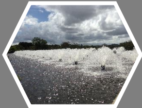
112 FILTRATION PLANTS with 136 intakes
