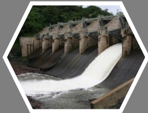
8 DAMS Owned by PRASA
