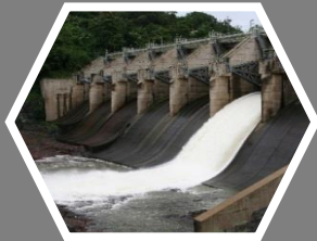
8 DAMS Owned by PRASA
