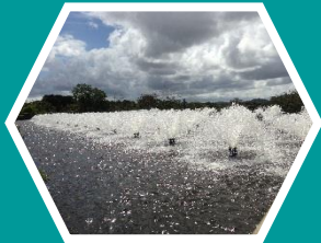
112 FILTRATION PLANTS with 136 intakes
