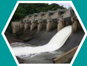
8 DAMS Owned by PRASA
