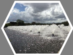
112 FILTRATION PLANTS with 136 intakes
