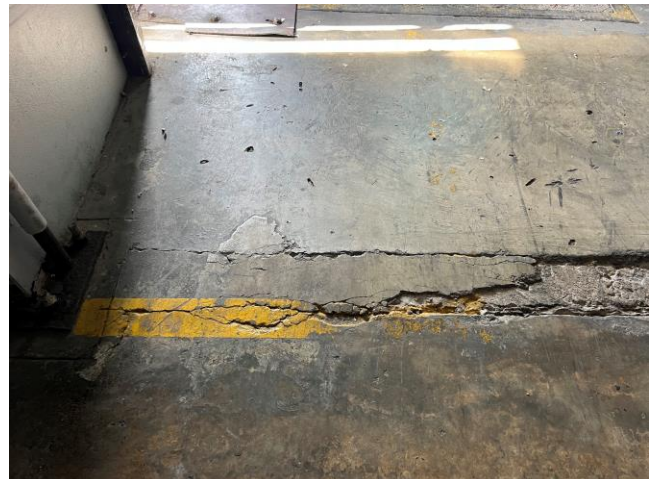
Room 1- Concrete Yellow Floor Lines with Lead Based Paint
