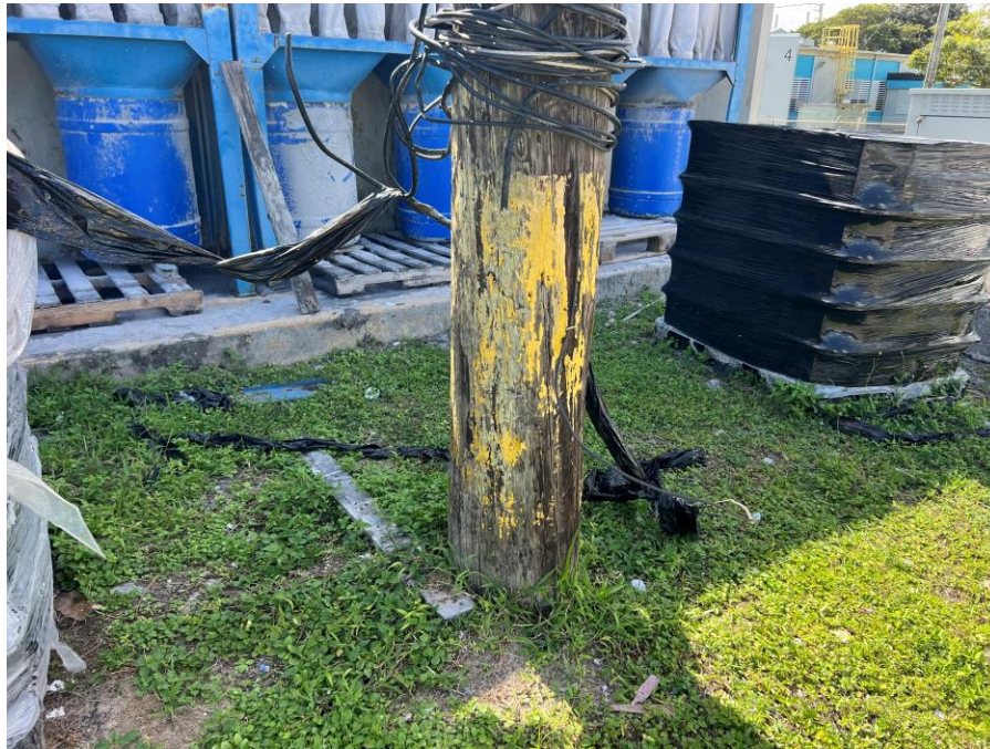
Exterior – Side B- Wood Electric Pole with Lead Based Paint
