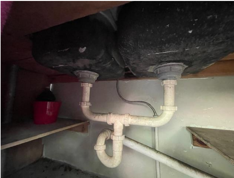
Black Mastic under sink with Asbestos
