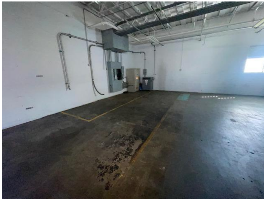
Room 1- Concrete All Yellow Floor Lines with Lead Based Paint
