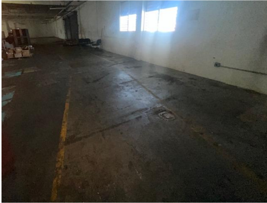
Room 1- Concrete All Yellow Floor Lines with Lead Based Paint
