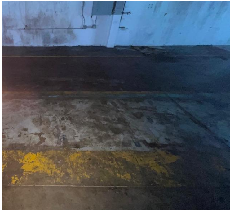
Room 1- Concrete All Yellow Floor Lines with Lead Based Paint
