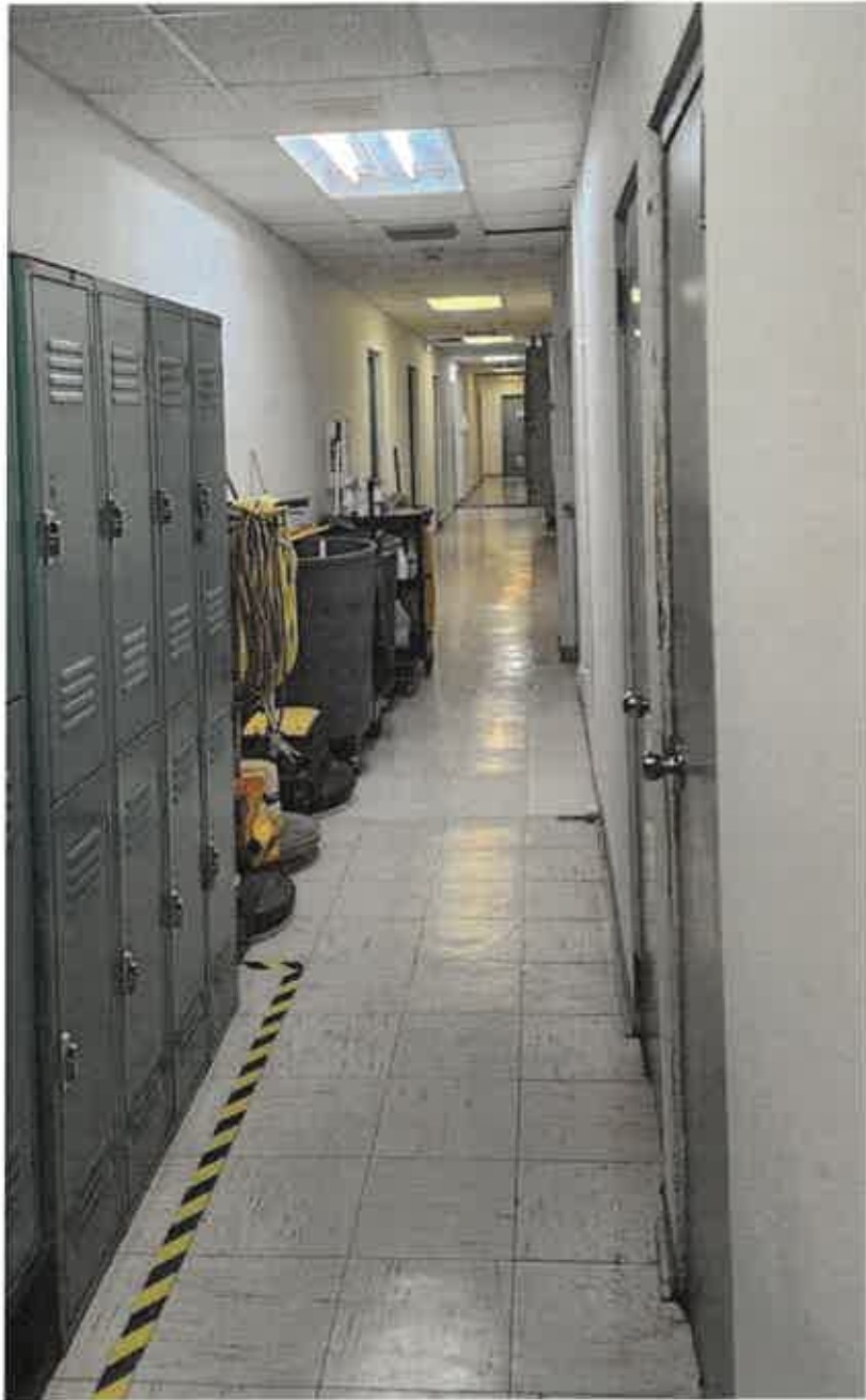
Main Entrance Foyer, Hallway Floor Vinyl Tile, 800 ft 2
