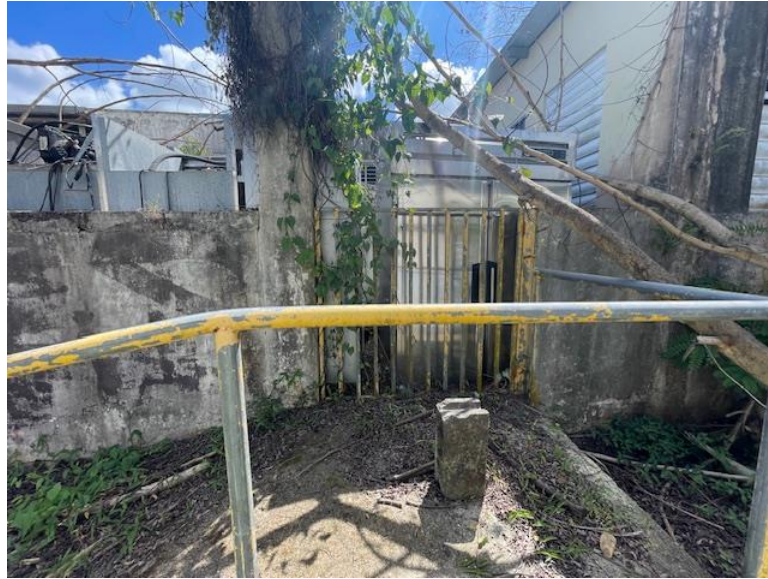
Exterior- Side D- Metal Gate with Lead Based Paint
