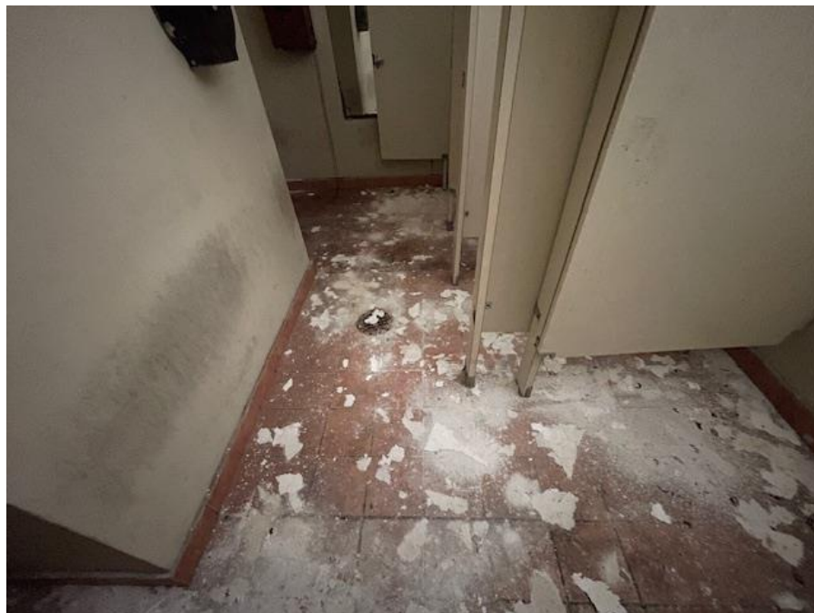
Bathroom 5- Ceramic Floor Tiles & Baseboards Tiles with Lead Based Paint
