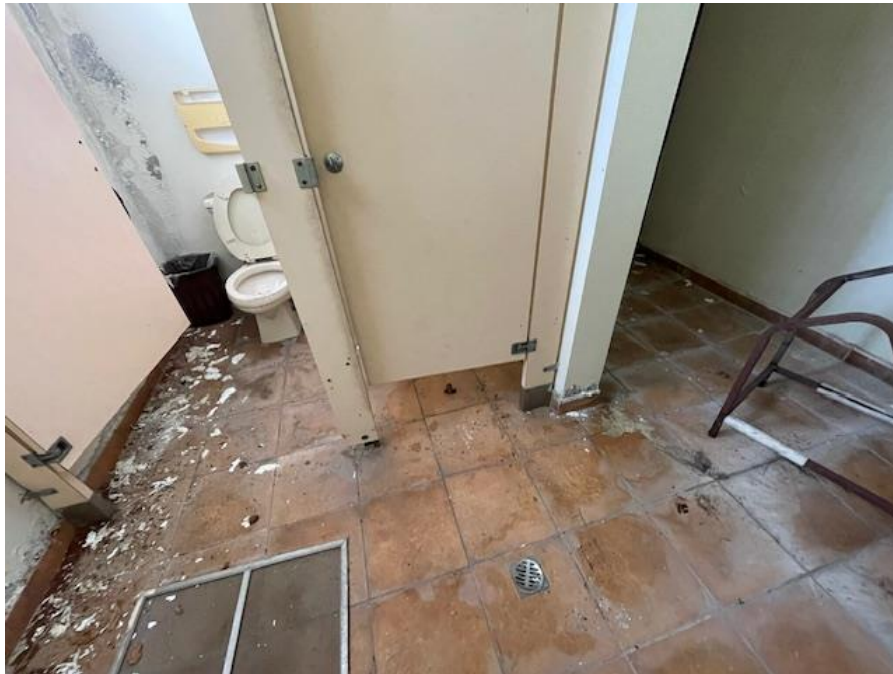
Bathroom 2- Ceramic Floor Tiles & Baseboards Tiles with Lead Based Paint
