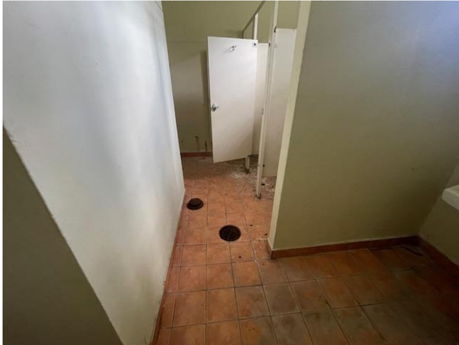
Bathroom 7- Ceramic Floor Tiles & Baseboards Tiles with Lead Based Paint
