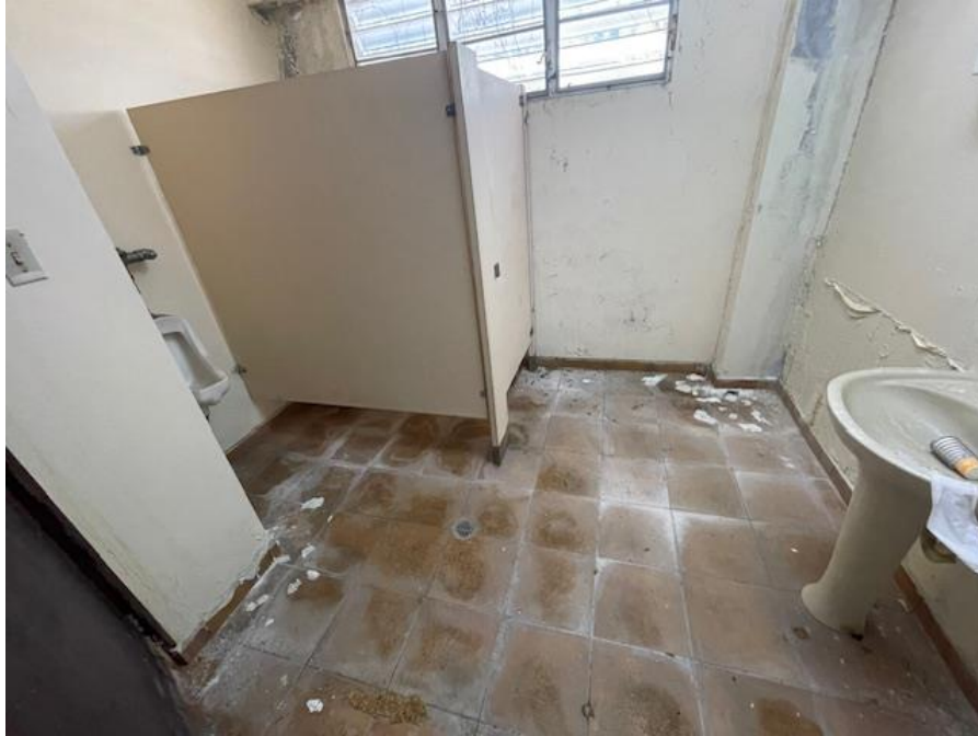
Bathroom 3- Ceramic Floor Tiles & Baseboards Tiles with Lead Based Paint
