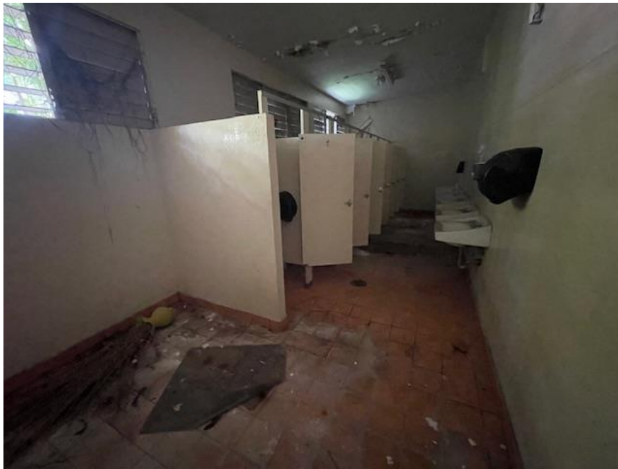
Bathroom 6- Ceramic Floor Tiles & Baseboards Tiles with Lead Based Paint
