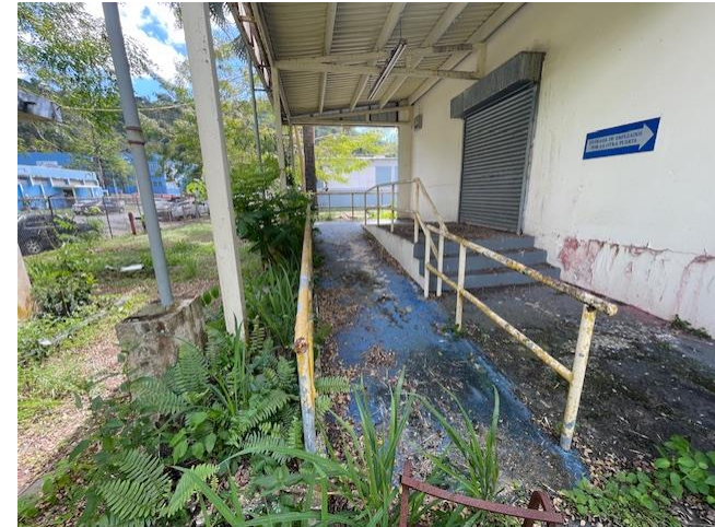
Exterior- Sides - Metal Handrails with Lead Based Paint
