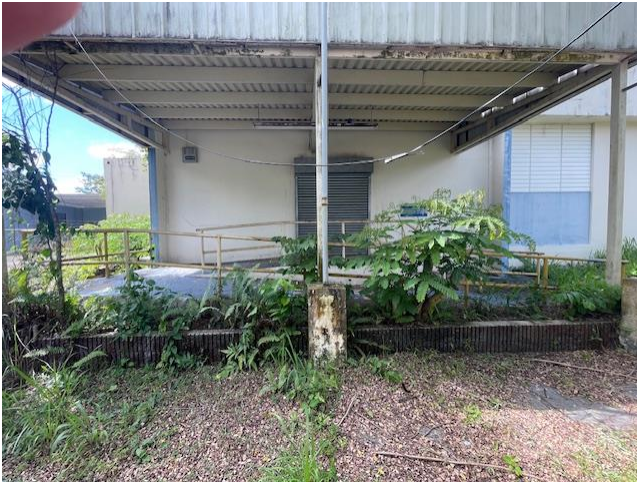
Exterior- Sides - Metal Handrails with Lead Based Paint
