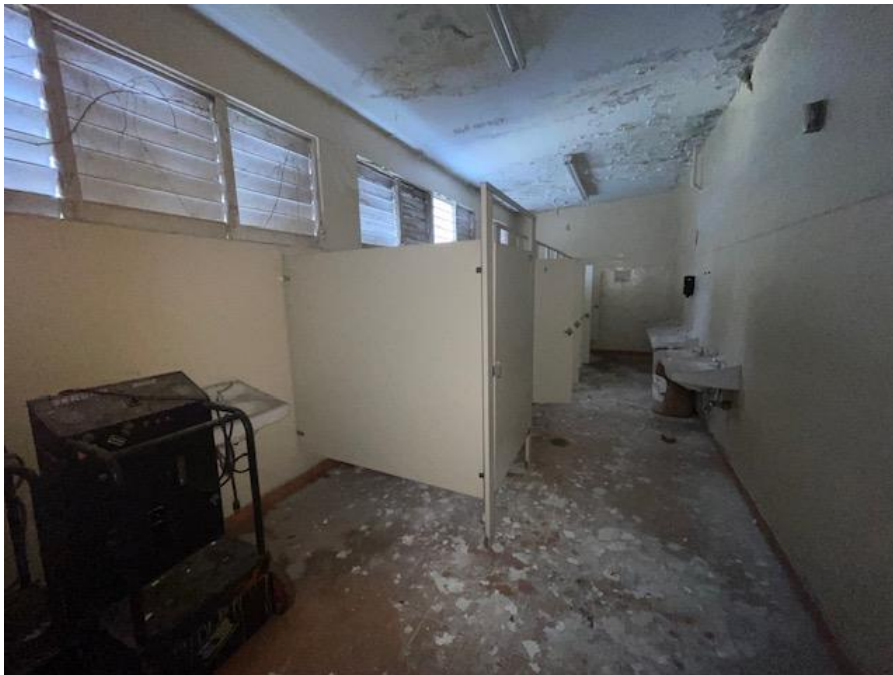
Bathroom 4- Ceramic Floor Tiles & Baseboards Tiles with Lead Based Paint
