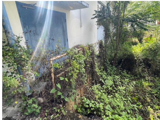
Exterior- Side D- Metal Gate with Lead Based Paint
