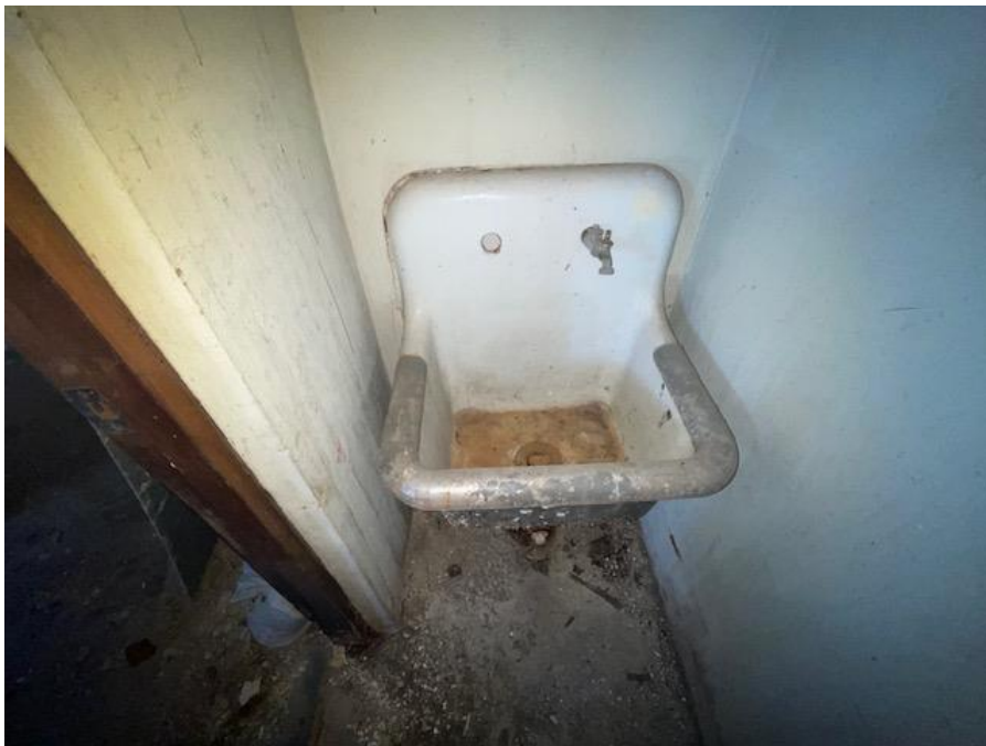
Janitor 2- Ceramic Sink with Lead Based Paint
