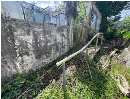
Exterior- Side D- Metal Gate with Lead Based Paint
