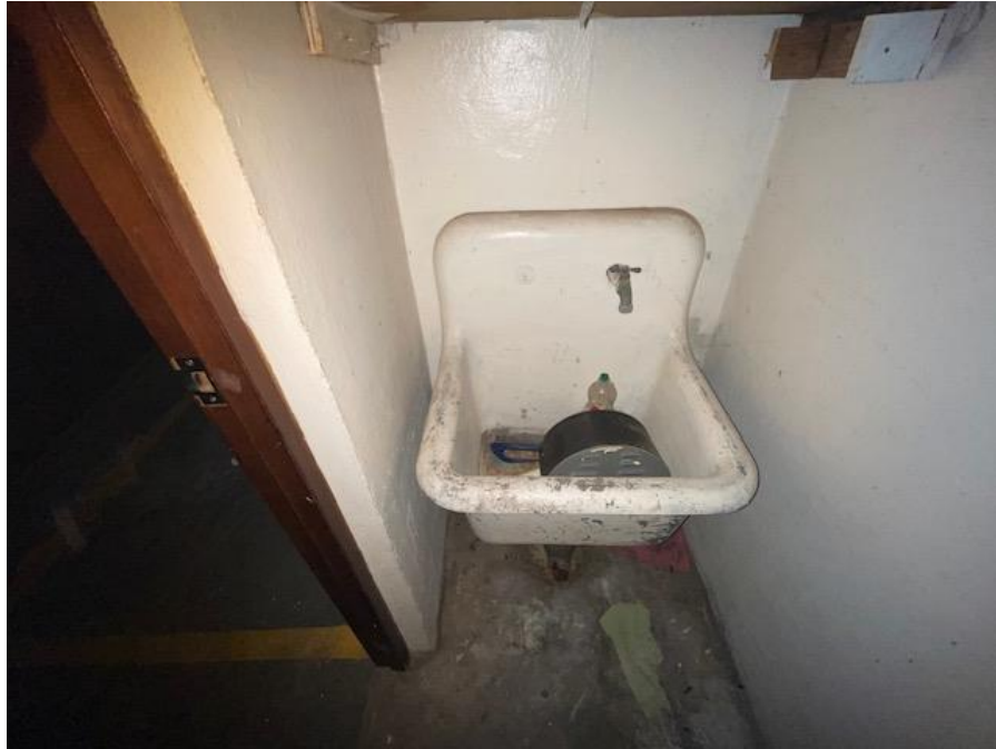
Janitor 1- Ceramic Sink with Lead Based Paint
