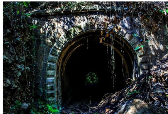
Guaniquilla old train tunnel
