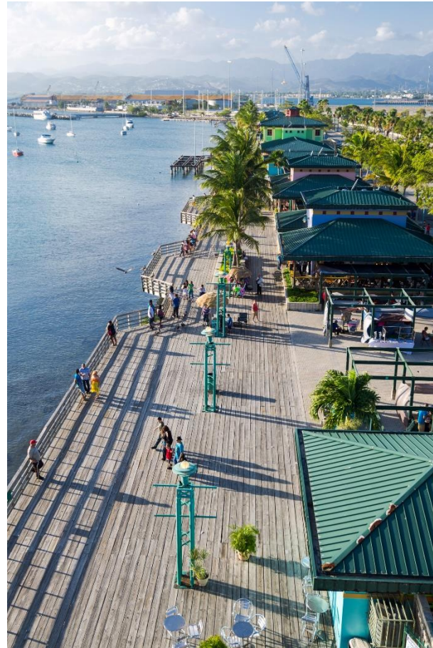
La Guancha in Ponce is one of the most visited outdoor recreation facilities. It has been severely impacted by the earthquakes that are still affecting the south of Puerto Rico.
