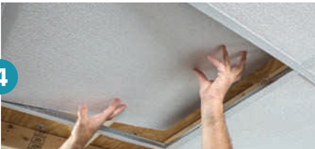
Install ceiling panels
