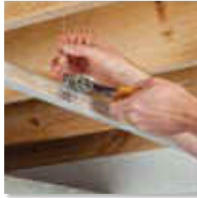
2 Suspend main beams with hanging hardware
