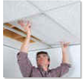
4 Install ceiling panels
