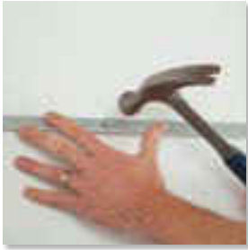
1 Install wall moldings
