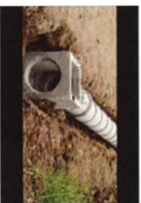
Precast Installation at Parking
