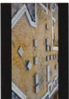
Foundations near completion at area A
