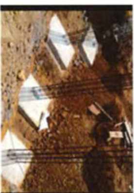
Spread footings near Mechanical Room 104
