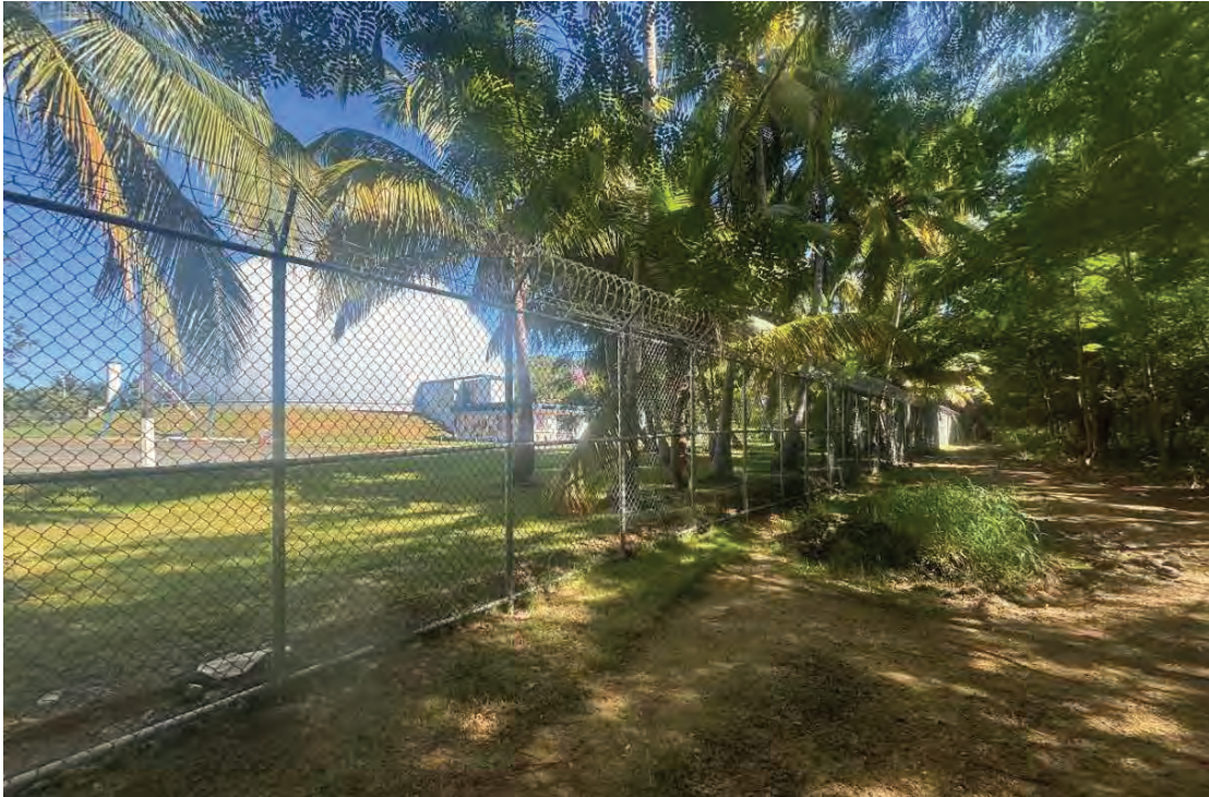
Photo 5. General view of BONUS reactor facility from outside fence (taken December 2025).
