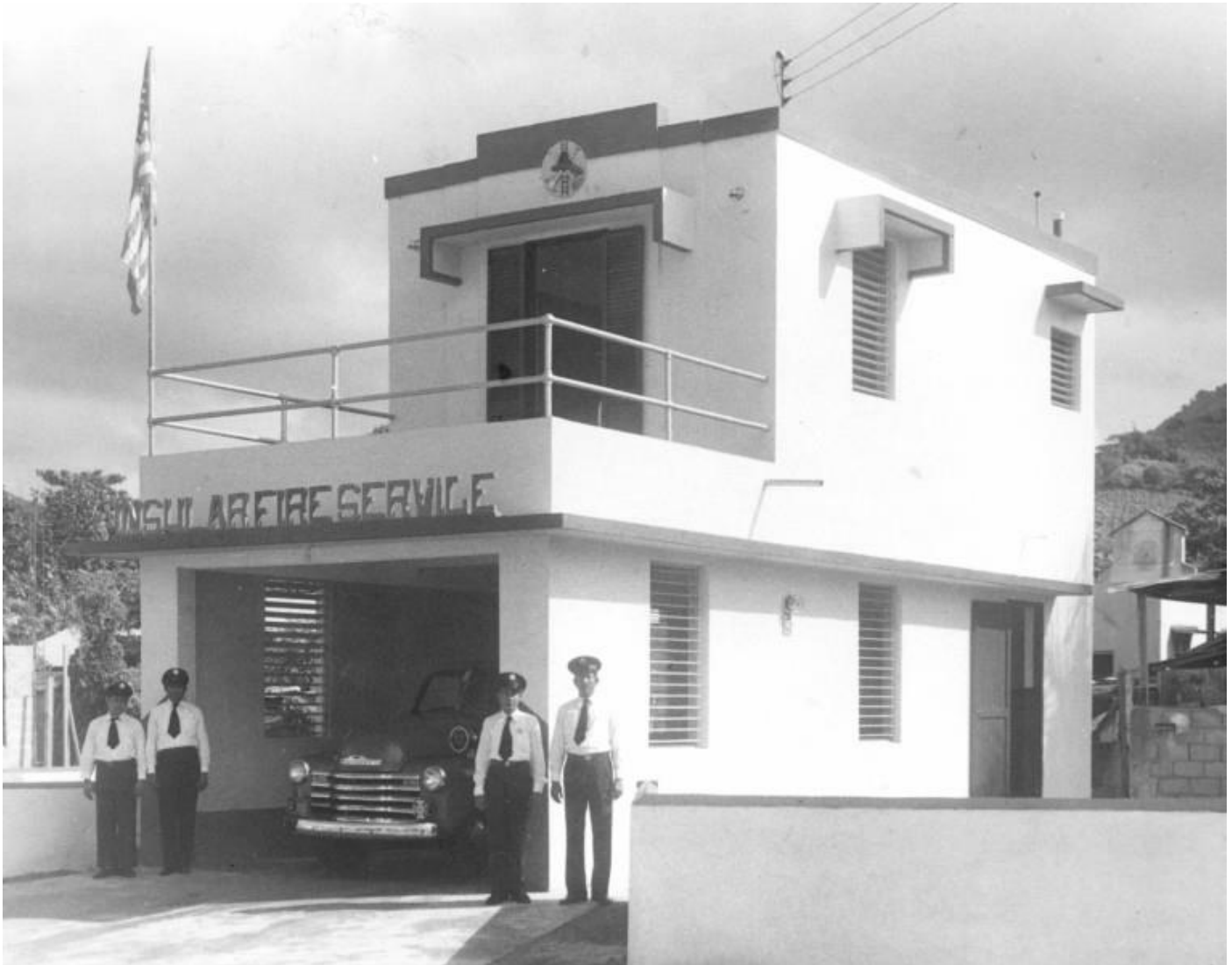
Fig. 23: Prototype A at an unidentified location. Source: Cuerpo de Bomberos de Puerto Rico
