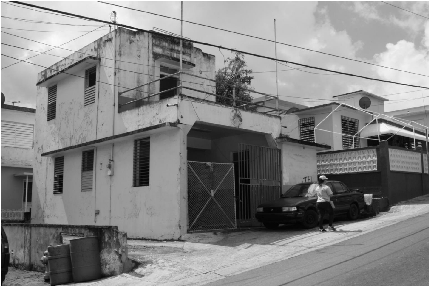
Fig. 27: Aguas Buenas firehouse today. Photo: Guillermo Marrero, 2011
