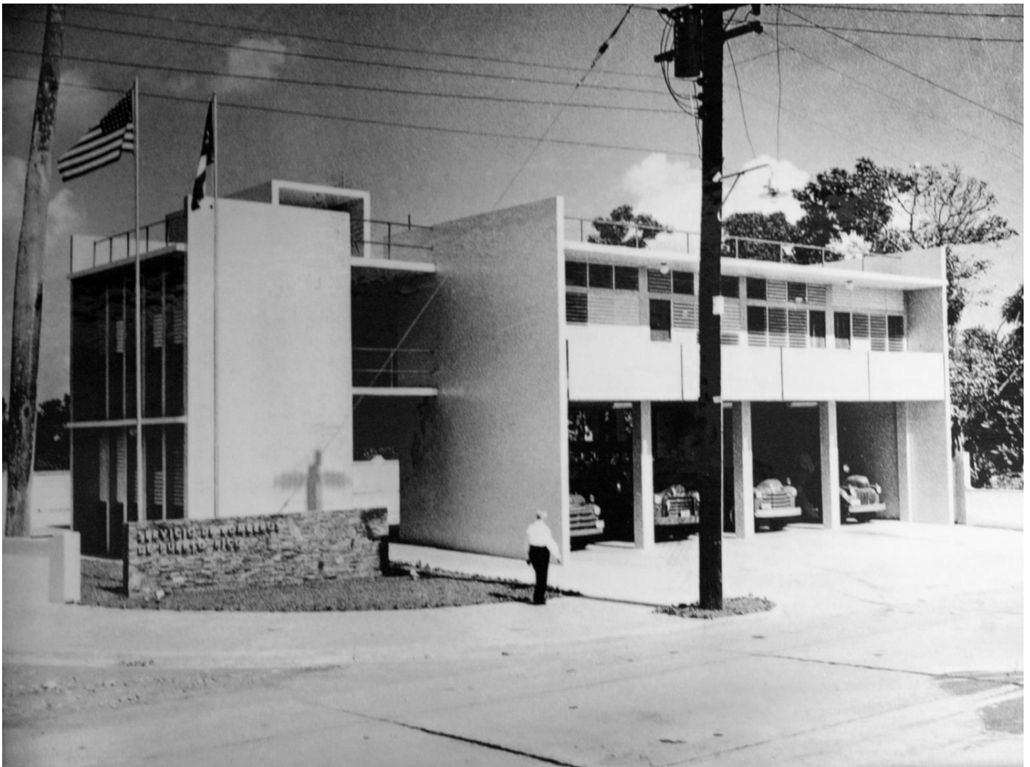
Fig. 26: Modern Fire Station built in Hato Rey, 1952. The iconic structure appeared in the educational comic book "Fuego" published by Puerto Rico Fire Service in 1959. Source: Photo after 1952
