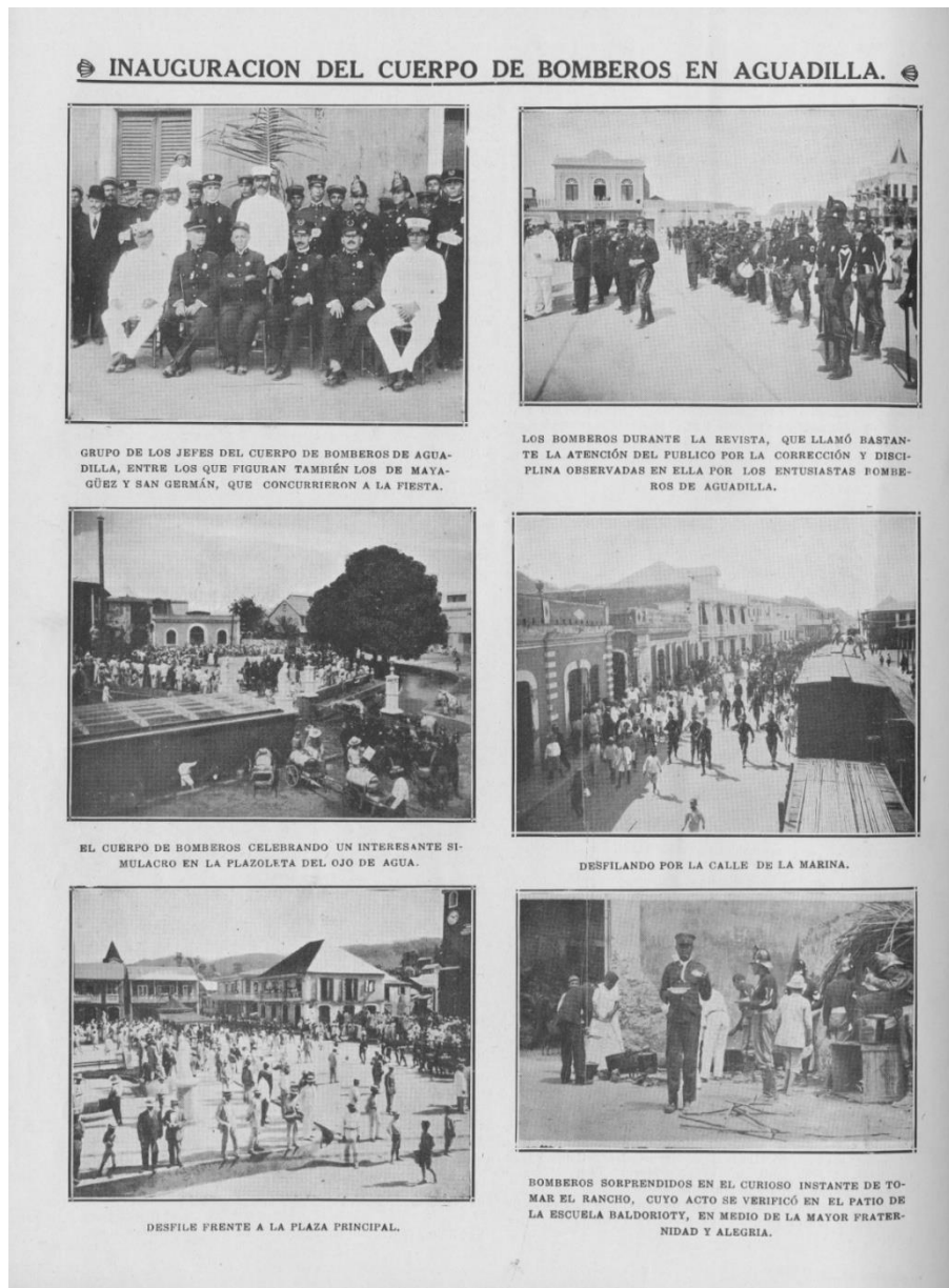
Fig. 2: Events held during the inauguration ceremony of the Fire Station in Aguadilla.
