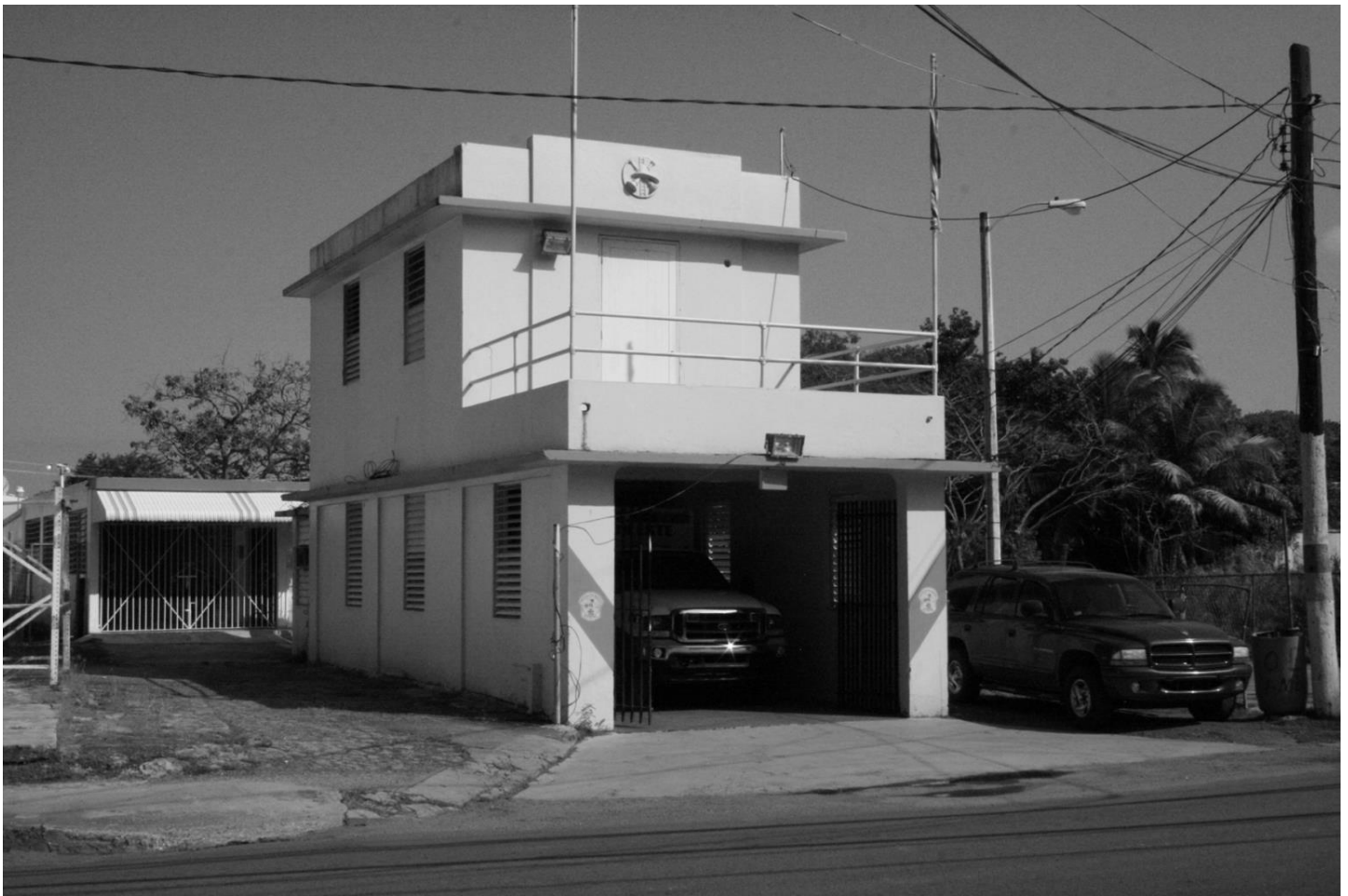
Fig. 28: Ceiba's fire station today. Photo: Guillermo Marrero, 2011
