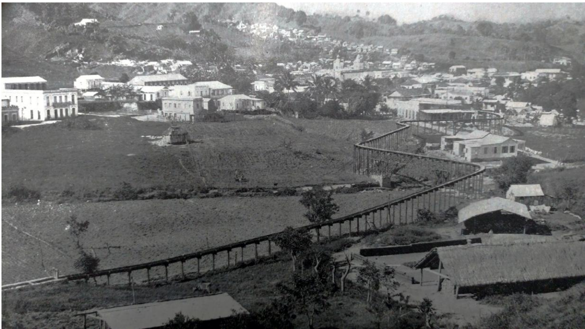
Figure 16. The aqueduct system in Utuado. 87
