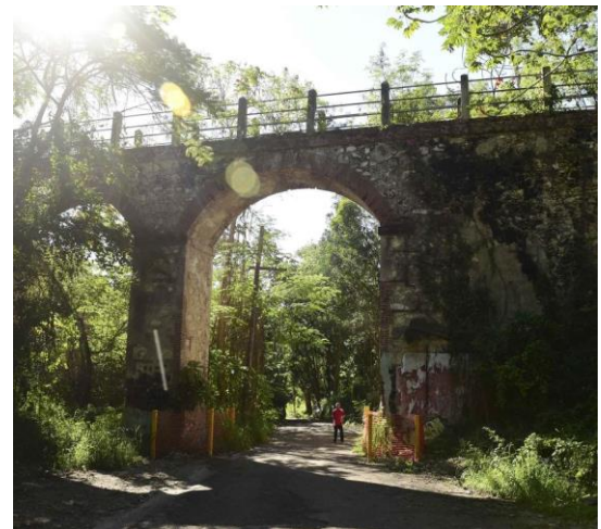
Figure 20. Above, the 1875 Lubelza's plan for the Murallón de la Cantera . Below, a partial view of the extant resource. The water ran in the canal atop, while the elevated arcs allow the downpour flow and folks transit. From its top, the structure is about fifty-feet high. (Juan Llanes Santos, photographer)
