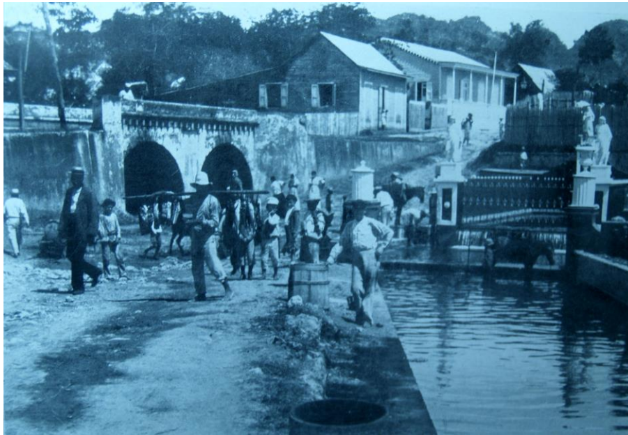
Figure 15. The “Ojo de Agua” in Aguadilla. The three statues mark the masonry box built around the spring, which access was blocked by a set of elaborated iron fence. Just below the spring fountain is the public bathing pool, and at a lower level in the foreground is the animal pond. An “aguador” poses at the center of the photo. Water was carried by the “aguadores” to private homes at a rate of ten cents per bucket. To the left, is the 1865 Puente de la Reina Bridge. 84
