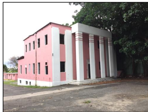
[Figure 45] Public health unit, Santurce (not in use) / 2017
