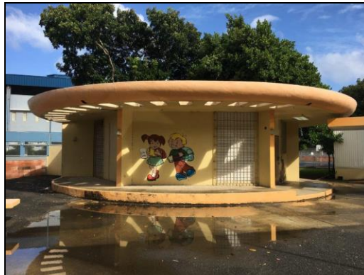
Figure 21 JOHN F. KENNEDY ELEMENTARY SCHOOL (Levittown), Toa Baja. Cylindrical feature housing the kindergarten. Architect: David P.C. Chang. Photo: Jorge Rigau
