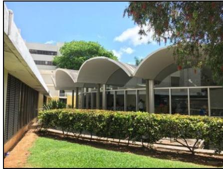
Figure 34: SAN JUAN MEDICAL CENTER, San Juan. Cafeteria with vaulted arches in concrete and extended glazing. Architects: Isadore and Zachary Rosenfield. Photo: Jorge Rigau
