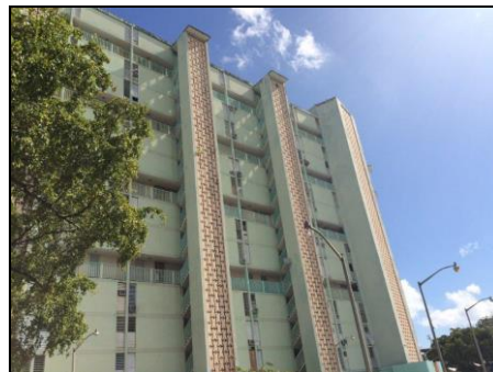
Figure 33: CONDOMINIOS QUINTANA, Hato Rey. Screened stairs and alternating hallways grant depth to the façade. Architects: Reed, Basora y Menéndez. Photo: Jorge Rigau
