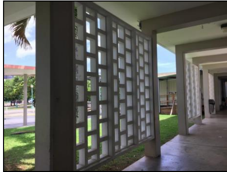
Figure 29: SAN JUAN MEDICAL CENTER, San Juan. Cement screens at breezeways. Architects: Isadore and Zachary Rosenfield. Photo: Jorge Rigau
