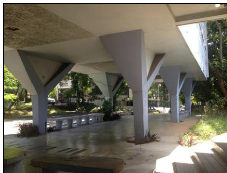
Figure 14: STUDENT DORMITORIES, EVANGELICAL SEMINARY, Río Piedras Recreation lobby, including sculptural/trapezoidal columns, ceiling texture treatment, and paving patterned in hexagons. Architects: Horacio Díaz and Enrique Soler Cloquell. Photo: Jorge Rigau
