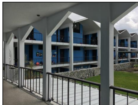
Figure 39: STUDENT CENTER, CATHOLIC UNIVERSITY, Ponce. Hallways facing courtyard, articulated from the ground. Architect: Carl Brunner. Photo: Jorge Rigau
