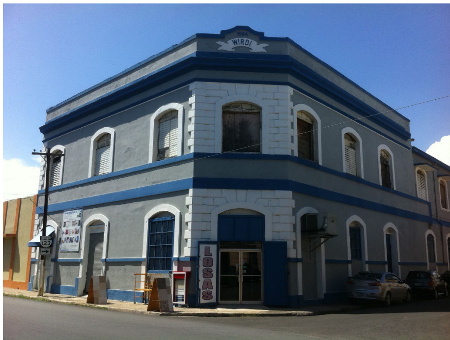
Figure 39. Two buildings designed by A. B. Wiechers in Playa. Above, the 1914 meat and milk depot at the corner of Calle Virtud and Alfonso XII. Below, the 1917 warehouse at Calle Comercio.
