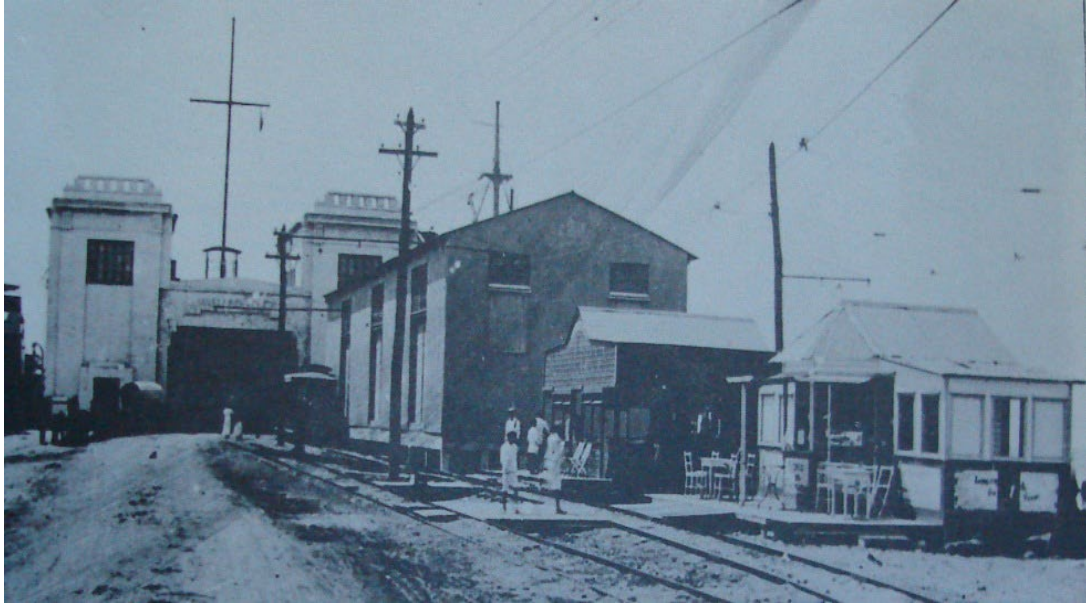
Figure 21. Port at Peñoncillo. The road built to reach it, had it railroad and trolleys connections 62
