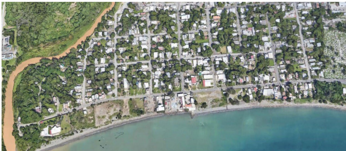
Figure 36. Above, the 1936 aerial photo of Los Meros. Below, a Google map of the same area. The photos show the occupation of Los Meros started as part of the 1940's policies of land distribution. Matilde River (on the left) is Playa de Ponce's official western boundary since 1955. The 1911 Cemetery shows on both pictures on the extreme right. The row of houses in the 1936 photo, were front-beach-villas of some of Ponce's bourgeoisie, no longer at the site.
