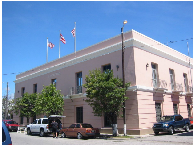
Figure 8. Partial view of the Aduana, the oldest custom building in continuous use in Puerto Rico.
