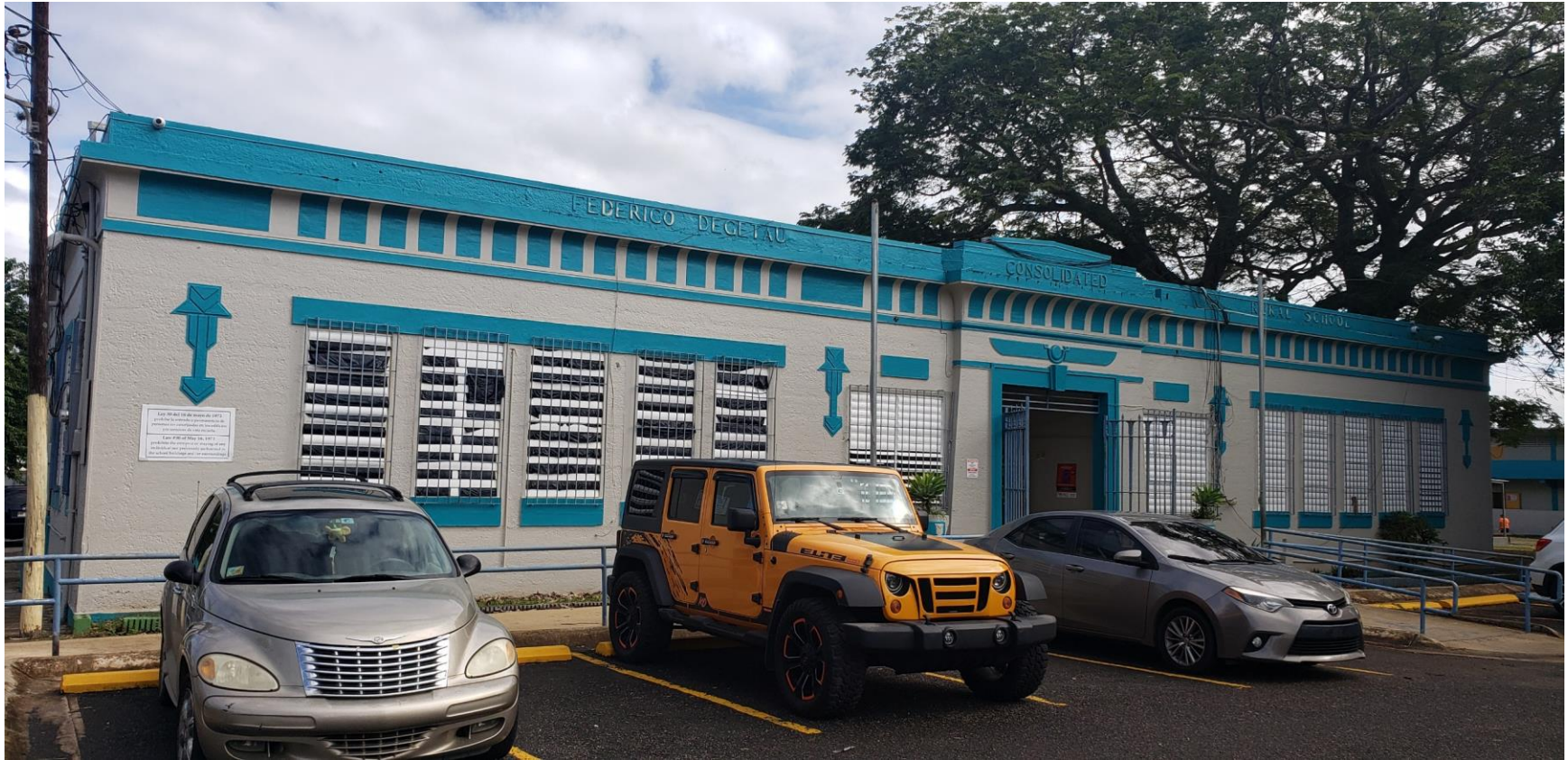
PR_Arecibo_Federico Degetau Consolidated Rural School_0001
