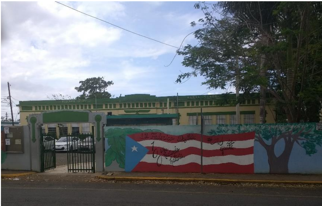
Figure 2. Detail of the concrete fence, showing the pedestrian entrance gate and front sidewalk.
