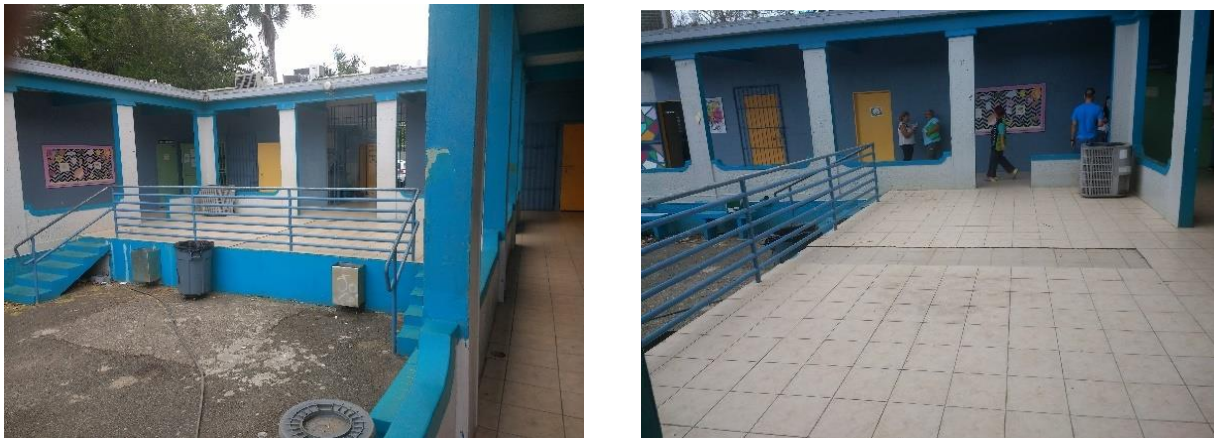
Figure 8. Views of the gallery and the elevated platform.
