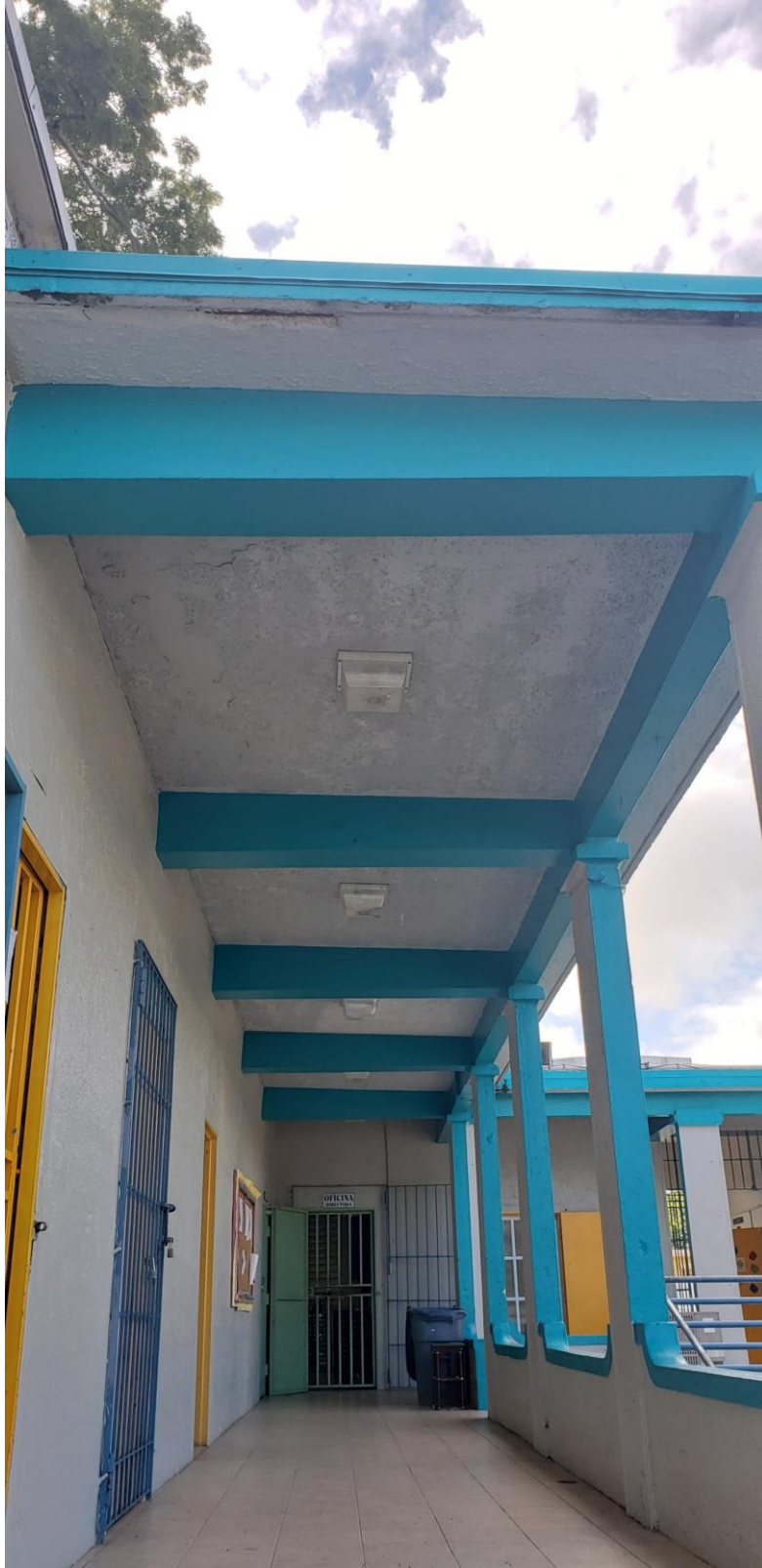
PR_Arecibo_Federico Degetau Consolidated Rural School_0005
