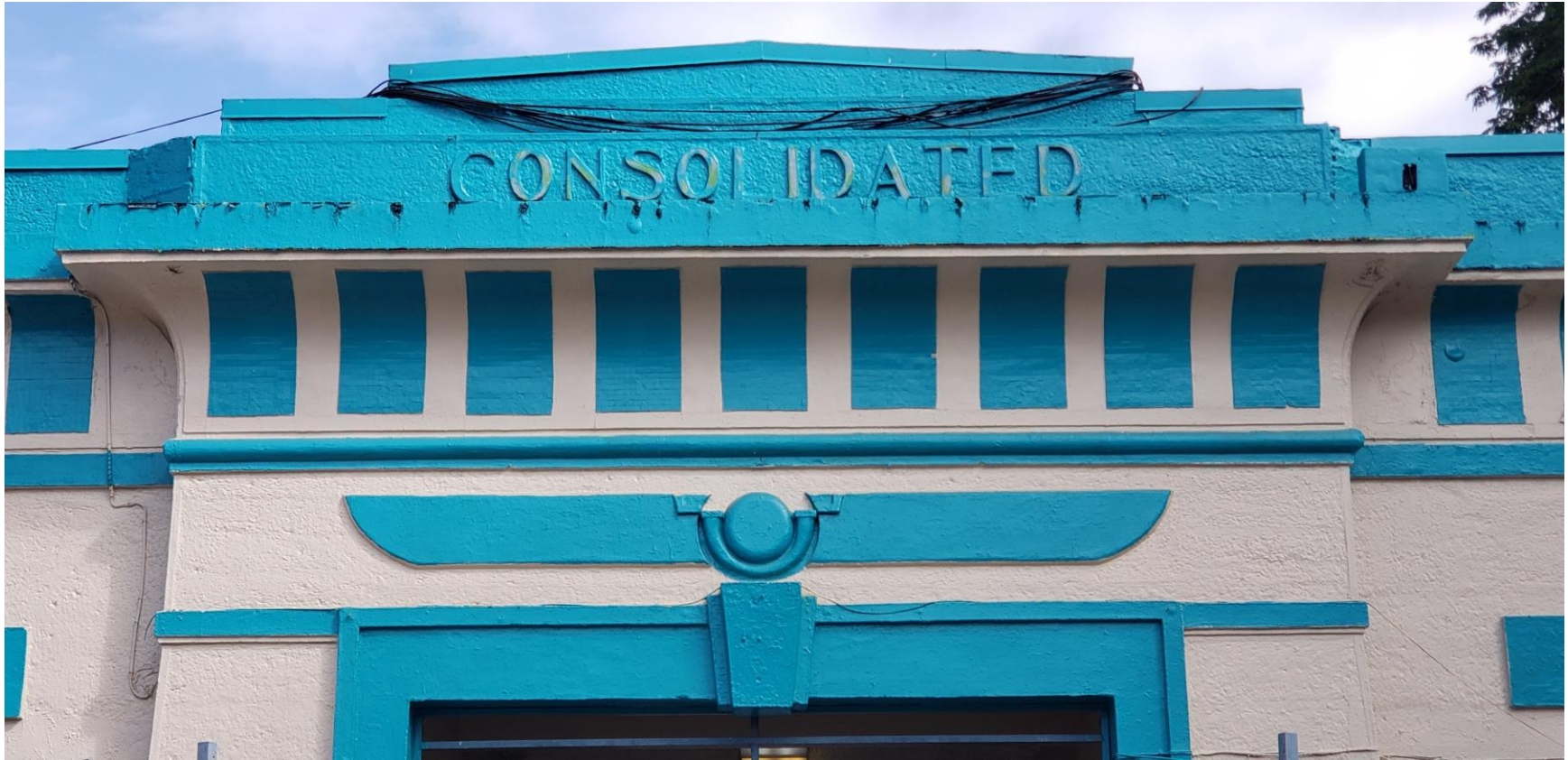
PR_Arecibo_Federico Degetau Consolidated Rural School_0003
