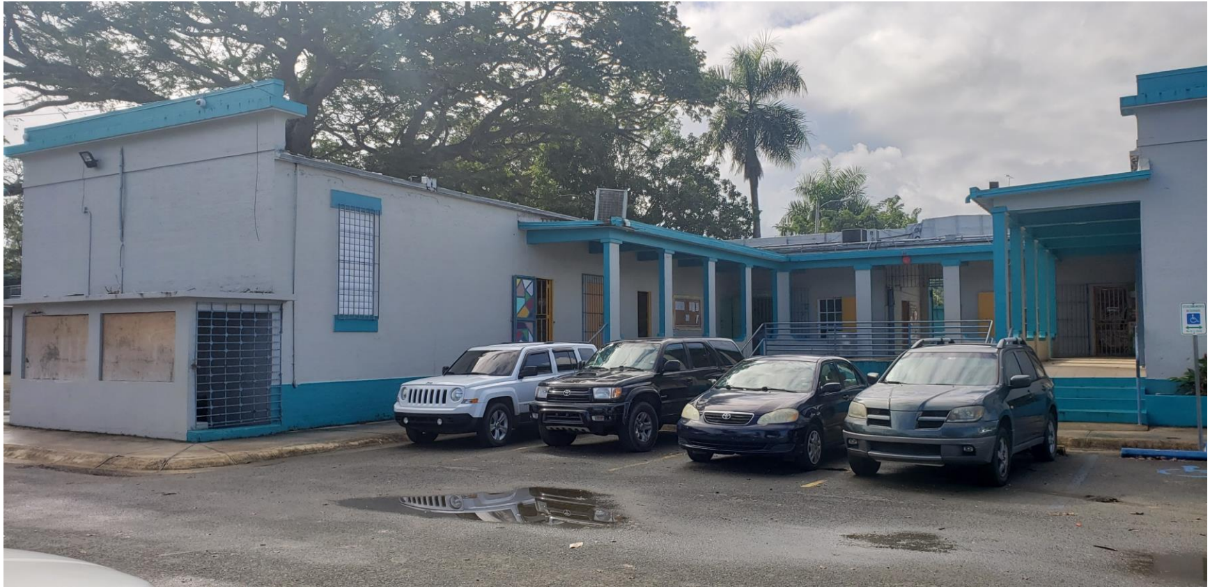
PR_Arecibo_Federico Degetau Consolidated Rural School_0002
