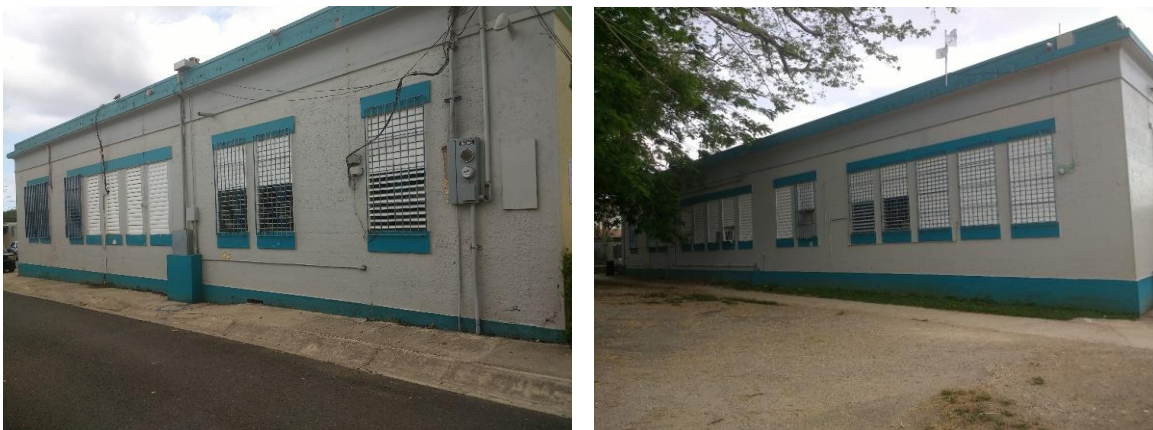
Figure 7. Partial views of the western façade (left) and eastern façade (right).
