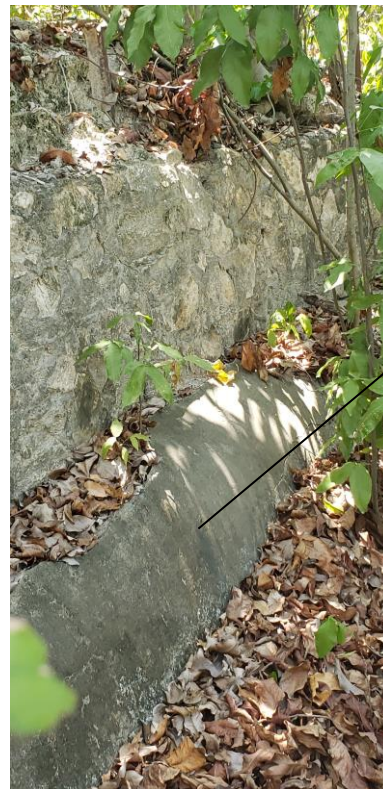
Figure 7. Photos show sections of the conduit channel showing construction material: brick, stone and hydraulic concrete for the outer shell, with the interior vault made of brick with a hydraulic cement grout. The conduit channel in the pictures below still retains parts of its outer fabric horseshoe vaulted component. (Juan Llanes, 2019)
