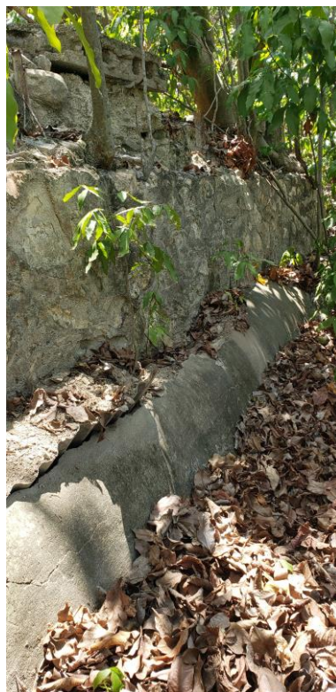
Figure 7. Photos show sections of the conduit channel showing construction material: brick, stone and hydraulic concrete for the outer shell, with the interior vault made of brick with a hydraulic cement grout. The conduit channel in the pictures below still retains parts of its outer fabric horseshoe vaulted component. (Juan Llanes, 2019)
