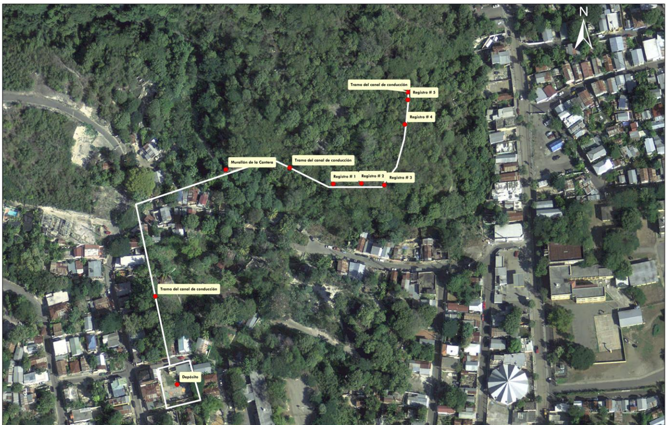
Figure 6. Alignment of the conduit channel found, along with the five manholes: Registro #1 (UTM, E 752676 / N 1994170); Registro #2 (UTM, E 752694 / N 1994168); Registro #3 (UTM, E 752711 / N 1994166); Registro #4 (UTM, E 752727 / N 1994218); Registro #5 (UTM, E 752728 / N 1994233). (Map prepared by Eduardo Cancio, PRSHPO, 2019).
