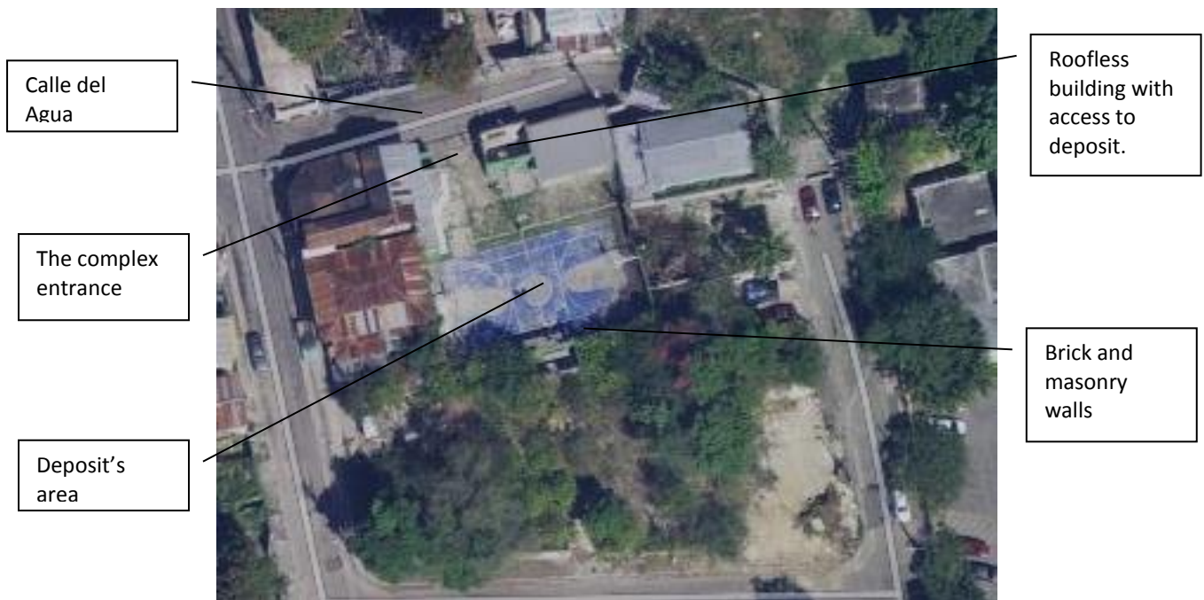
Figure 5. Aerial view of the deposit's area: the basketball court, the brick and masonry roofless building with sealed-off access to the deposit and the brick and masonry wall that surrounds most of the area.
