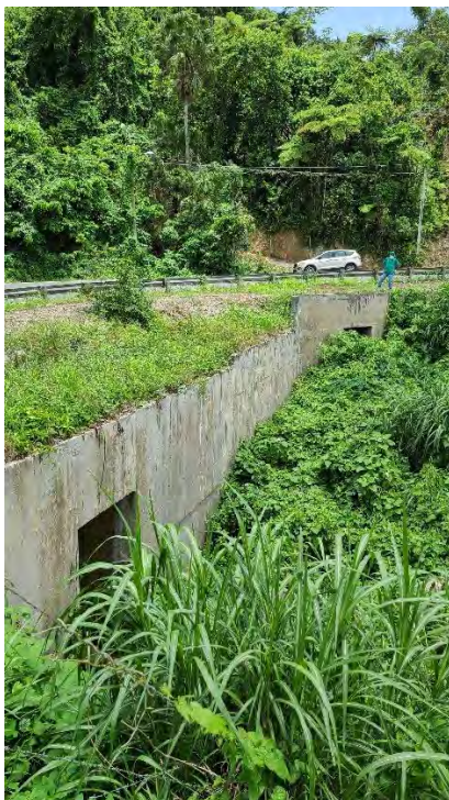
Figure 51. Above, photo of a pair of culverts included in the Report of the Military Governor of Porto Rico , published in 1900. Below, a photo of the very same resources. The concrete façade responds to a modern expansion of the road, hiding and extending the historic culvert. However, if approach from the hillside on the background, both 1900's façades come to perfect view, allowing, even with the sediment, the entrance into the historic culverts. From the inside, the 1900 construction and the modern concrete expansion are easily identifiable and distinguishable. (Photo, Juan Llanes Santos)
