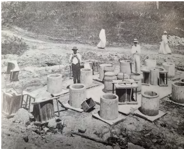
Figure 38. Above, a 1901 drawing of a concrete pipe culvert to be used somewhere in Carretera Num. 6 , between Utuado and Arecibo. 71 Below (left), shows a concrete pipes construction site. 72 Below (right) an example of the many extant cylindrical concrete pipe culverts, introduced in Carretera Num. 6 , during the early stage of the road construction after 1898 by the American engineers. The concrete cylinders were about one meter in length, with widths ranging from sixty to almost eighty centimeters. Mortar jointed, they extended the road's width, usually in a decline angle on which logically the pipe inlet was placed higher than the pipe outlet. In the culvert's 2020 photo, located at Km. 37, the collecting box, the headwall, the wing-walls, and the parapet are decorated with the extruded mortar joint technique with an added Grapevine design, similar to the design depicted in the 1901 drawing. (Photo, Juan Llanes Santos)
