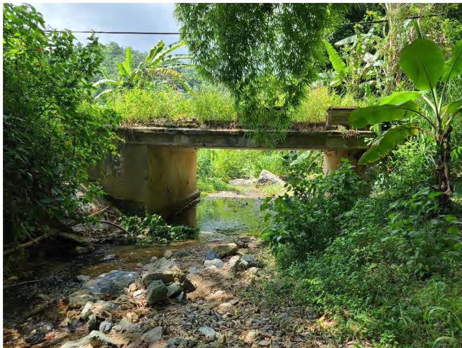
A 1920's concrete slab bridge, located at Km. 46.7, with its exposed aggregate as a trademark of the 1920's construction period. The structure type was a quick solution to cross water obstacles widely used by the Department of the Interior. (Photo, Juan Llanes Santos)
