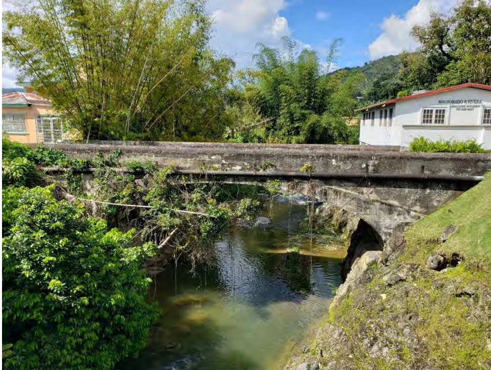
Just as Carretera Núm. 6 leaves Adjuntas' urban core on its way to Utuado, this 16.8 meters, elliptic arch reinforced concrete bridge was built in 1901 above Rio Cidra. Used as a pedestrian bridge today, is located at km. 35.8. (Photo, Juan Llanes Santos)
