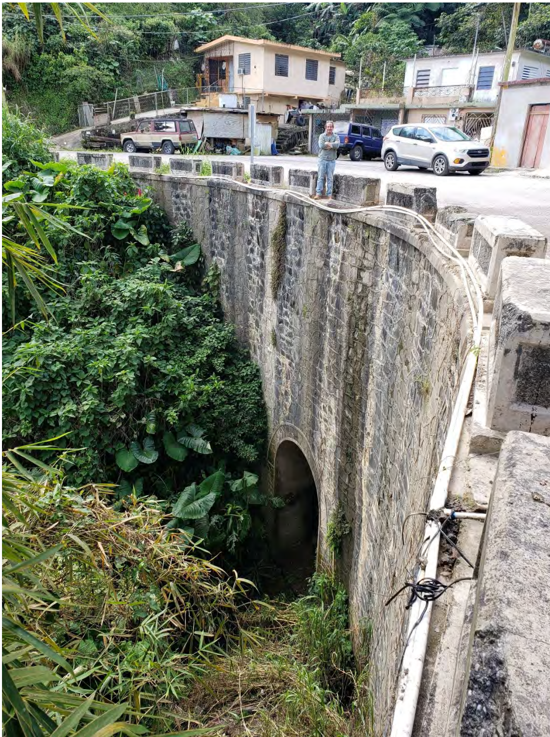
Located at Km. 27.6, in the Ponce-Adjuntas Section (Adjuntas's jurisdiction), this impressive and inaccessible culvert shows an intense purpose of making an aesthetical statement out of a practical structure. The extruded mortar joint effect was profusely used in the culvert's headwall and in the entire retaining wall. (Photo, Juan Llanes Santos)
