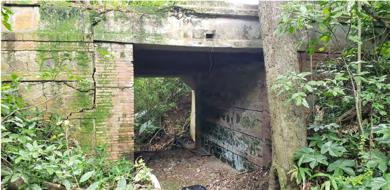
Pontón with its 19 th century brick, stone, and masonry abutments, and its original longitudinal iron beams. The parapets are an early 20 th century addition. The structure is located at Km. 14.0, in the Ponce-Adjuntas Section. (Photo, Juan Llanes Santos)
