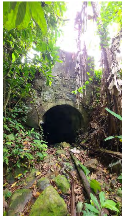
Figure 51. Above, photo of a pair of culverts included in the Report of the Military Governor of Porto Rico , published in 1900. Below, a photo of the very same resources. The concrete façade responds to a modern expansion of the road, hiding and extending the historic culvert. However, if approach from the hillside on the background, both 1900's façades come to perfect view, allowing, even with the sediment, the entrance into the historic culverts. From the inside, the 1900 construction and the modern concrete expansion are easily identifiable and distinguishable. (Photo, Juan Llanes Santos)
