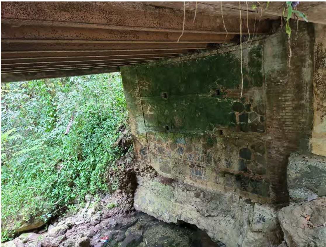
Partial view of a 19 th century bridge with its stone, brick and masonry abutments, built upon the natural rock foundation, with its original longitudinal iron beams, supporting the modern asphalted roadway. The structure is located at Km. 17.7 in the Ponce-Adjuntas Section. (Photo, Juan Llanes Santos)
