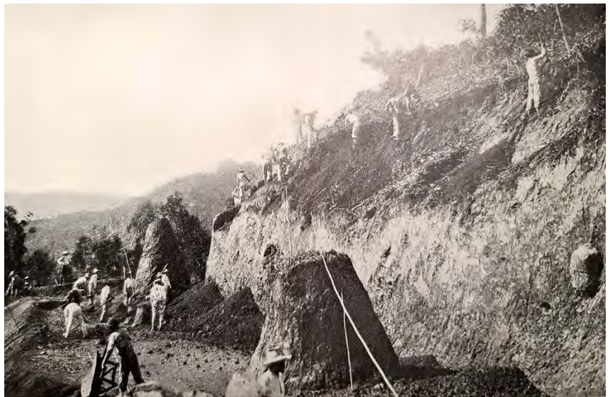
Figure 39. Above, workers grading a section between Utuado and Adjuntas. Below, all hands on deck filling, grading, and shaping the box for the eventual macadam, also in Carretera Núm. 6 . 73
