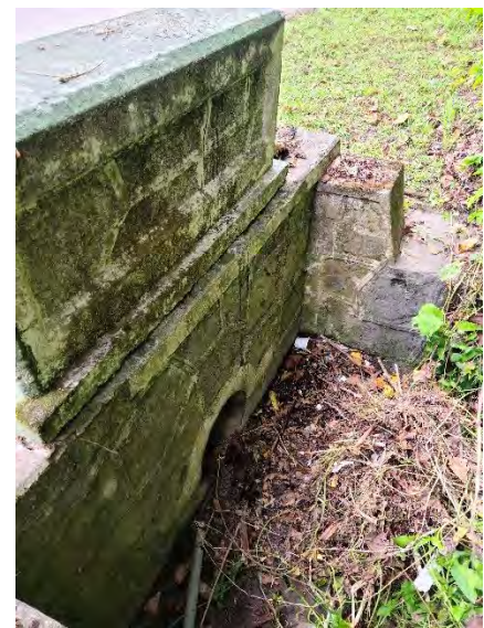
Figure 38. Above, a 1901 drawing of a concrete pipe culvert to be used somewhere in Carretera Num. 6 , between Utuado and Arecibo. 71 Below (left), shows a concrete pipes construction site. 72 Below (right) an example of the many extant cylindrical concrete pipe culverts, introduced in Carretera Num. 6 , during the early stage of the road construction after 1898 by the American engineers. The concrete cylinders were about one meter in length, with widths ranging from sixty to almost eighty centimeters. Mortar jointed, they extended the road's width, usually in a decline angle on which logically the pipe inlet was placed higher than the pipe outlet. In the culvert's 2020 photo, located at Km. 37, the collecting box, the headwall, the wing-walls, and the parapet are decorated with the extruded mortar joint technique with an added Grapevine design, similar to the design depicted in the 1901 drawing. (Photo, Juan Llanes Santos)
