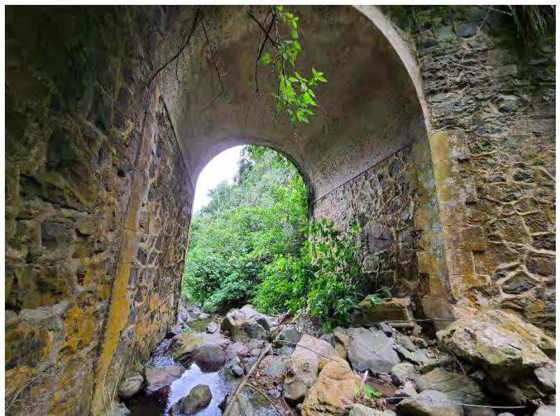
Figure 34. Above, Gandía Cordova's 1900 drawing for the Defendini's culvert. Located at Km. 28.4, the culvert was built at the center of the dense vegetation of the horseshoe bend of Carretera Núm. 6 . Hardly accessible and unseen from the roadway, the pontón received a beautiful treatment using the Cyclopean masonry arrangement in the culvert's headwall, wing-walls, and interior walls, topped with a concrete barrel vault with exposed aggregated. (Photos, Juan Llanes Santos)
