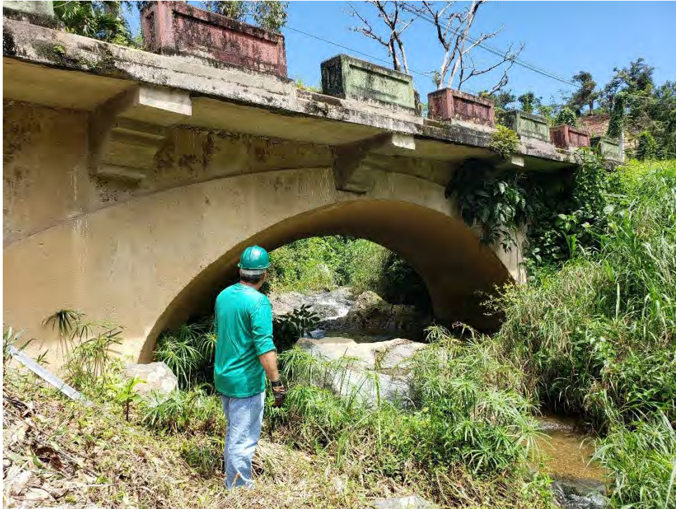
Resembling the previous pontón in construction material and style with its concrete elliptic arch, the one located at km. 32.2, shows the original width of Carretera Núm. 6 , with its 1930's extension.
