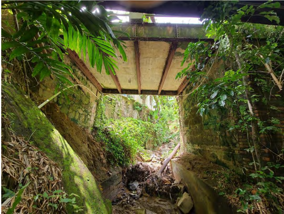
Figure 24. The six meters structure above contains the components specified by Larrinaga in the 1880s for a pontón of this size: brick and masonry abutments, the needed transversal rolled iron beams (5 in this case) and two embedded longitudinal iron beams. (Photo, Juan Llanes Santos)
