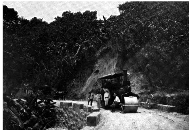
Figure 36. Images above were all taken during the actual construction of the Arecibo – Ponce Road, Carretera Núm. 6 . (Source of the first three photos, left to right: Report of the Military Governor of Porto Rico on Civil Affairs, 1900). At the moment of the photo, the steam roller shown above has been used in Tallones, Adjuntas, the last section of Carretera Núm. 6 , finished by 1904. (Source: Report of the Commissioner of the Interior, 1901).
