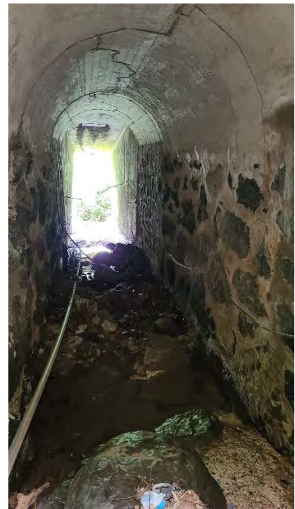
Figure 51. Above, photo of a pair of culverts included in the Report of the Military Governor of Porto Rico , published in 1900. Below, a photo of the very same resources. The concrete façade responds to a modern expansion of the road, hiding and extending the historic culvert. However, if approach from the hillside on the background, both 1900's façades come to perfect view, allowing, even with the sediment, the entrance into the historic culverts. From the inside, the 1900 construction and the modern concrete expansion are easily identifiable and distinguishable. (Photo, Juan Llanes Santos)
