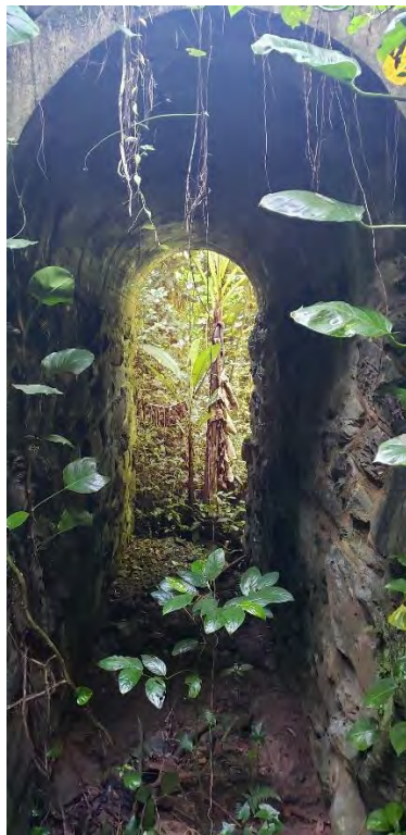
Figure 37. Two early 20 th century culverts with rough facing stones in the headwalls and wing-walls, with concrete vaulted ceilings. Both culverts are located within the Ponce - Adjuntas section built under the new American engineers. (Photos, Juan Llanes Santos)
