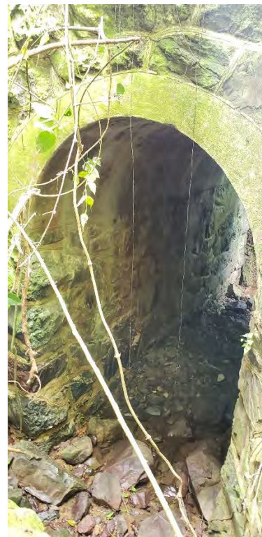
Figure 37. Two early 20 th century culverts with rough facing stones in the headwalls and wing-walls, with concrete vaulted ceilings. Both culverts are located within the Ponce - Adjuntas section built under the new American engineers. (Photos, Juan Llanes Santos)
