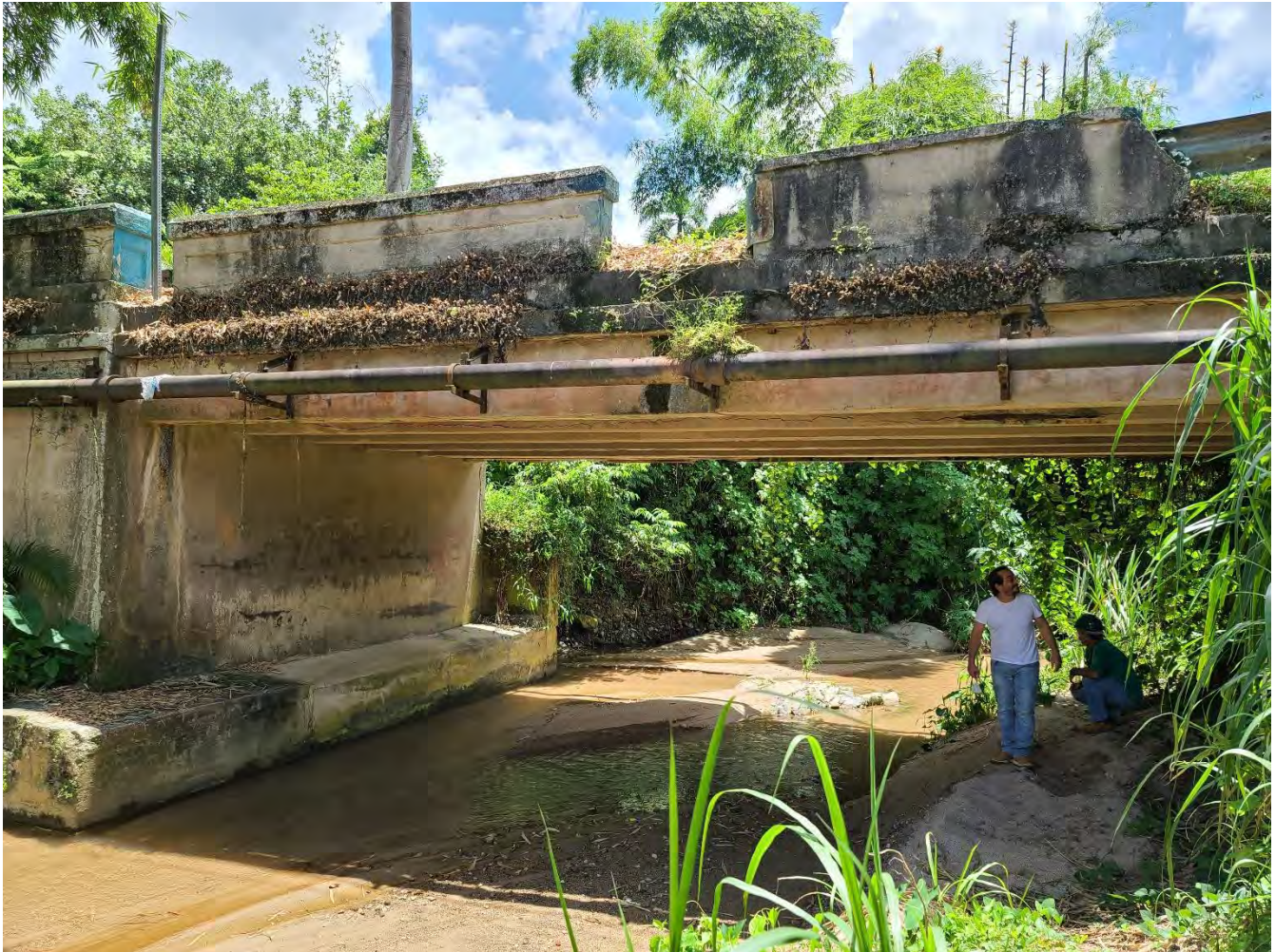
The reinforced concrete slab, with longitudinal concrete coated iron beams, spans ten meters over Quebrada Arenas. The bridge, located at Km. 53.5, was built in 1924. Just like the previous bridge at Km. 46.7, this model had the advantage of been a quick construction to be overcome the natural obstacle. The Department of the Interior at this time (1920's) was under direct control of a new cadre of Puerto Rican engineers. (Photo, Juan Llanes Santos)
