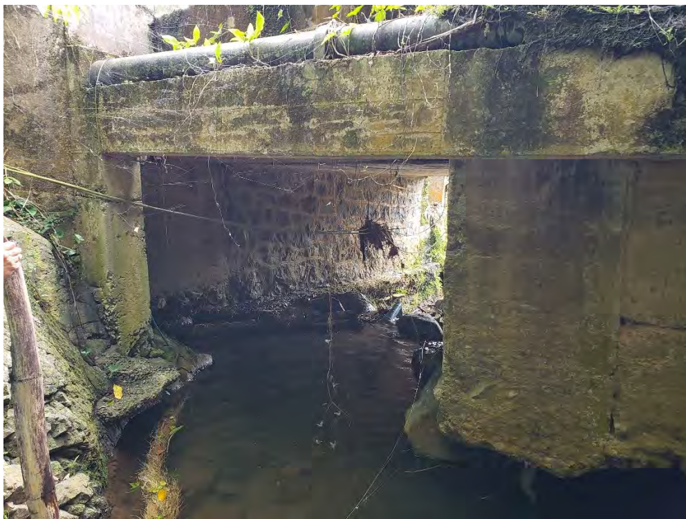
Located at Km. 34.7, this early 20 th century pontón , uses the extruded concrete mortar joint technique resembling the Cyclopean masonry method used by the Spanish engineers. It is possible that this similarity could be attributed to the contractors and labor used, more than to the American engineers in charge at the time. (Photo, Juan Llanes Santos)
