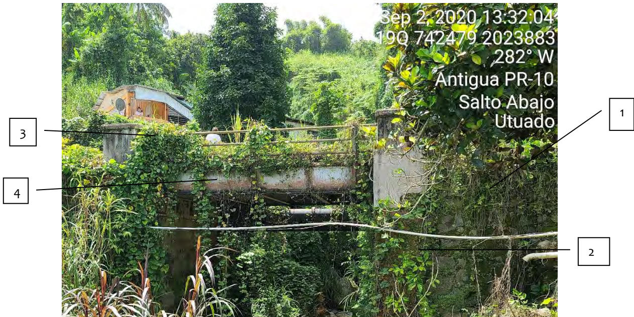
Figure. 21 Above, partial view of an 1891 drawing done by engineer Pedro F. Fernandez to be used as model for a ten-meter span bridge with a tramo metálico . 33 Below, an 8.5 meters span bridge in the Utuado-Arecibo section, on which the major structural components from the 1880's still present: 1) masonry abutments; 2) brick columns; 3) metal railings; 4) full body ( alma llena ) longitudinal iron beams. Although not depicted in the 1891 drawing, been a ten meters span bridge required supporting transversal (not longitudinal) iron beams. The photo below shows the transversal beams for this particular structure. (Photo, Juan Llanes Santos)
