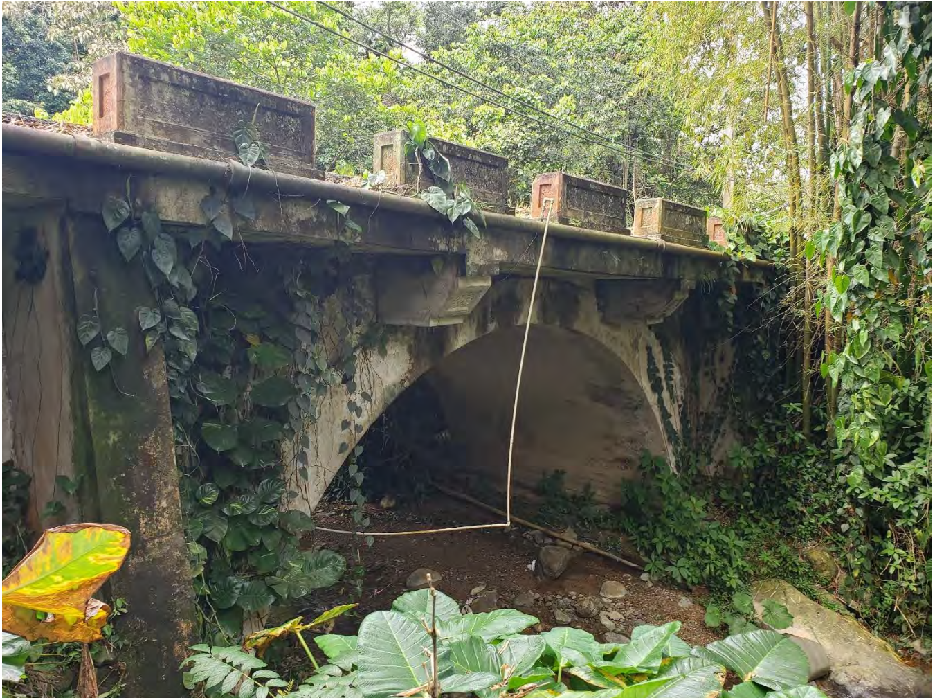
Few kilometers short of reaching Adjuntas' urban center, this pontón located at km. 32, shows reinforced concrete used as the new construction material in substitution of stones, brick and masonry. However, the molding accentuating the elliptic arch resemble the traditional Spanish's methods of construction. (Photo, Juan Llanes)
