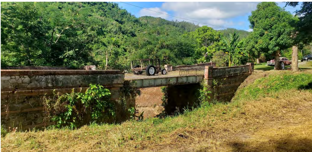
Puente Juana Matos , located at Km. 14.9, in the Ponce-Adjuntas Section. Finished in the early 1890s, the Juana Matos Bridge combined brick, stone and masonry for the abutments, iron beams and metal plates for roadway support, masonry parapets with added bronze metal railings. The bridge sits today in a private property, as PR-123 was diverted and widened just fifty meters northeast of the bridge. (Photo, Juan Llanes Santos)
