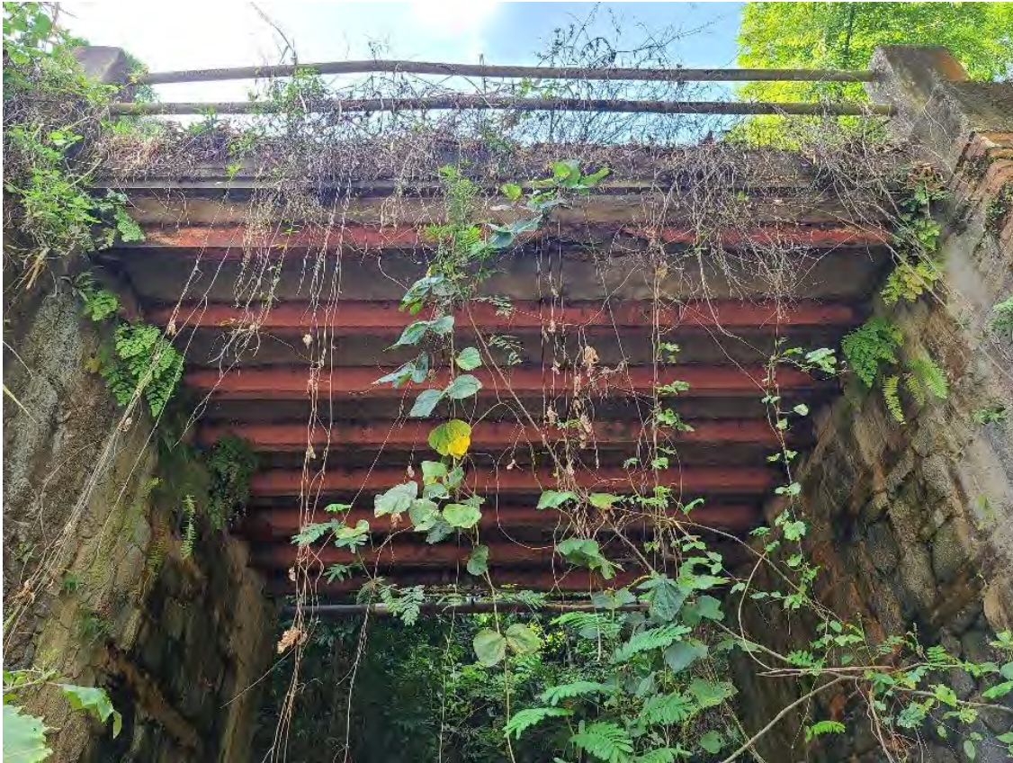
Figure 23. This five-meter span pontón , located at km. 57 in the Utuado-Arecibo section, retains most of the construction specifications as instructed by Tulio Larrinaga in the 1880s: its brick and masonry abutments, the eight longitudinal beams of rolled iron (painted red) embedded in the masonry interior walls supporting today concrete pavement and its two longitudinal iron beams providing support to the safety railings, parapets, and railing pedestals. (Photo, Juan Llanes Santos)
