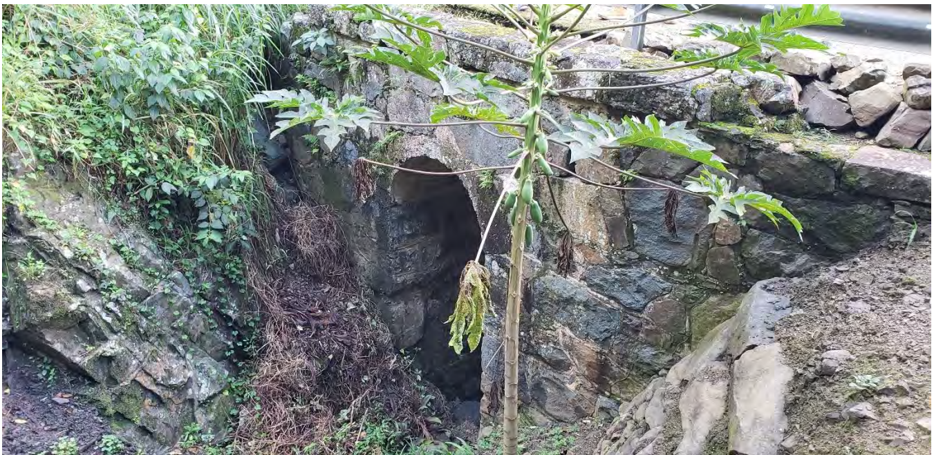
Km. 26.0. The culvert shows the 1940's expansion (above) on its eastern façade, while retaining its early 20 th century (1899-1904) construction technique on its western entrance.
