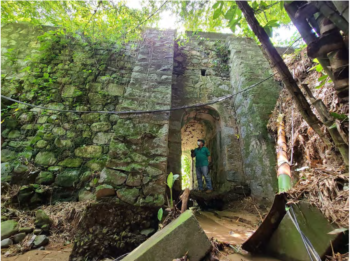
A fabulous culvert, located at Km. 54.7, in the Adjuntas-Utuado Section (municipality of Utuado). The structural design includes un-coursed rubble for the retaining walls, Cyclopean masonry arrangement in the culvert's headwall and interior wall, with a concrete barrel vault. The structure is supported by two coursed wall buttresses. (Photo, Juan Llanes Santos)
