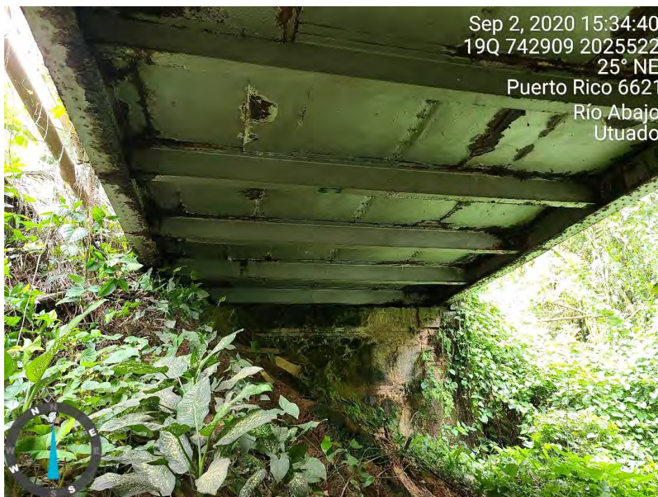
Figure 25. This six-meter long, six meters wide pontón , located at Km. 59.6, in the Utuado-Arecibo section, retains practically all the structural components mentioned by Larrinaga for a structure of its size: brick and masonry abutments, transversal iron beams, two main longitudinal iron beams, and even, the undulated metal planks. (Photo, Juan Llanes Santos)
