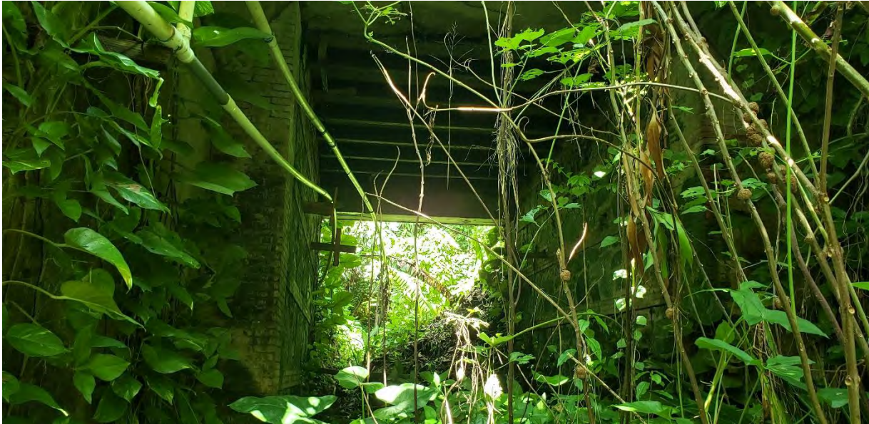
A pontón , in the Ponce-Adjuntas Section, at Km. 15.5, with its 19 th century stone, brick and masonry abutments, and its 19 th century longitudinal iron beams supporting the modern concrete/asphalted roadway. (Photo, Juan Llanes Santos)
