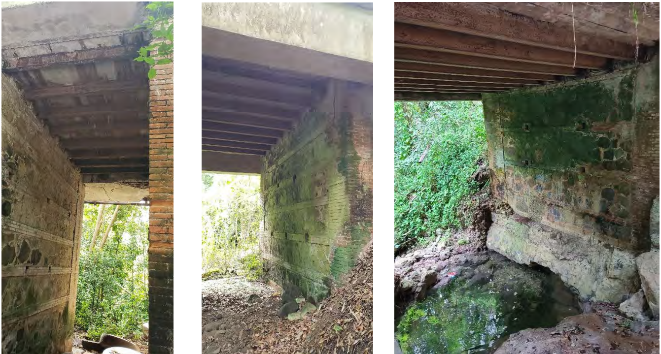
Figure 18. (Left to right) A two-meter culvert located at km. 13.6 and two five-meter pontones , located at km. 14.3 and 17.7 respectively, show some of the components describe by Larrinaga, according to their size.
