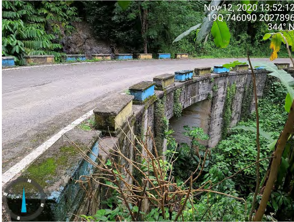
A late 1930's reinforced concrete bridge ( pontón ) at km. 67.4
