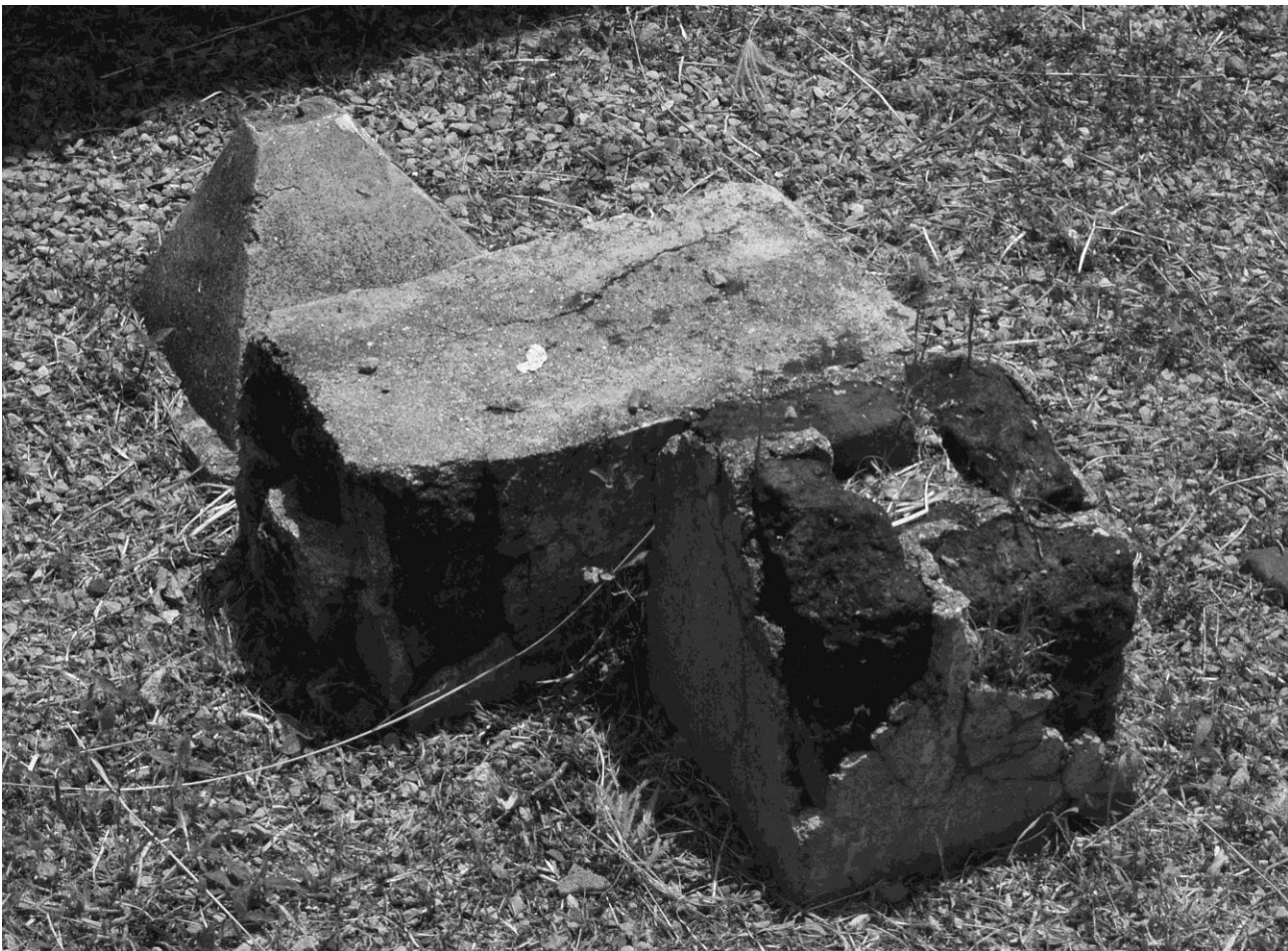
Fig. 7. The three masonry blocks, northwest corner.
