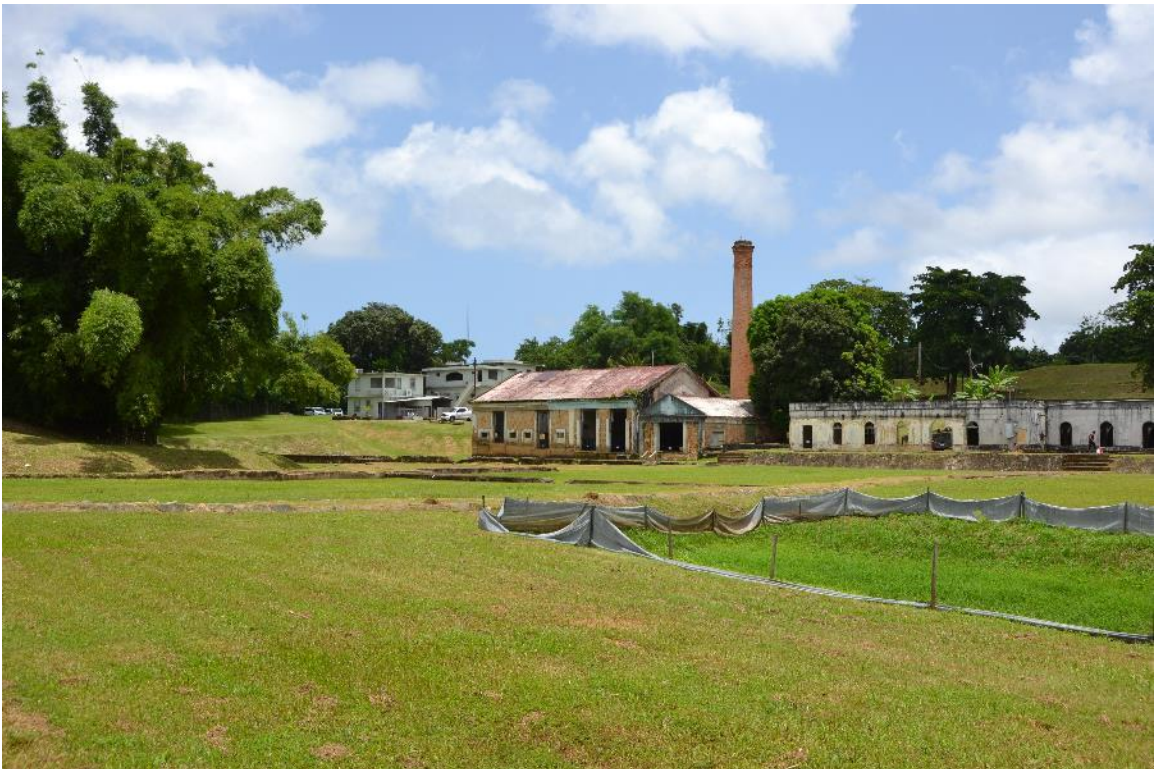
Photo #2: Settling basins, Director's Residence, Garage, Maid's House, Pumping House, and Chemical and Mechanical Filters' House
