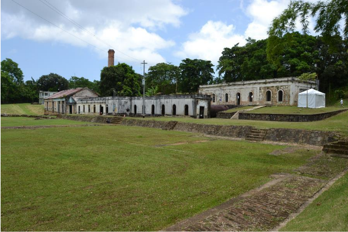
Photo #1: Settling basins, Chemical and Mechanical Filters' House, and Engineers and Caretakers' Residence, camera facing northeast
