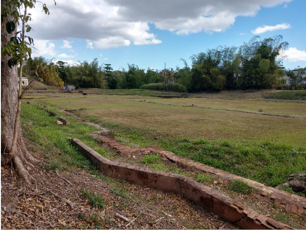
Photo #37: Settling Basins
