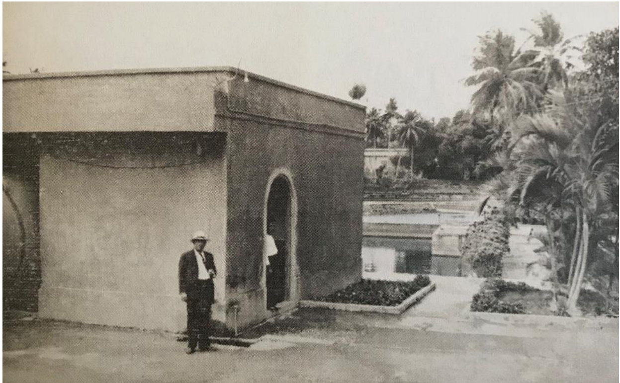
Figure #12: 1944 view of Chemical and Mechanical Filters' House
