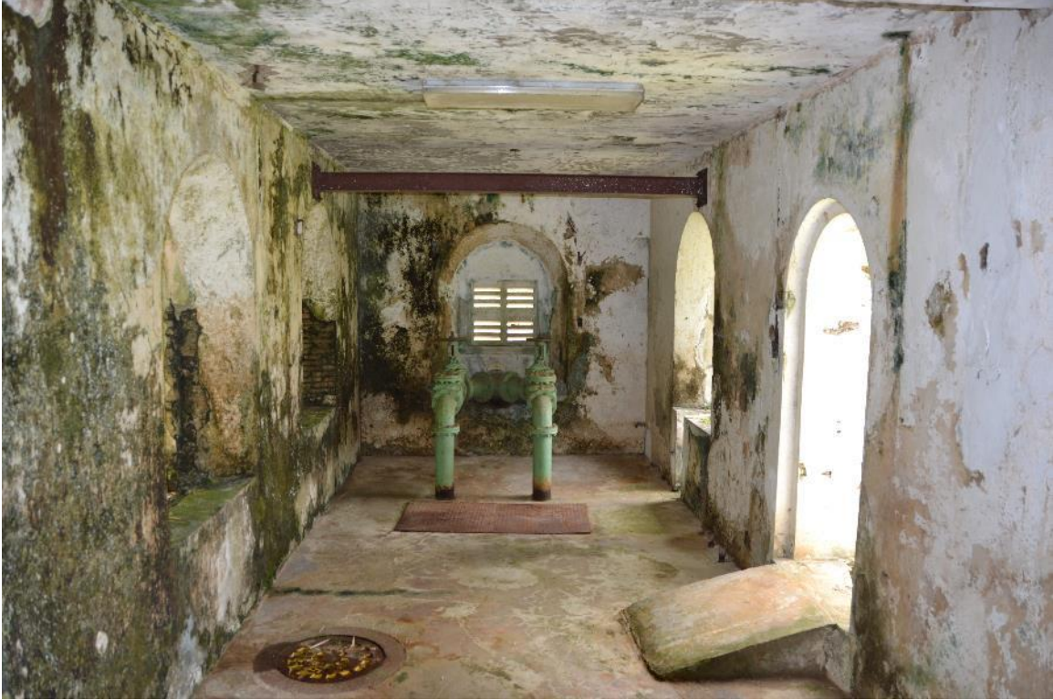
Photo #9: Mixing Chamber and Valve House, interior
