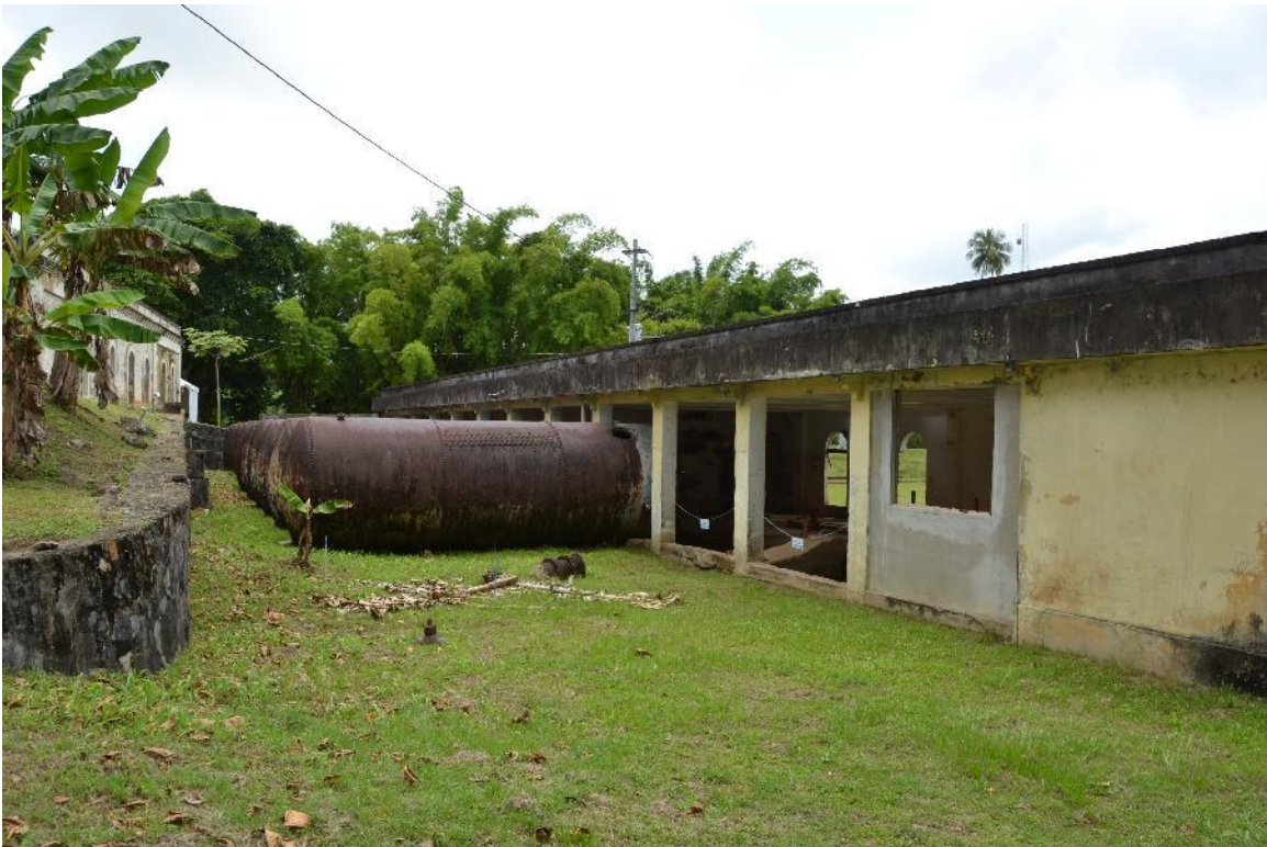
Photo #20: Chemical and Mechanical Filters' House
