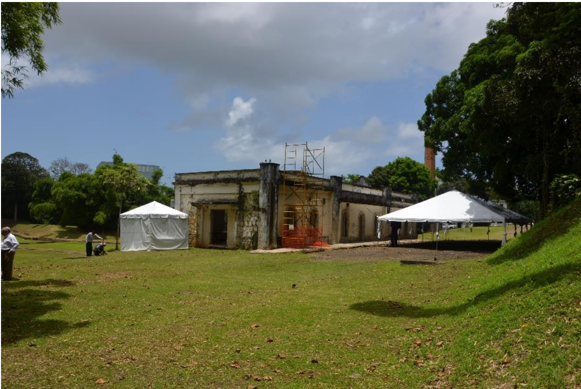
Photo 16: Engineers and Caretakers' Residence
