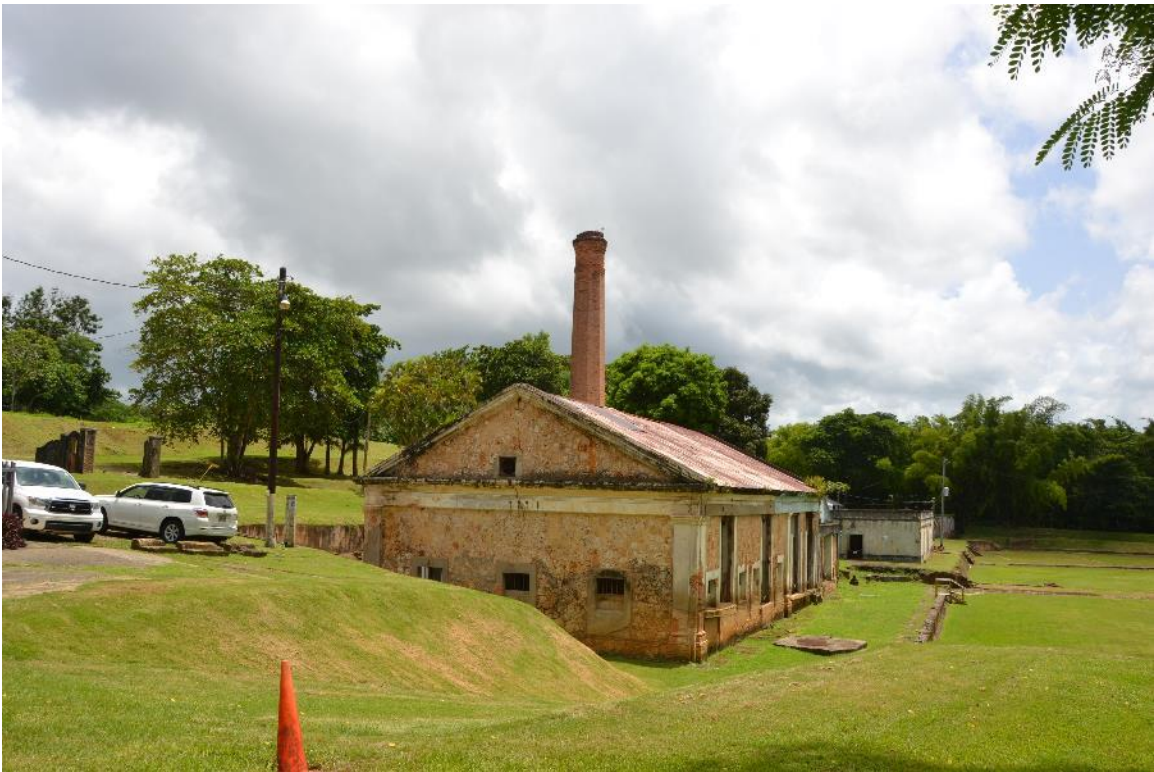
Photo #12: Pumping House
