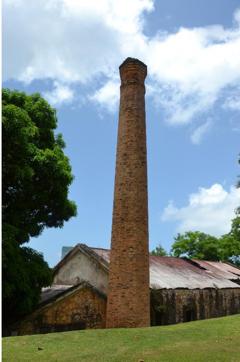
Photo #10: Pumping House
