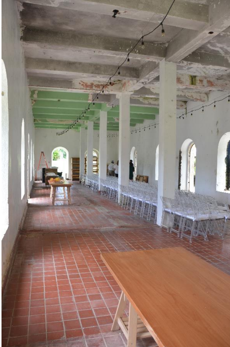
Photo #17: Engineers and Caretakers' Residence
