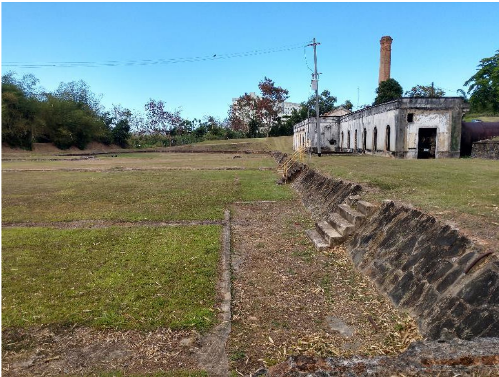
Photo #32: Settling Basins and Chemical and Mechanical Filters' House
