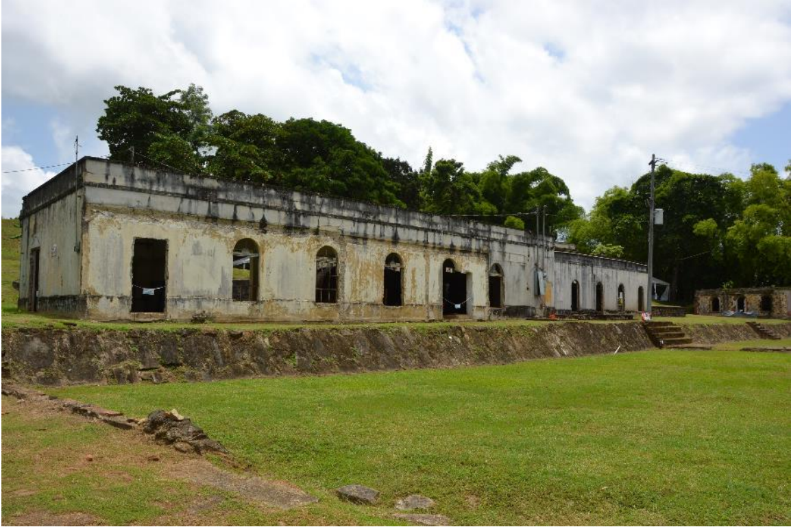
Photo #19: Chemical and Mechanical Filters' House
