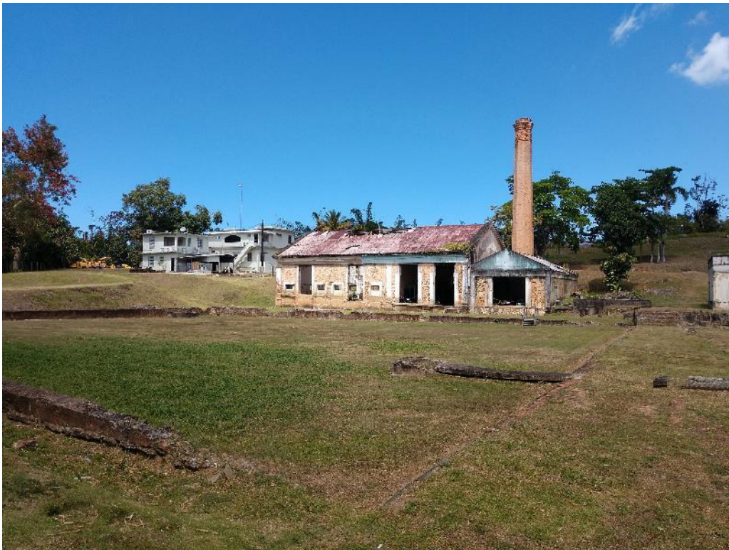
Photo #36: Settling Basins, Pumping House and Director's Residence
