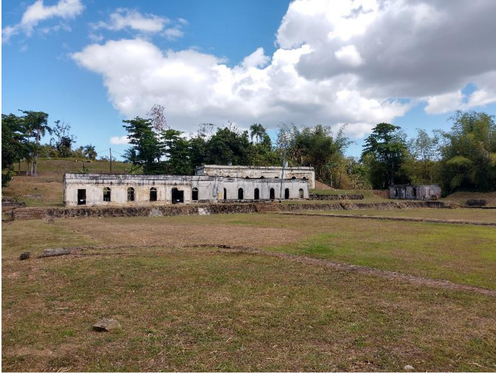
Photo #35: Settling Basins, Chemical and Mechanical Filters' House, and Engineer and Caretakers' Residence
