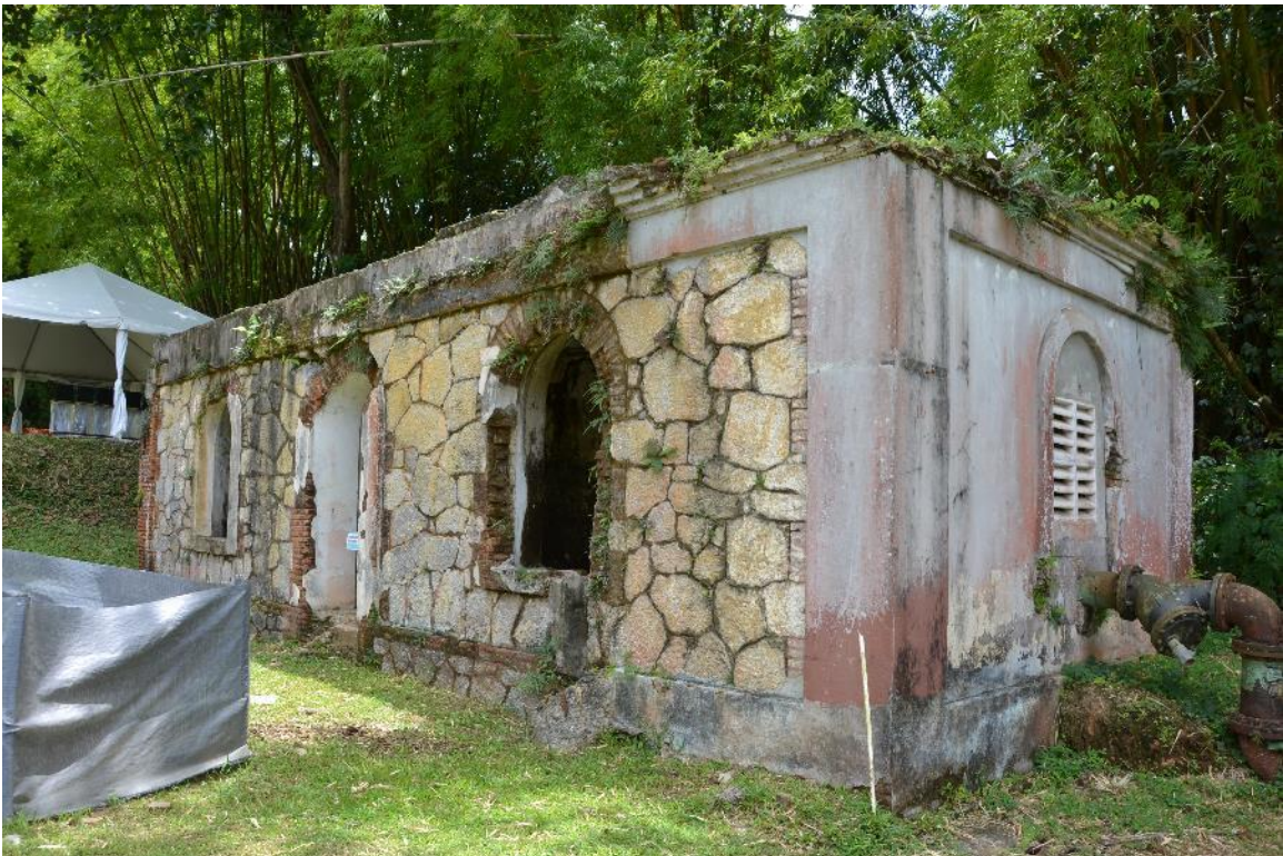
Photo #8: Mixing Chamber and Valve House
