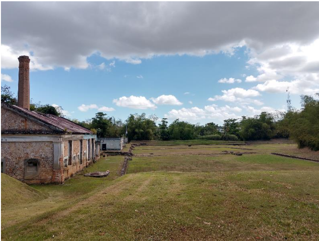
Photo #34: Settling Basins and Pumping House
