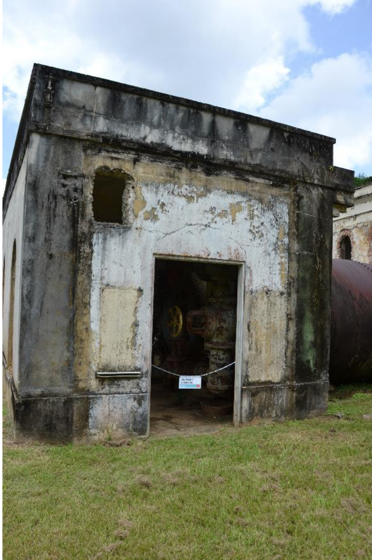
Photo #18: Chemical and Mechanical Filters' House
