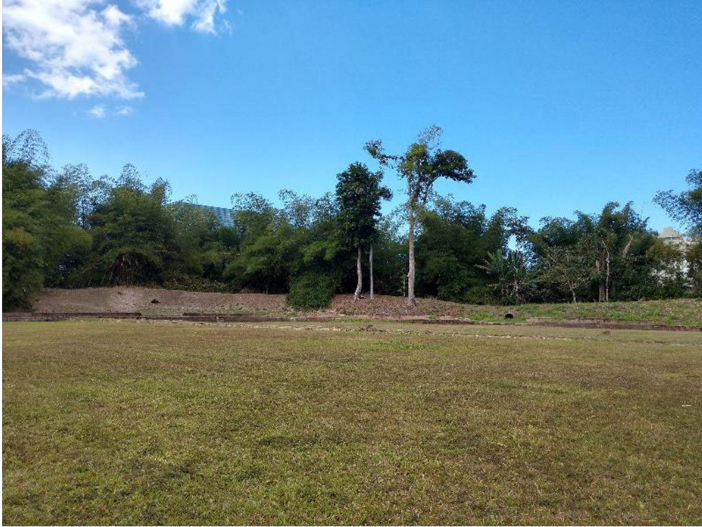
Photo #33: Settling Basins
