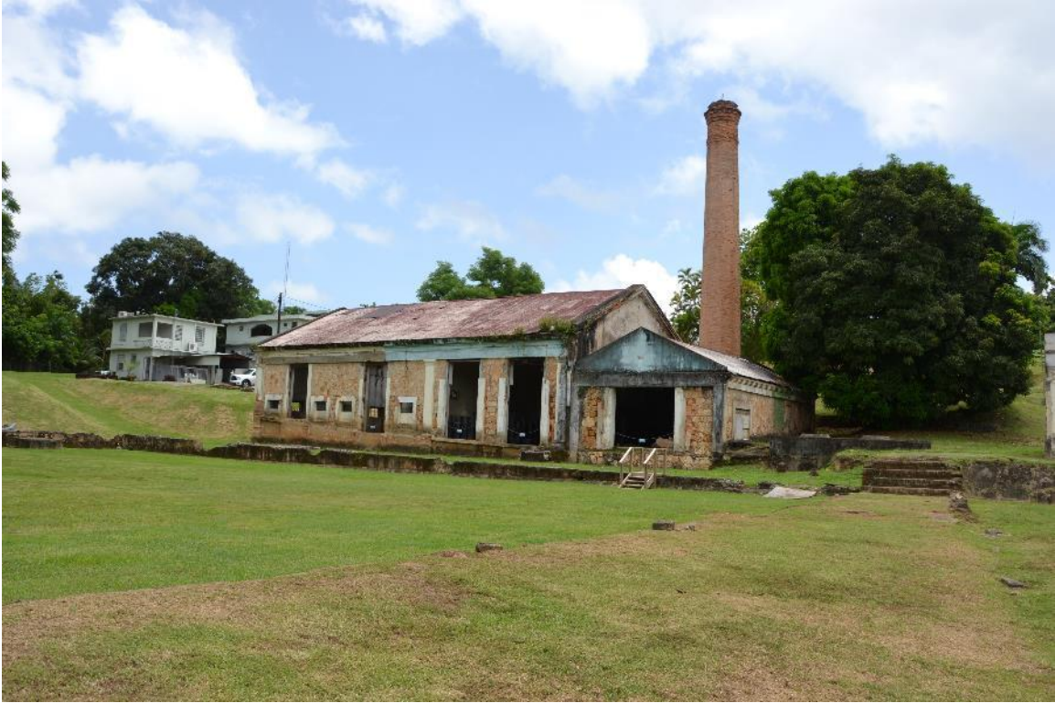
Photo #11: Pumping House
