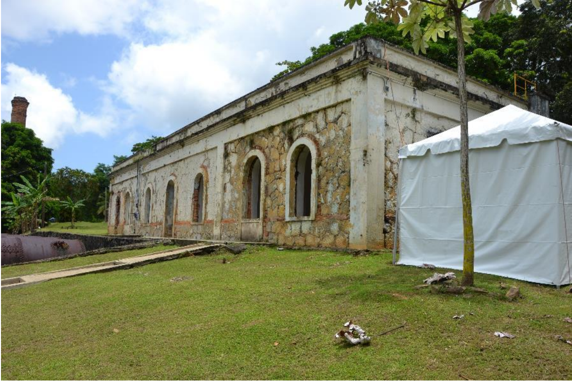
Photo #15: Engineers and Caretakers' Residence
