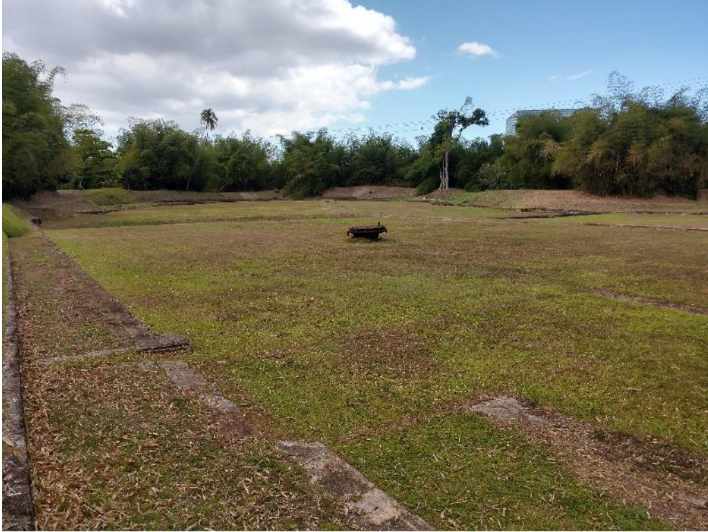
Photo #31: Settling Basins
