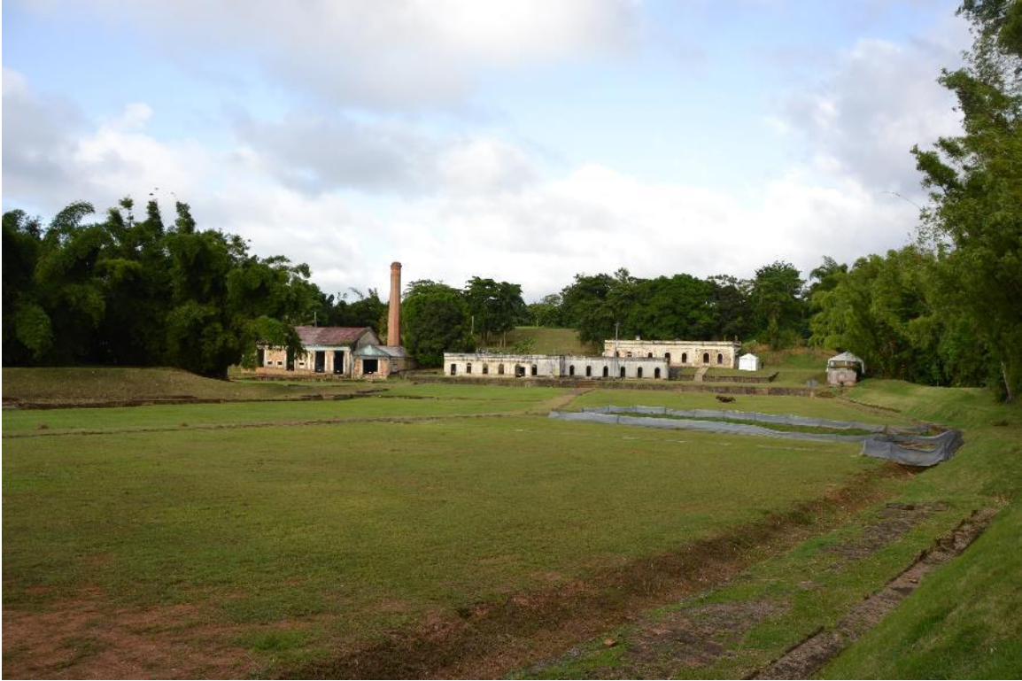
Photo #3: Settling basins, Pumping House, Chemical and Mechanical Filters' House, Mixing Chamber and Valve House
