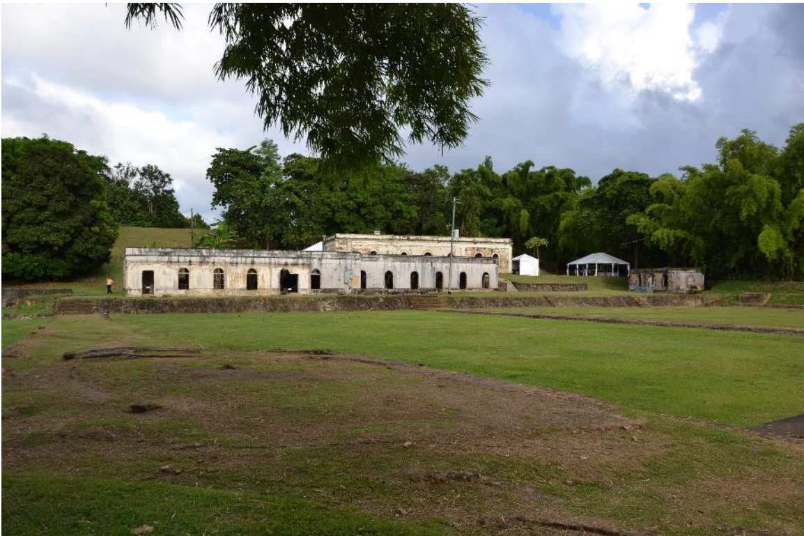
Photo #4: Settling basins, Chemical and Mechanical Filters' House, Engineers and Caretakers' Residence, Mixing Chamber and Valve House
