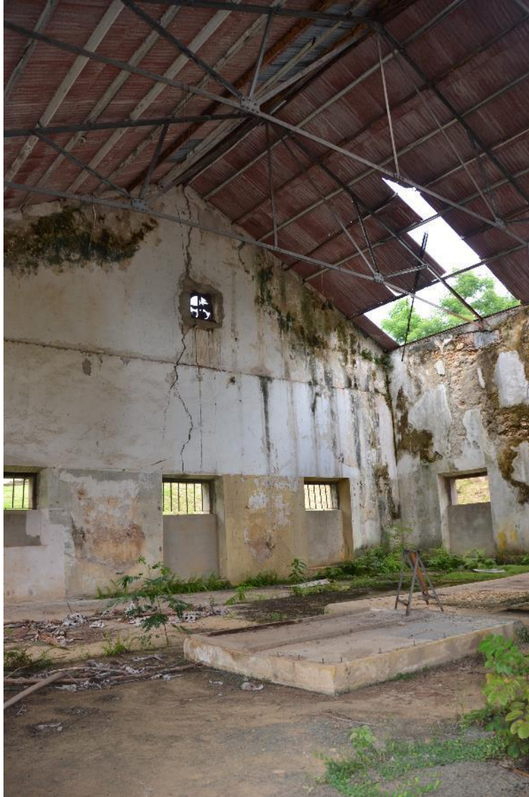
Photo #14: Pumping House
