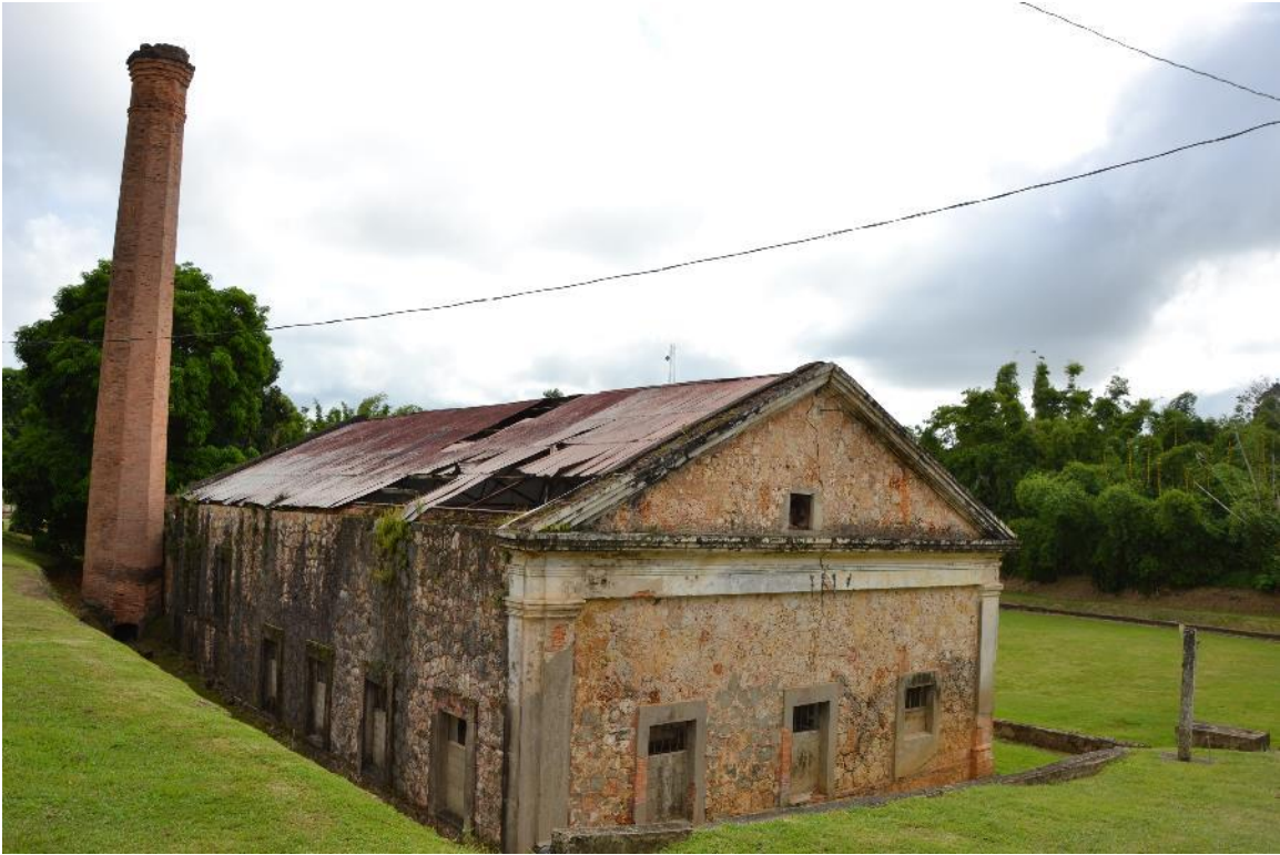
Photo #13: Pumping House
