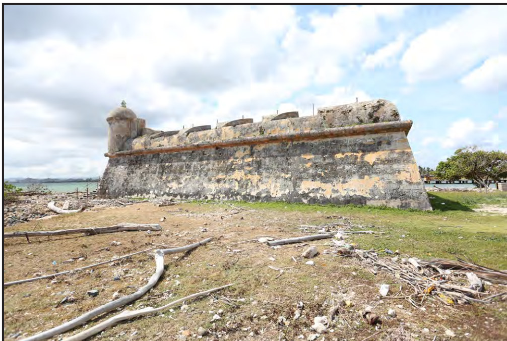
6 Fortín San Juan de la Cruz, Northeast Front, looking south.
