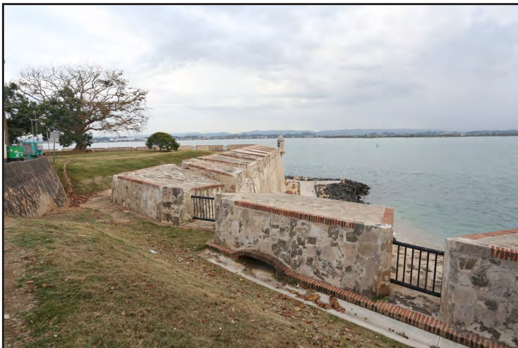
40 San Juan City Walls - West Wall, San Agustín Bastion, looking south.
