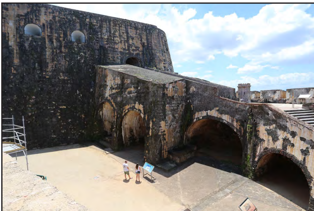
14 Castillo San Felipe del Morro, looking south. View of Kitchen Courtyard, Great Wall, and main ramp.
