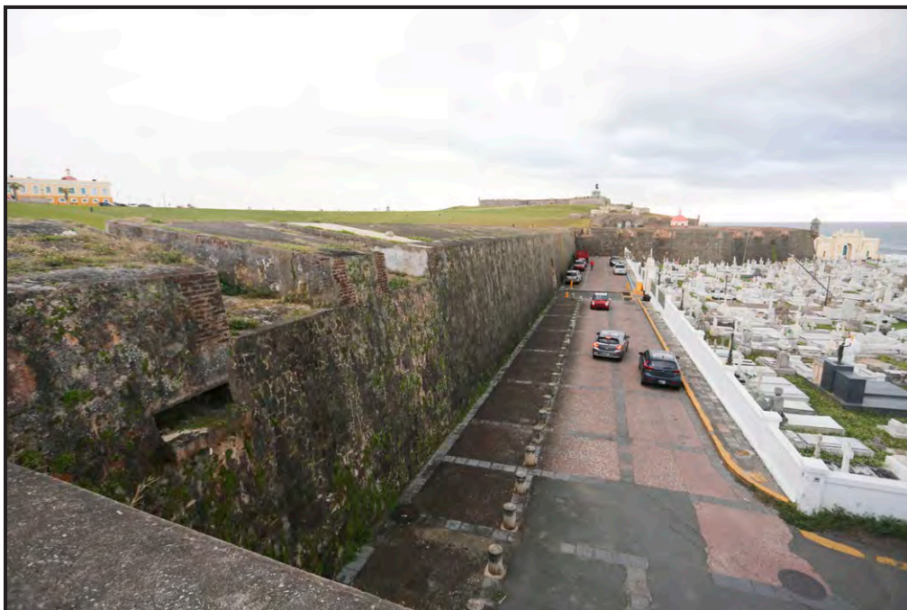
36 San Juan City Walls - North Wall, looking northwest. Resources shown: Santa Rosa Bastion, San Jose City Gate; El Morro Esplanade, Castillo San Felipe Del Morro. Santa María Magdalena de Pazzi Cemetery at right.
