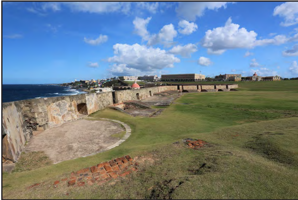
37 San Juan City Walls - North Wall, San Antonio Bastion, looking east.
