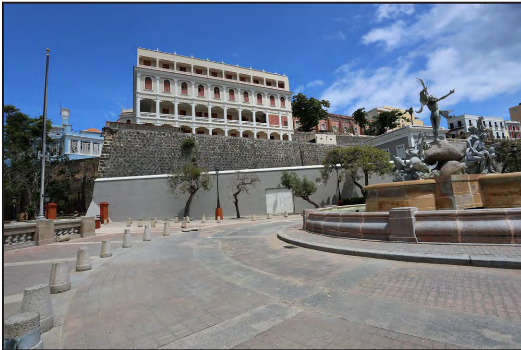
5 San Juan City Walls - South Wall, La Concepción Bastion, looking north.
