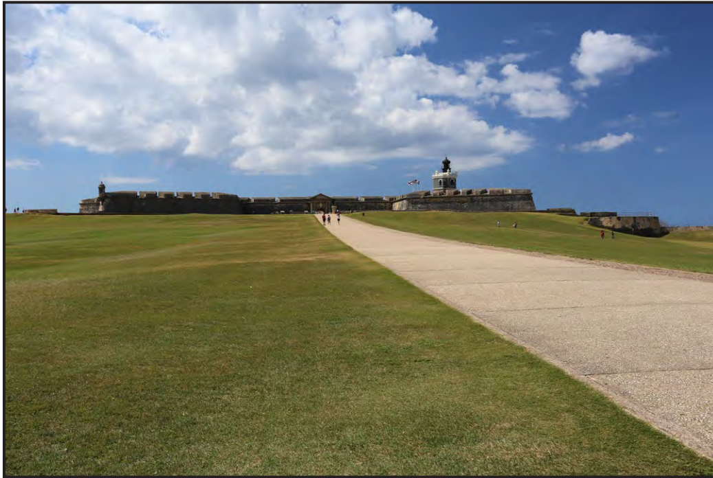
1 Castillo San Felipe del Morro, East Front, looking northwest. El Morro Road and El Morro Esplanade in foreground.
