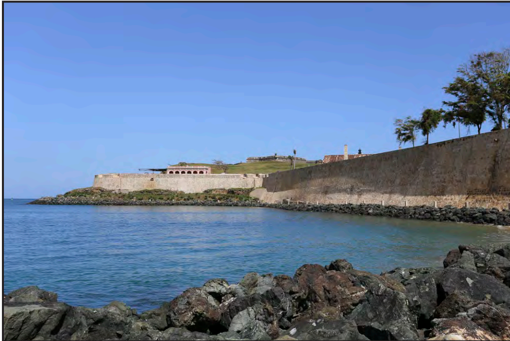
39 San Juan City Walls - West Wall, Santa Elena Bastion, looking north. Curtain wall between Santa Elena and San Agustín bastions at right.
