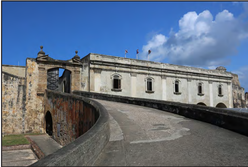
23 Castillo San Cristóbal, West Front, looking southeast. Resources shown: Main Gate at San Cristóbal; Officer's Quarters at San Cristóbal.
