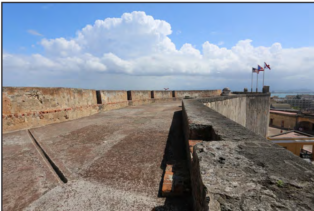
24 Castillo San Cristóbal, El Caballero terreplein, looking south.
