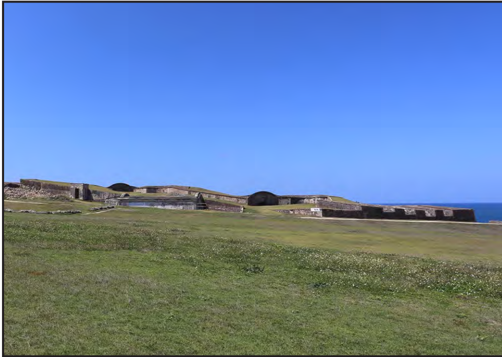
33 Castillo San Cristóbal Outworks, Santa Teresa Battery, looking northwest.
