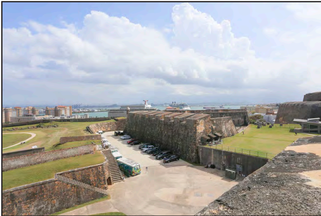
25 Castillo San Cristóbal Outworks, view south. Resources shown: portion of North Covered Way (at left); San Carlos Ravelin; San Cristóbal Moat; South Covered Way.
