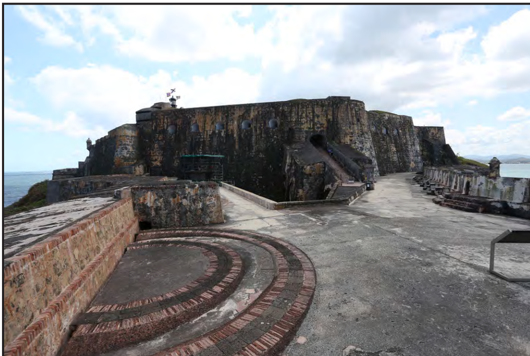
13 Castillo San Felipe del Morro, looking southeast. Resources shown: Santa Bárbara Bastion, Great Wall, and El Morro Fire Control Station A.
