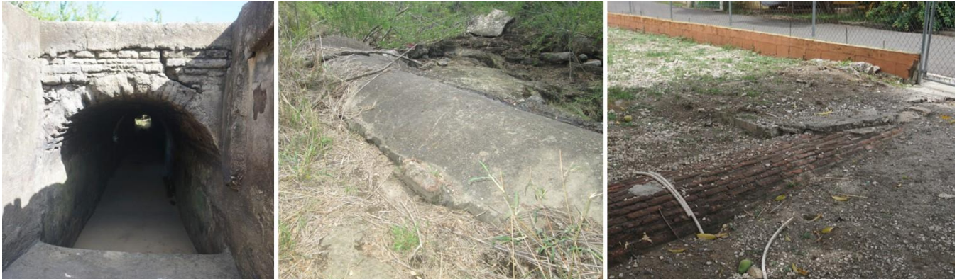
On the left, entrance to the Supply channel at the low-waters module, looking south from within the inlet. In the center, vaulted segment of the supply channel that runs along the surface in the area of the dam. Notice the concrete plastering over the vault. On the right, view of the channel as it emerges to the surface, in the backyard of a property of the El Ojo Community. Note that the vault does not have plastering.
