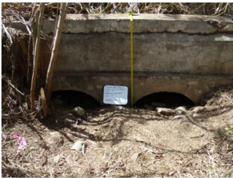
Left; Channel of the Hacienda Florida, raised on arches. Center; Channel of the Hacienda Florida, elevated on a base (note black arrows). Right; Channel of the Hacienda Florida, raised using a staggered base.
