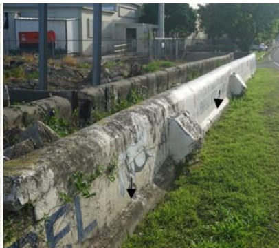
Left; Channel of the Hacienda Florida, raised on arches. Center; Channel of the Hacienda Florida, elevated on a base (note black arrows). Right; Channel of the Hacienda Florida, raised using a staggered base.
