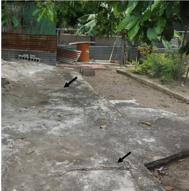
On the left, section of the supply channel covered with corrugated metal sheets and a slab of concrete. Arrows indicate the channel's route. To the right, supply channel in a backyard, filled with earth.
