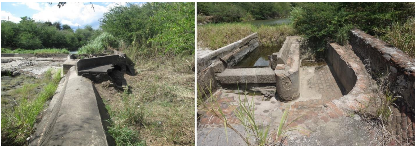
Left, general view of the area of the low waters and seasonal waters modules. In the foreground we see the supply channel, with the module and the dam in the background. Right, view of the modules, showing the low waters module full of water on the left and the seasonal waters module on the right of the photo, facing north.
