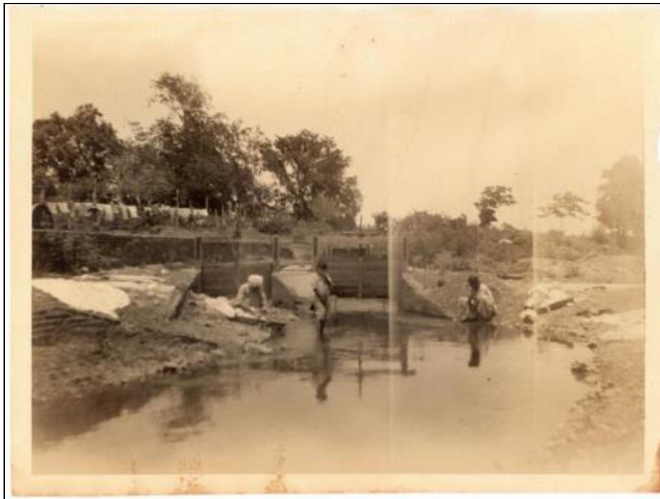
Photo of the main intake for the Florida, Santa Isabel and Destino Haciendas or Tres Haciendas at the junction of the main canal and the Coamo river, 1913, AAA (from Meléndez Maíz 2011).
