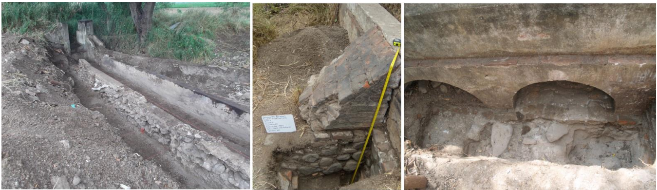
Left; view of the Hacienda Florida channel at its origin as it left the distribution module, facing northeast. Center; Detail of an abutment. Right; segment of the channel on arches. Note the stone pavement under the channel.
