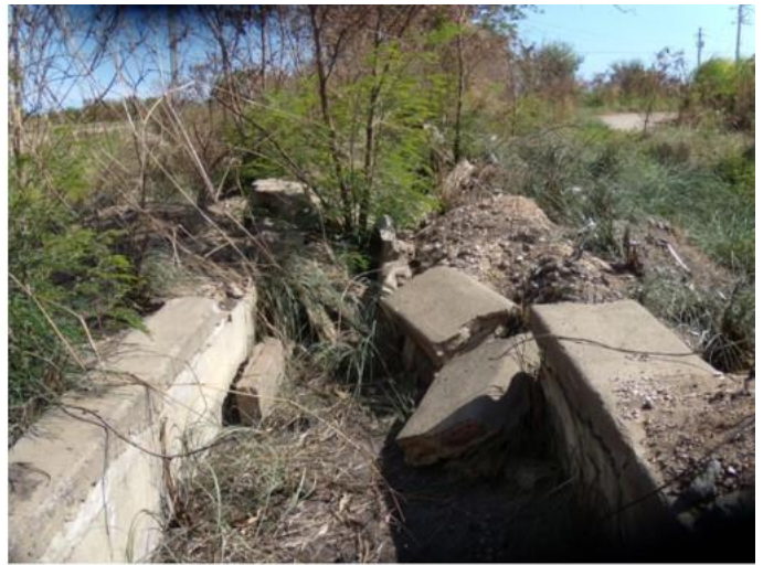
On the left, collapsed section of the torrential waters inlet channel, looking southwest. On the right segment of the supply channel with side impact caused by agricultural machinery.
