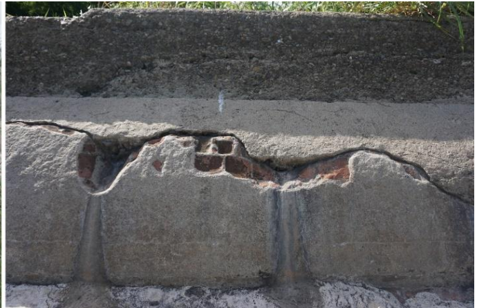
On the left, view the central area of the dam with the added opening for the sluice, seen upstream from the east bank. On the right; detail of the two construction phases of the structure: lower part built from brick masonry in the 19th century, and 20th century upper part of reinforced concrete.
