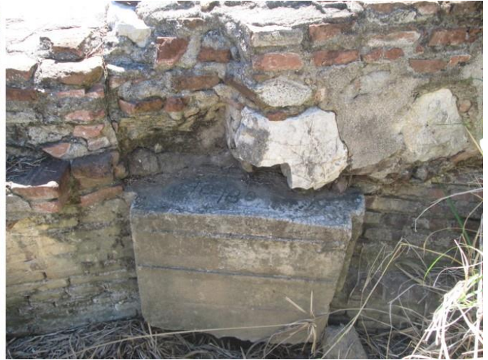
Repairs with date inscriptions. On the left, repair on the supply channel dated 1961 and to the right, repair to the low and torrential waters modules, dated 1980.
