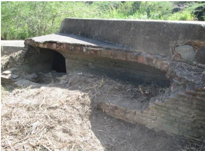
On the left, collapsed section of the torrential waters inlet channel, looking southwest. On the right segment of the supply channel with side impact caused by agricultural machinery.
