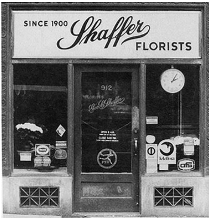
The original form and features of this 1920s storefront have been retained through Preservation. Photo: David W. Look, AIA.
