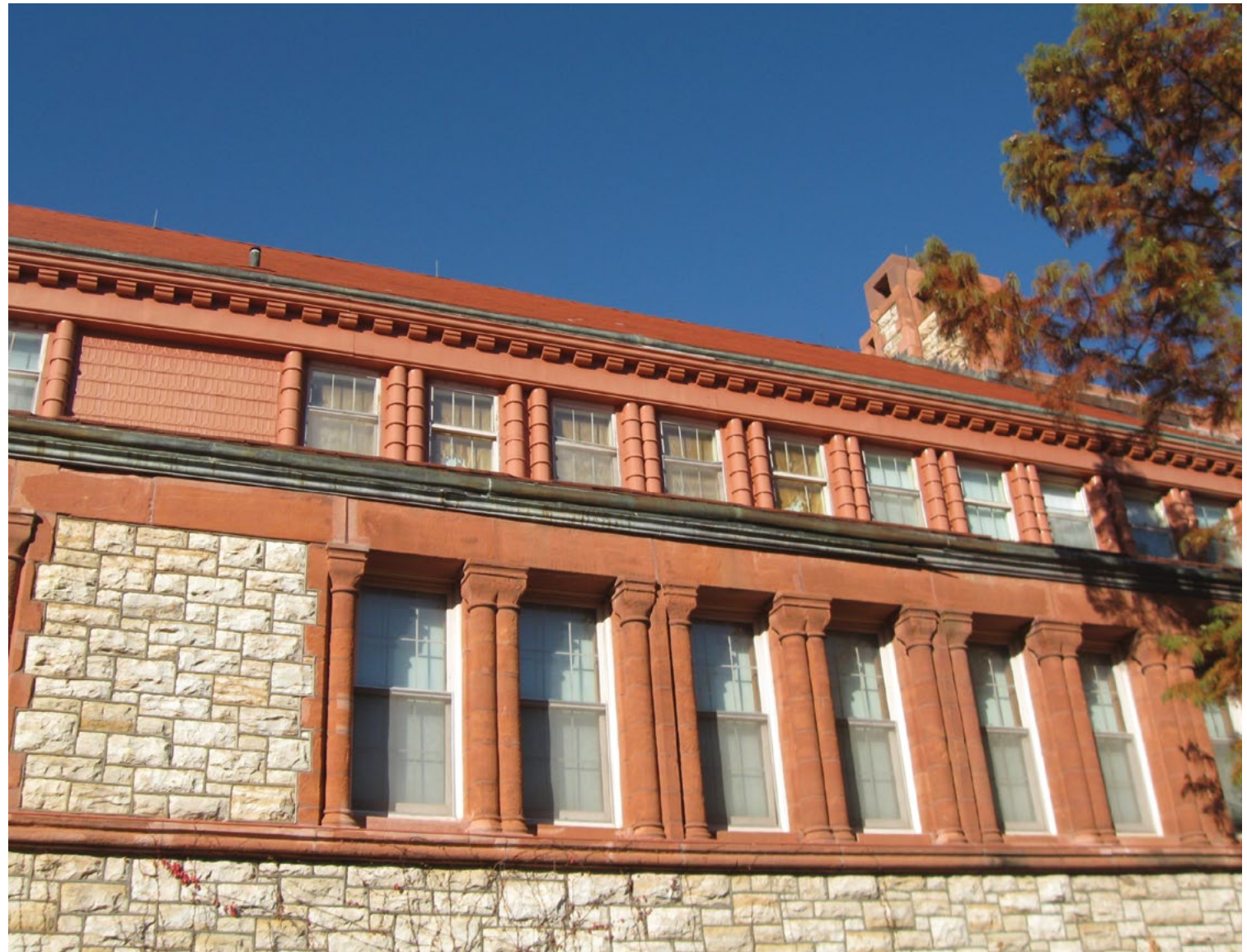
[6] Preliminary work before starting restoration revealed that the columns and the decorative shingles ornamenting the top floor of this historic building were fabricated of metal to imitate the red sandstone used elsewhere on the building.
