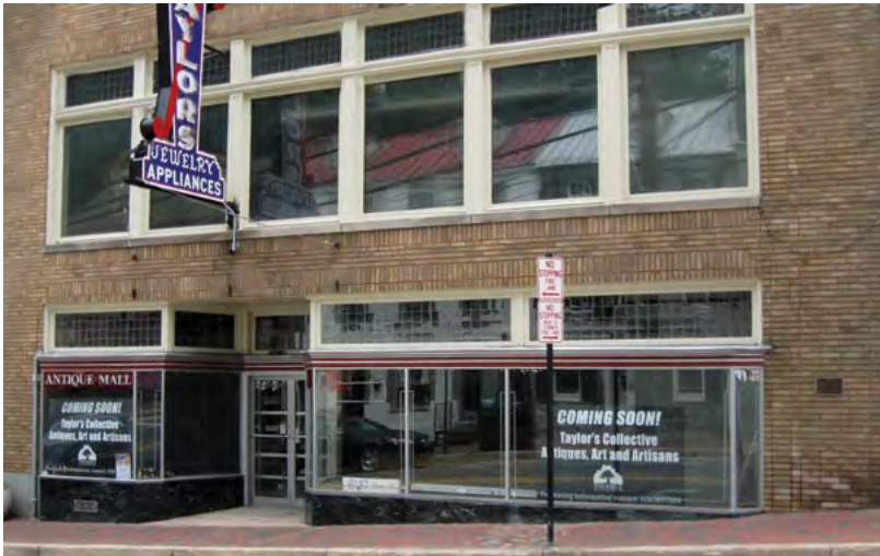
[15] Regular maintenance has helped to preserve this historic storefront, which retains all of its character-defining features, including the granite bulkhead, multi-paned transom glazing, and recessed entrance.
