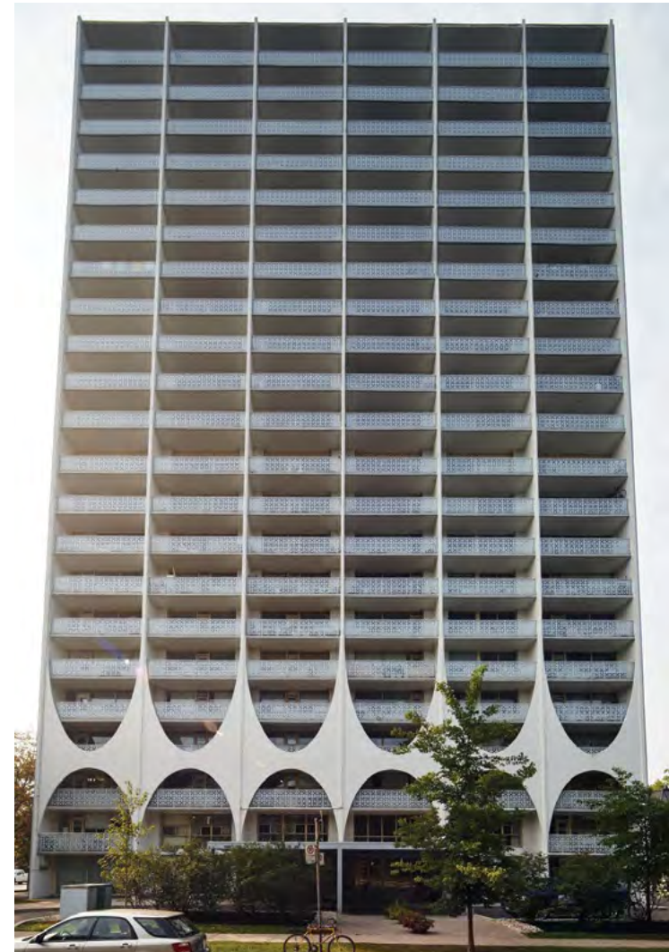
[59] (a-b) The decorative concrete balcony railings on this 1960s building did not meet life-safety code requirements. They were replaced with new glass railings with a fritted glass pattern matching the original design—a creative solution that satisfies codes, while preserving the historic appearance of the building when viewed from the street (c-d). Photos: (a, b, d) ERA Architects, Inc.; (c) Nathan Cyprys, photographer.
