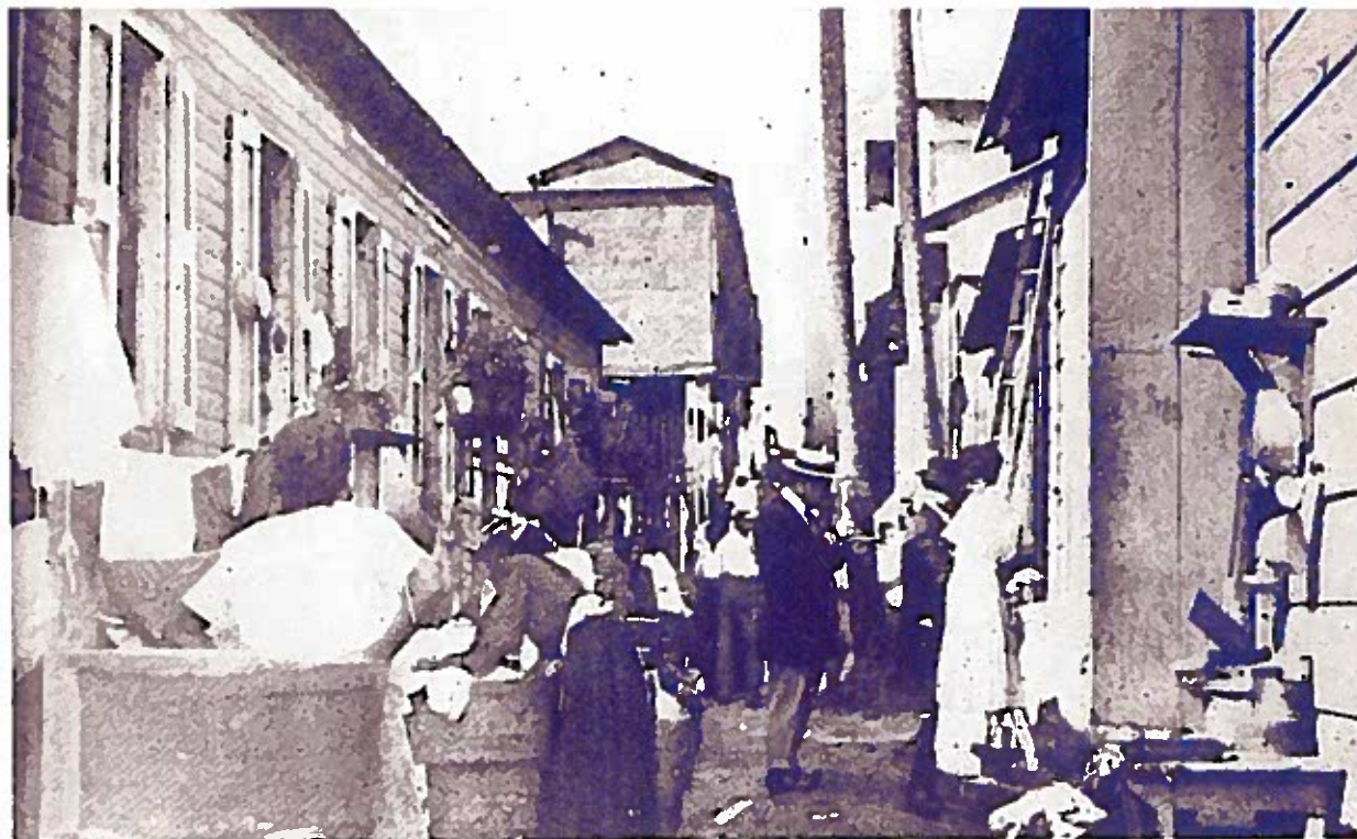
RANCHONES, 1914 J.C. Bills, Housing Conditions of Laborers in Puerto Rico , 1914.
