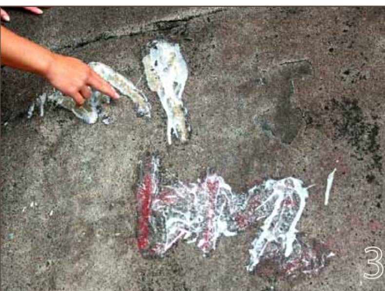
Lift-off can be applied via spray or paste to remove acrylic or enamel paint.
