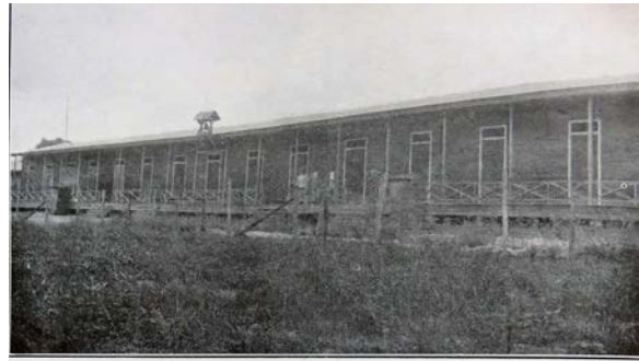
PLAYA SCHOOL, MAYAGUEZ. TEMPORARY FRAME BUILDING ERECTED AFTER EARTHQUAKE.
