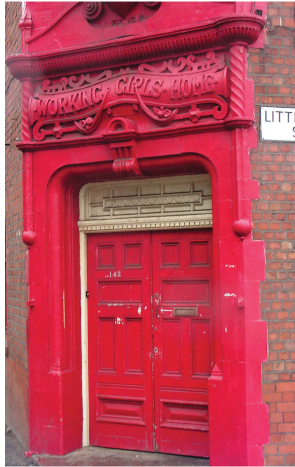
Main entrance, Charter Street Home for Working Girls. Photo by G. Marino
