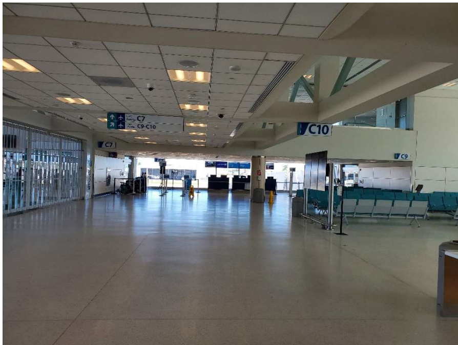
Ilustración 11: "Replace Deteriorating Flooring" – Final del Terminal "C"
