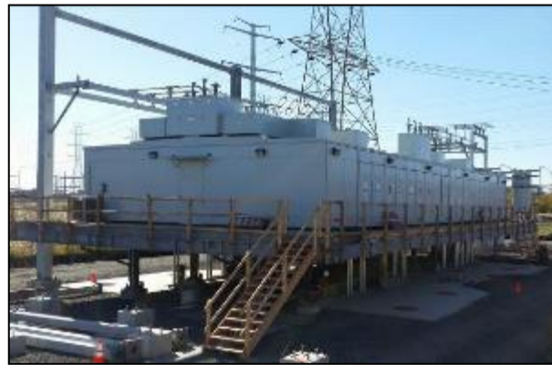
Figure 1.4.17 PSE&G Raised Switching Station
