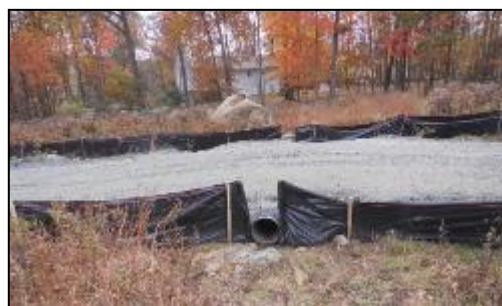
Figure 1.4.27 Wildlife Crossing Installed Along a Construction Access Road
