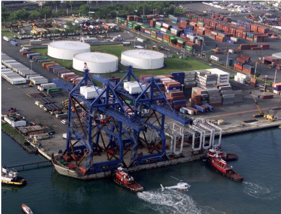
Figure 2. Wharves N and O receive container, general, and liquid cargo, including a connection to purpose-built storage tanks supporting a major distiller operating on the Island.
