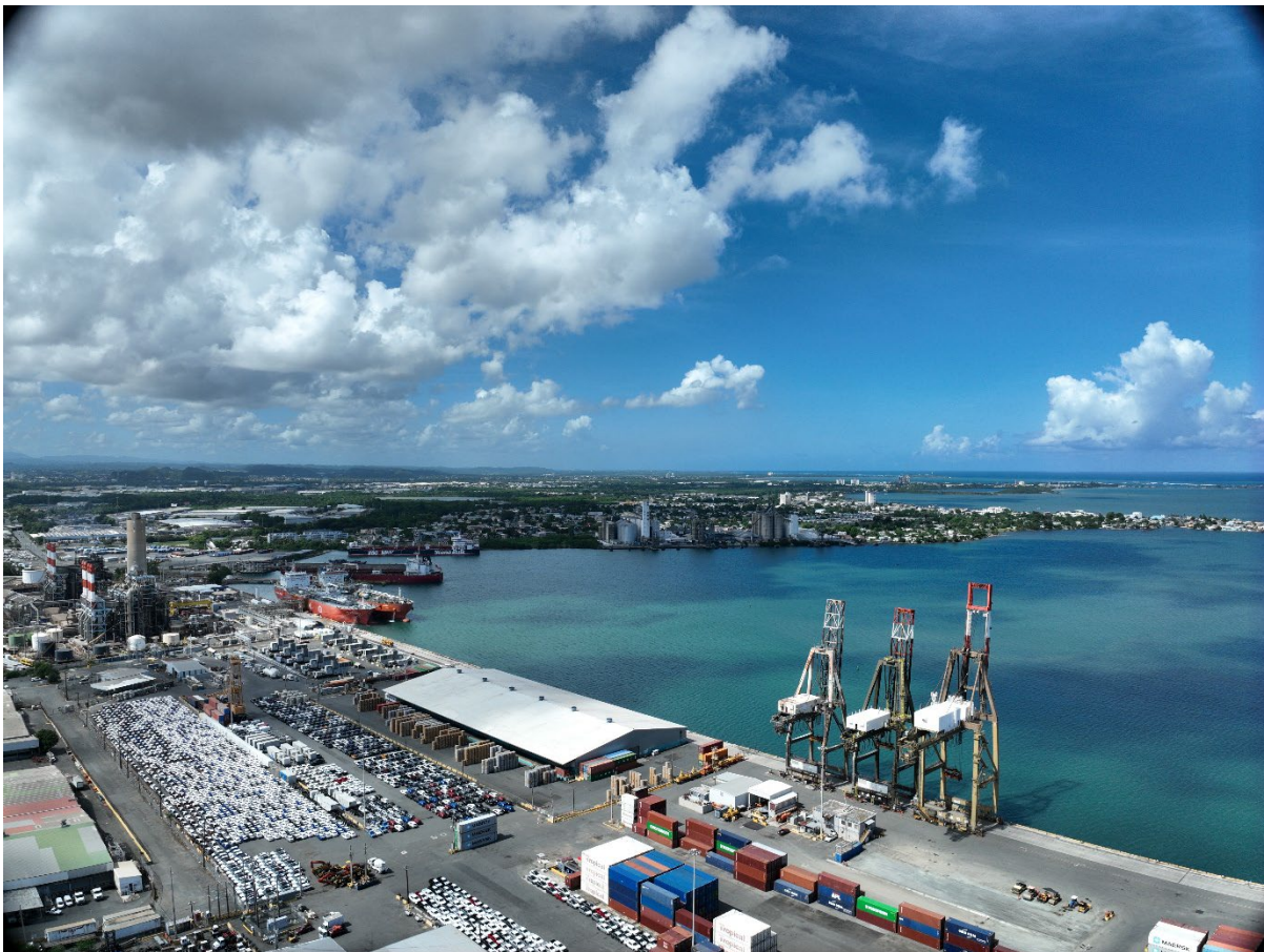
Figure 1. Wharf D at Puerto Nuevo houses a warehouse to store a variety of temperature-sensitive breakbulk cargo and automobiles.
