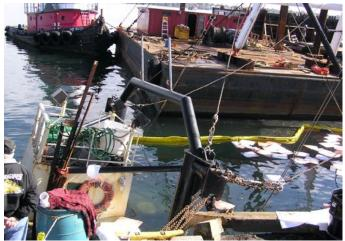
An abosorbent boom and fuel pads placed in water to collect oil released from a sunken boat. Photo credit: Massachusetts DEP.
