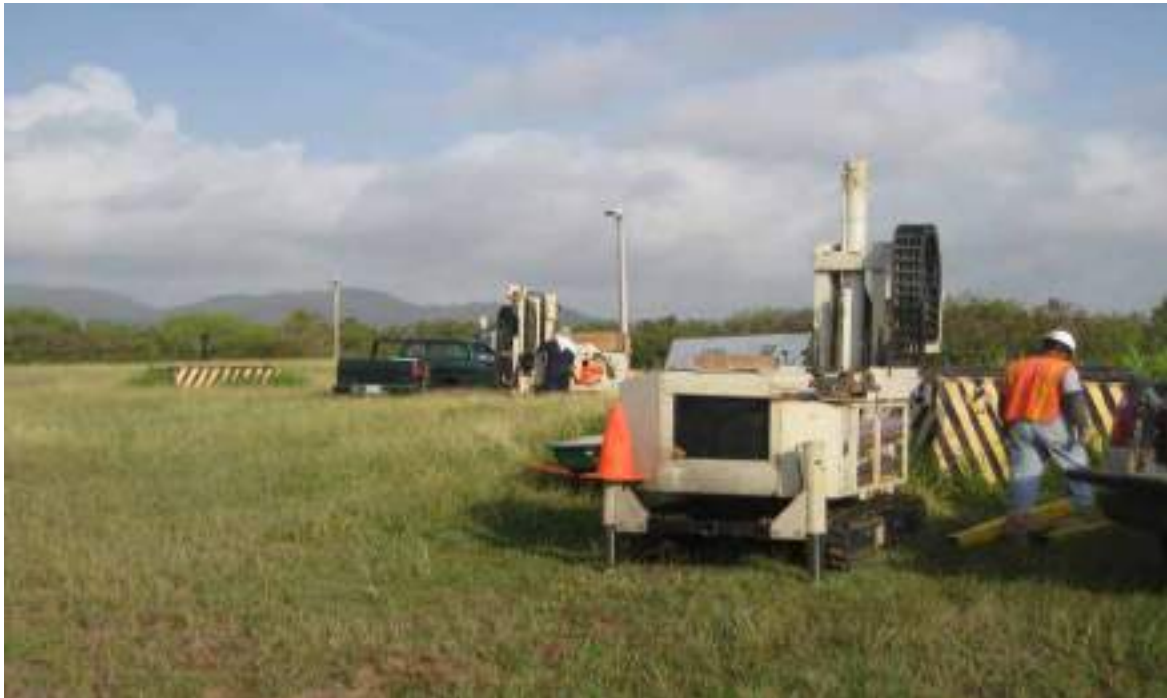
JFA Environmental Associates and GeoEnviroTech drillers both installing a groundwater monitoring well using a GeoProbe® Tracked Direct Push Machine at SWMU 9 A-B Area
