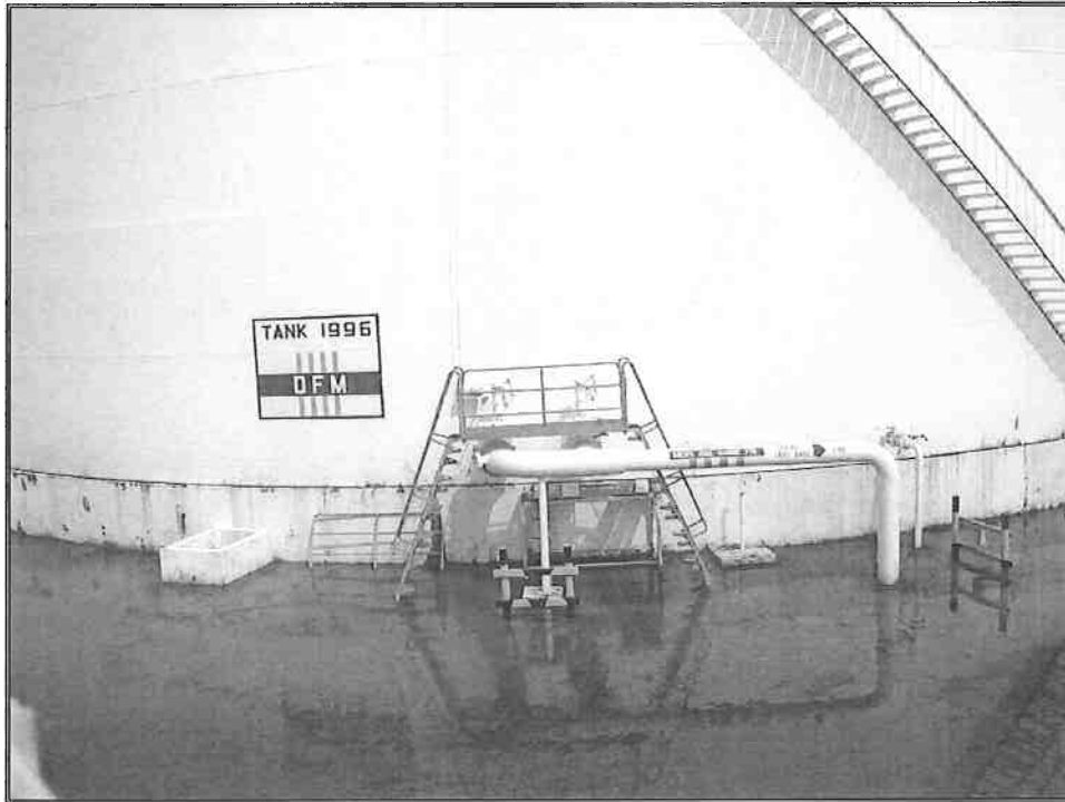
Photograph No. 27 – Test No. 12 DFM Tank 1996
