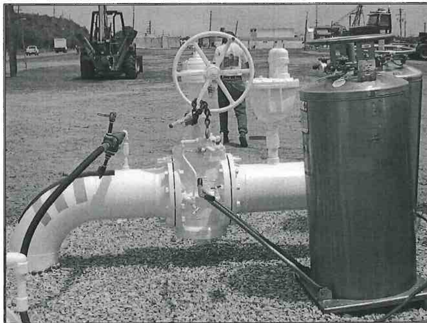
Photograph No. 44 – Nitrogen and SF6 Injection for Leak Detection
