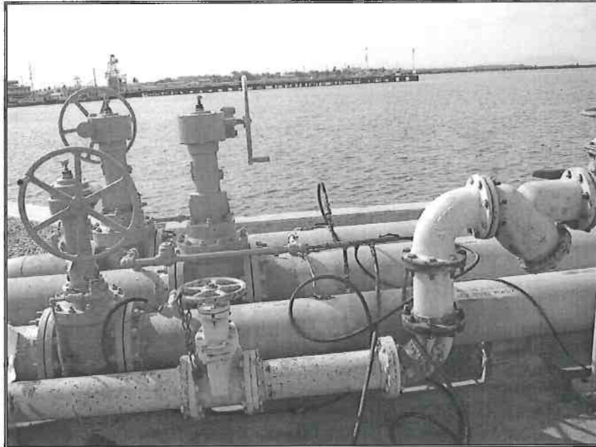
Photograph No. 1 – Test No. 1 Pier 1 Test Location
