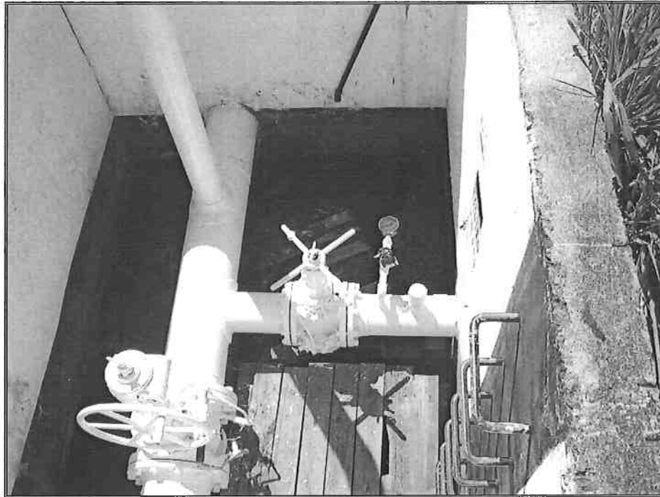
Photograph No. 21– Test No. 10 Test Location
