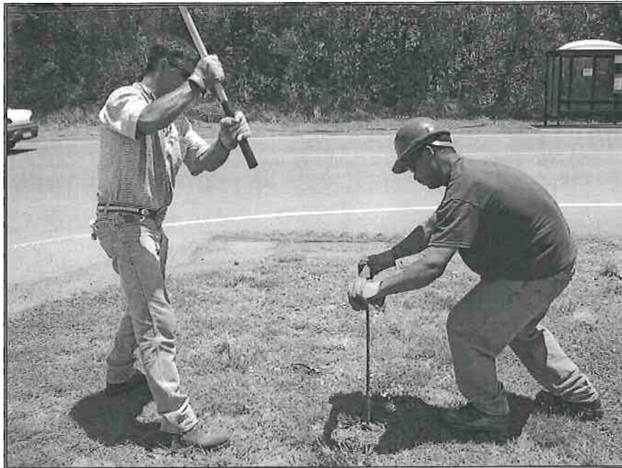
Photograph No. 43 – Leak Detection Probe Holes
