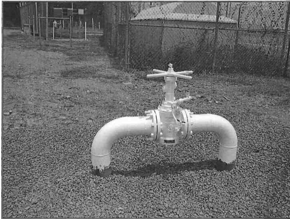
Photo 15E – VP 56 Valve Setting Installation DFM Pipeline
