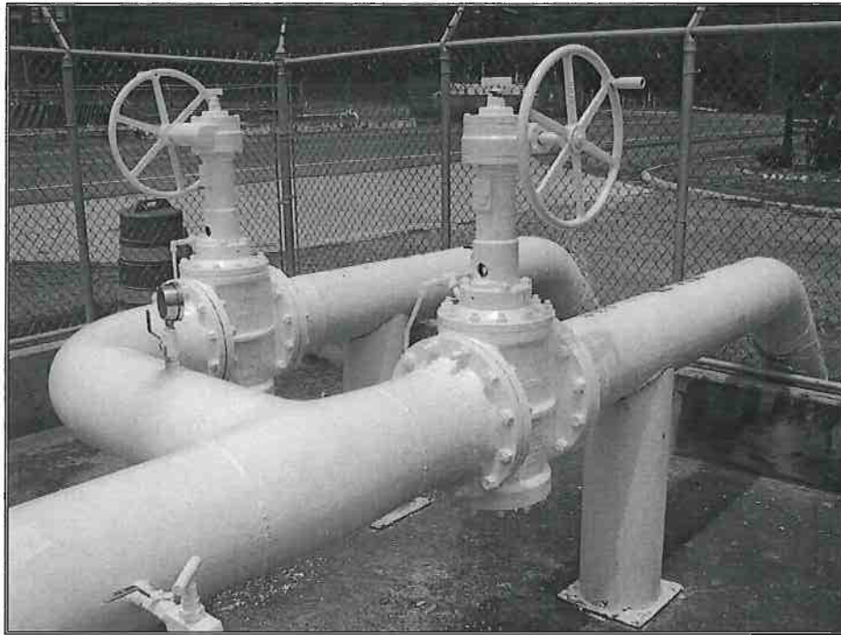
Photo 8A – PH 466 Valve Installations DFM-S Pipelines
