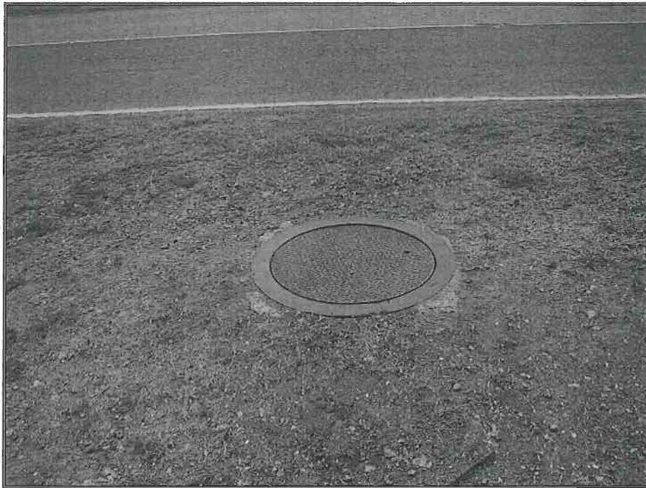
Photo 16A – Blow Out Pit Removal JP-5 Pipeline
