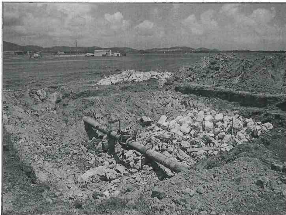
Photo 13C – VP 4 Valve Removal JP-5 Airfield Pipeline
