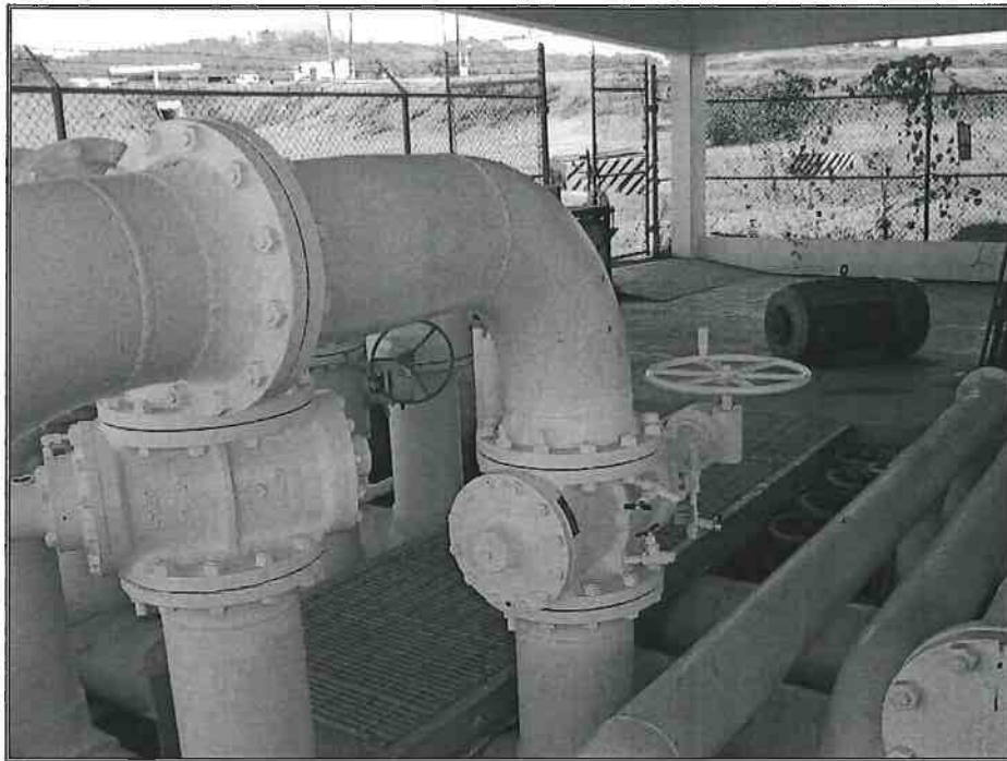
Photo 15A – PH 1982 Valve Installation
