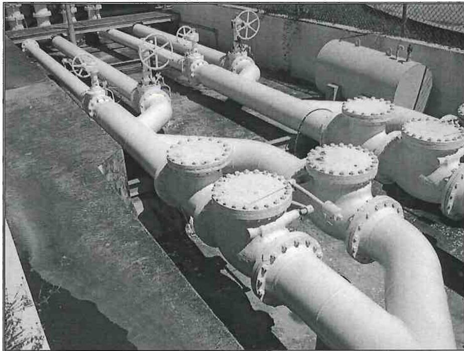
Photo 15D – PH 1982 Valve Installation and Meter Run Removal
