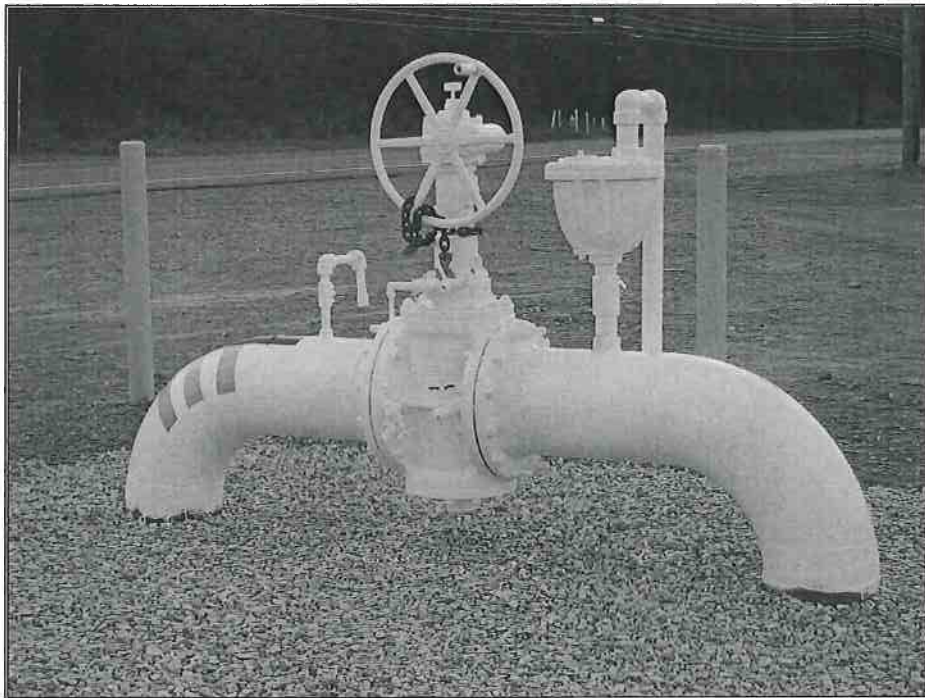
Photo 10D – VP 24 Valve Setting Installation JP-5 Pipeline to Pier 3
