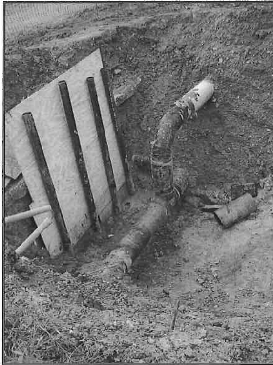
Photo 20A – Valve TFD-141 Removal DFM Pipeline
