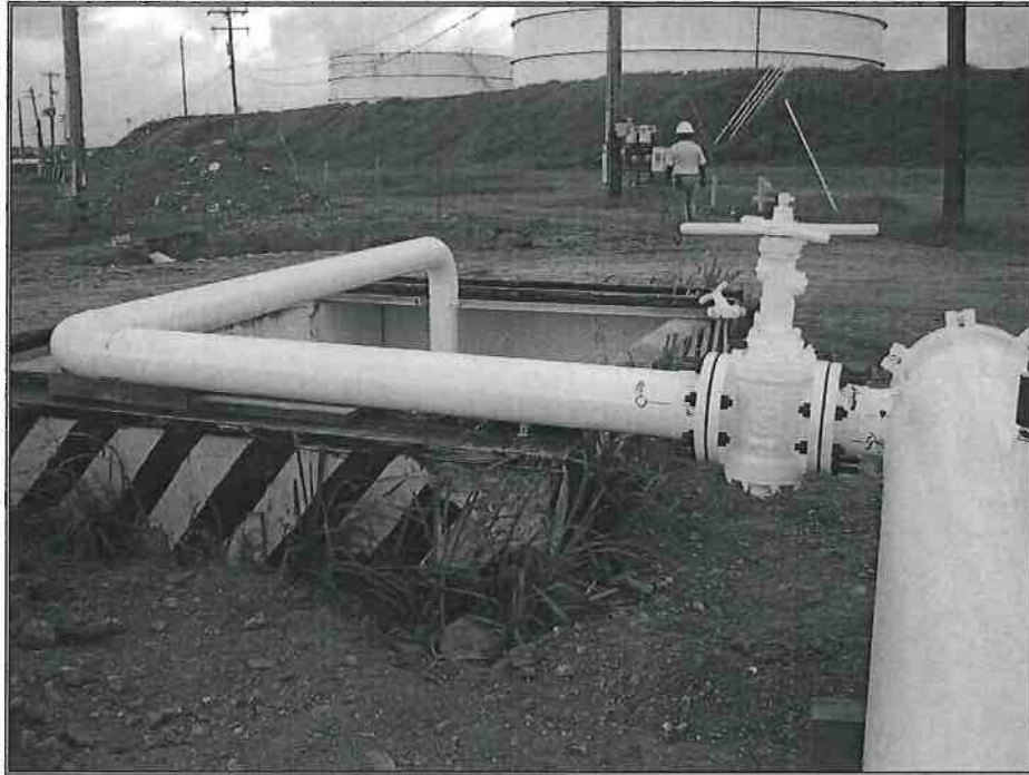
Photo 22D – VP 9 Pig Trap Installation JP-5 Pipeline
