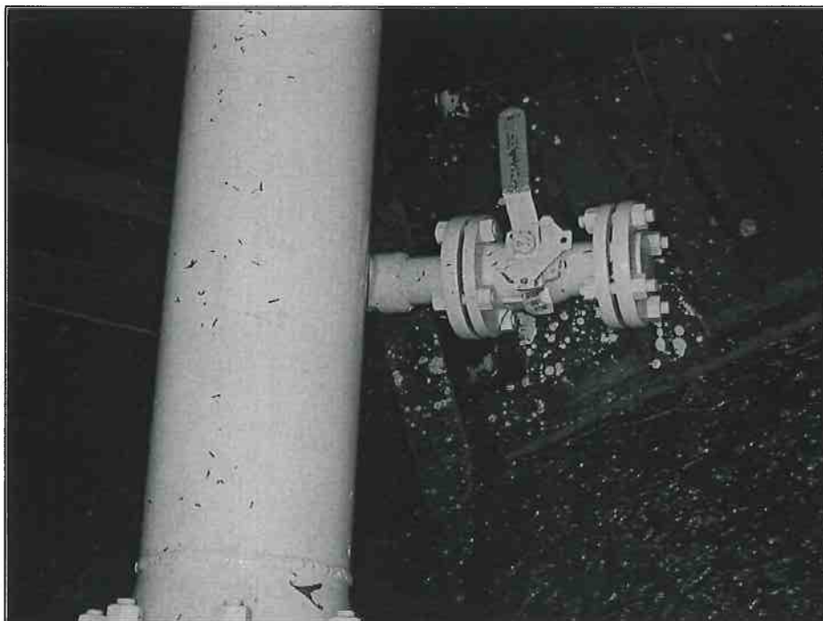
Photo 13G – VP 6 Drain Valve Installation JP-5 Airfield Pipeline
