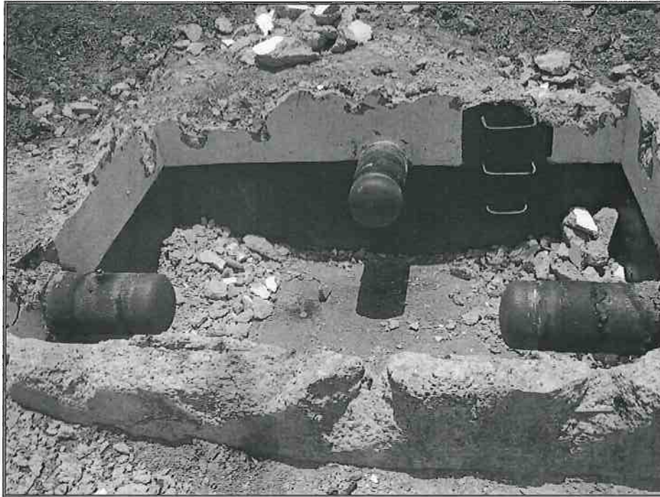
Photo 12A – VP 6 Valve Removal DFM-S Pipeline
