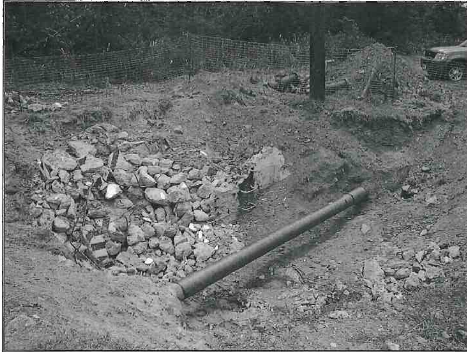
Photo 13D – VP 5 Valve Removal JP-5 Airfield Pipeline
