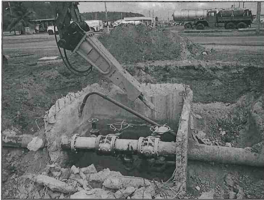
Photo 7A – Valve Pit 25 Valve Removal DFM-S Pipeline
