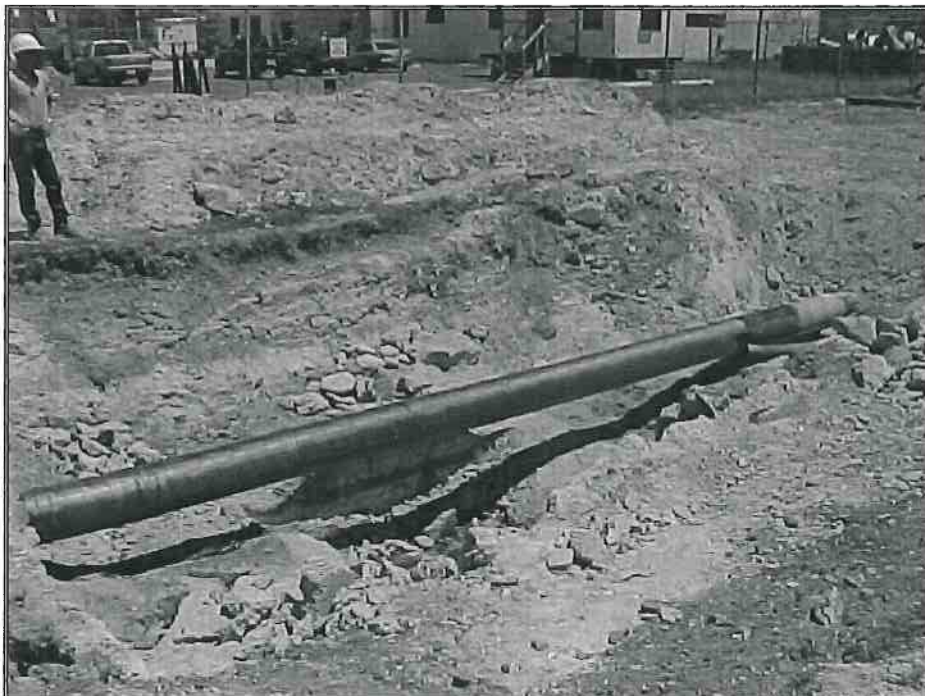
Photo 7B – Valve Pit 25 Valve Removal DFM-S Pipeline
