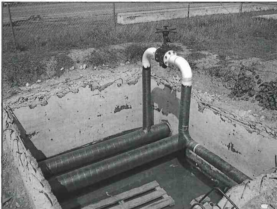
Photo 15F – VP 56 Valve Setting Installation DFM Pipeline
