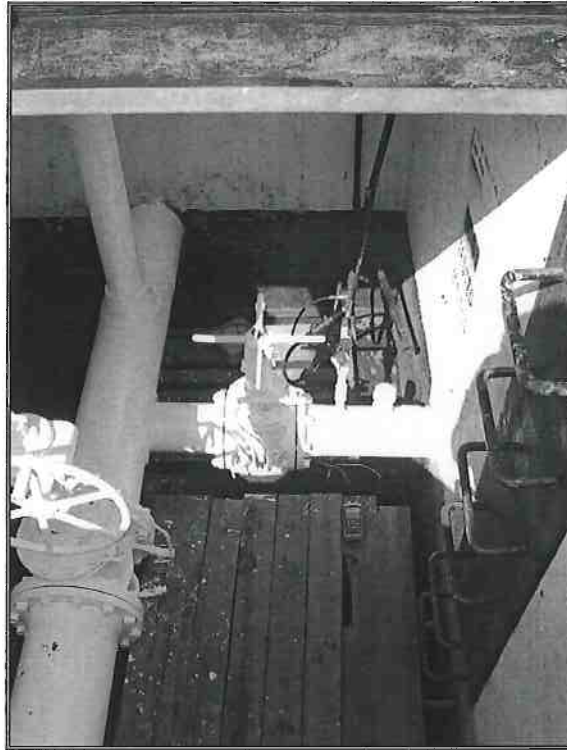
Photo 14A – VP 9 Valve Replacement JP-5 Pipeline
