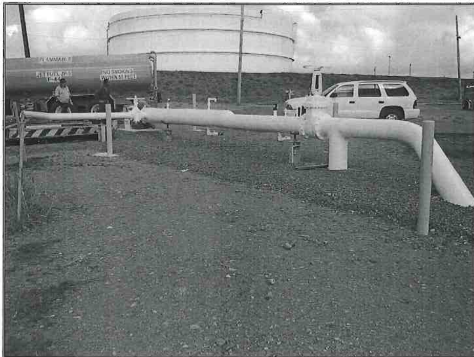
Photo 22A – VP 9 Pig Trap Installation JP-5 Pipeline
