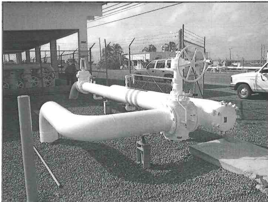
Photo 21A – PH 1982 Pig Trap Installation JP-5 Pipeline
