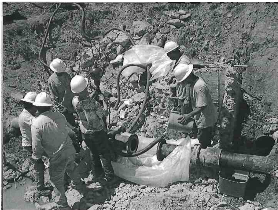
Photo 13D – VP 5 Valve Removal JP-5 Airfield Pipeline
