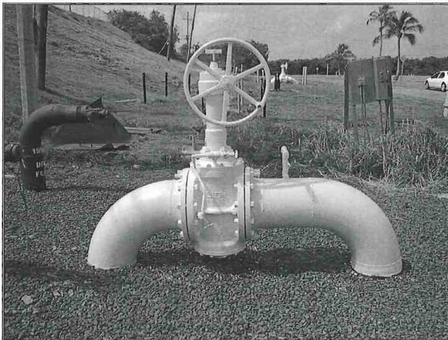
Photo 19B – Valve Pit 8 Valve Setting Installation DFM Pipeline
