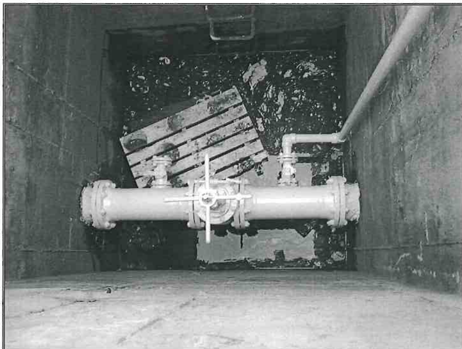
Photo 13A – VP 3 Valve Removal JP-5 Airfield Pipeline
