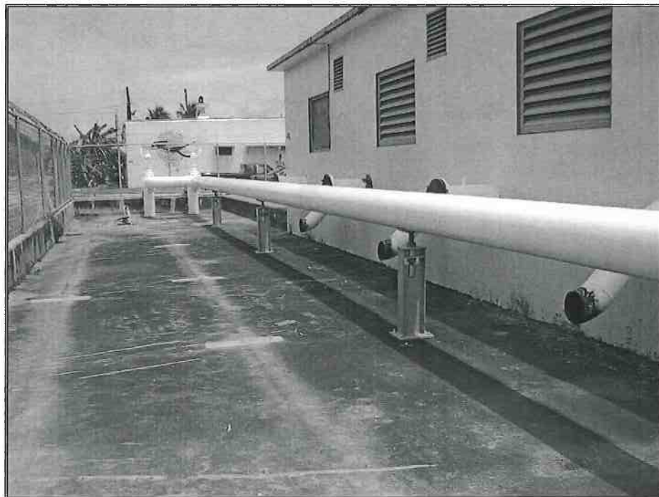
Photo 8B – PH 466 Pipe Installation DFM-S Pipeline
