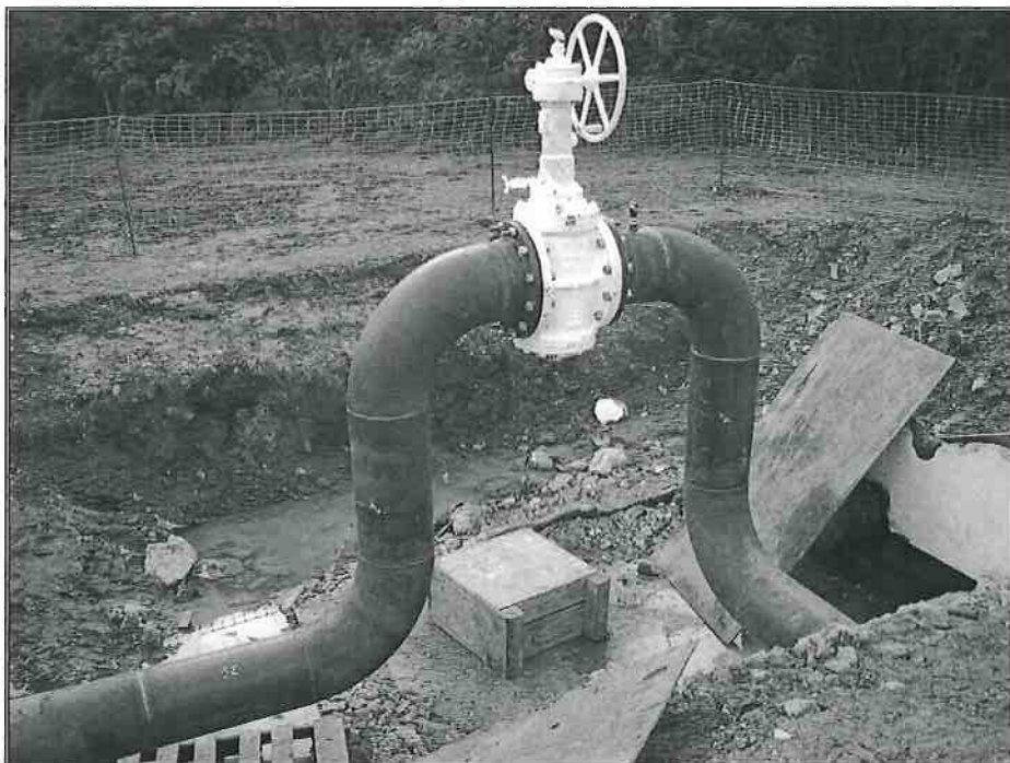
Photo 11B – VP 8 Valve Setting Installation DFM-S Pipeline
