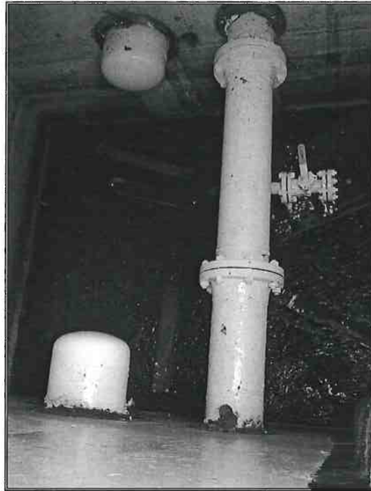
Photo 13F – VP 6 Valve Removal JP-5 Airfield Pipeline
