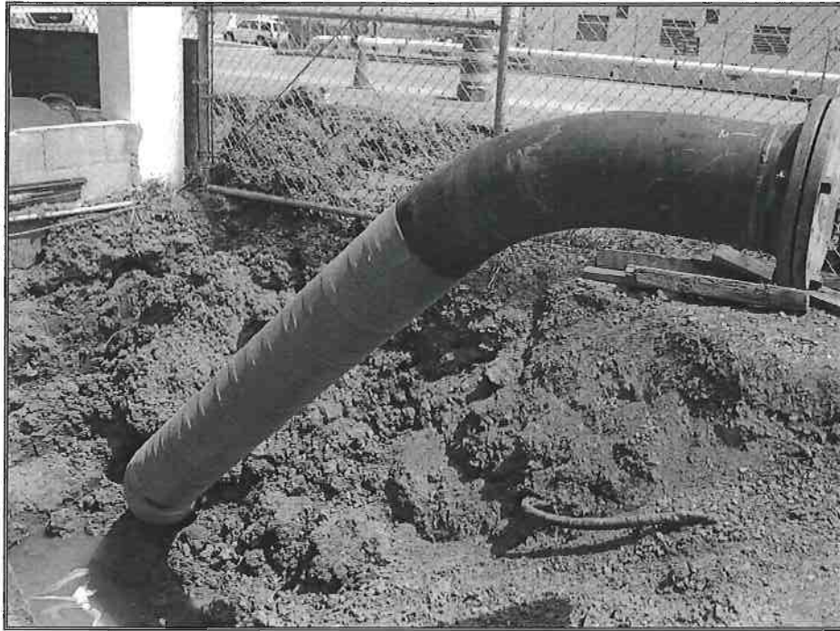
Photo 21D – PH 1982 Pig Trap Installation JP-5 Pipeline
