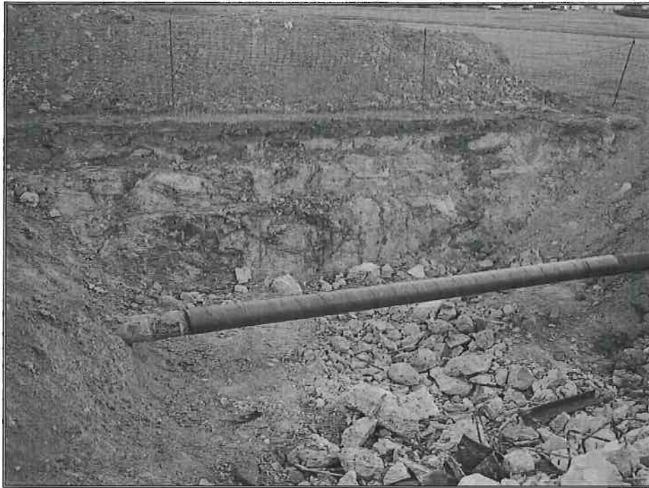
Photo 13B – VP 4 Valve Removal JP-5 Airfield Pipeline
