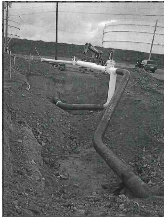
Photo 22B – VP 9 Pig Trap Installation JP-5 Pipeline
