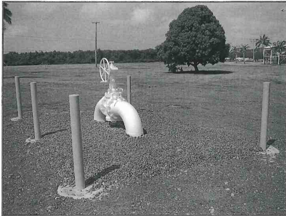
Photo 11A – VP 8 Valve Setting Installation DFM-S Pipeline
