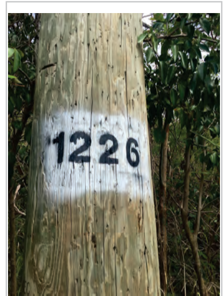
Photo 1: Pole Identification
