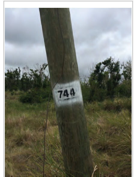
Photo 1: Pole Identification
