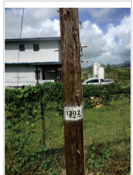
Photo 1: Pole Identification
