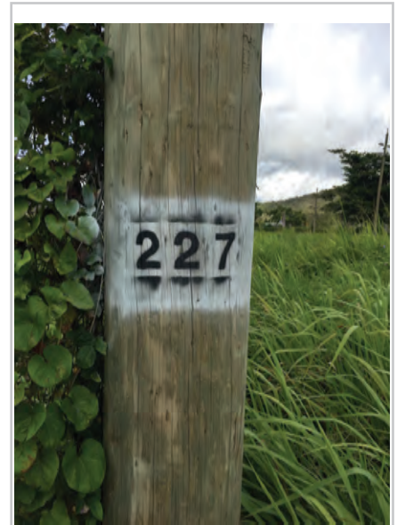
Photo 1: Pole Identification
