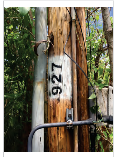
Photo 1: Pole Identification
