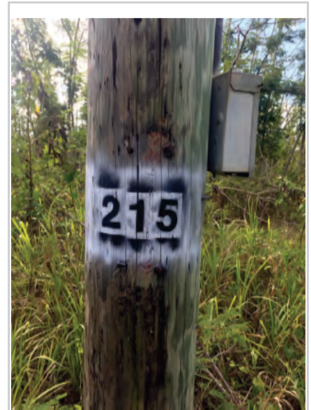
Photo 1: Pole Identification
