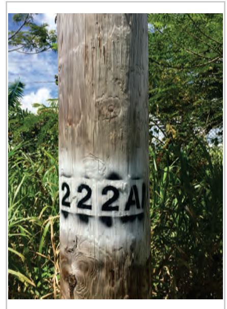
Photo 1: Pole Identification
