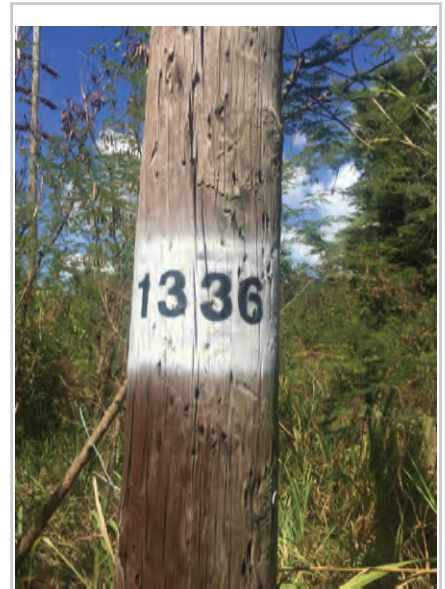
Photo 1: Pole Identification
