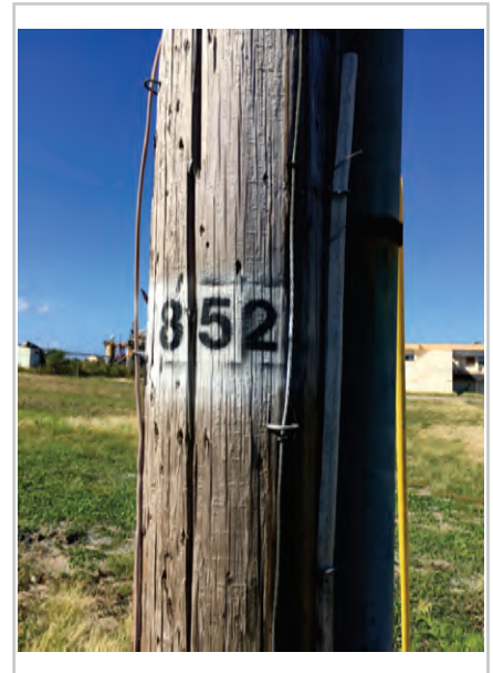
Photo 1: Pole Identification
