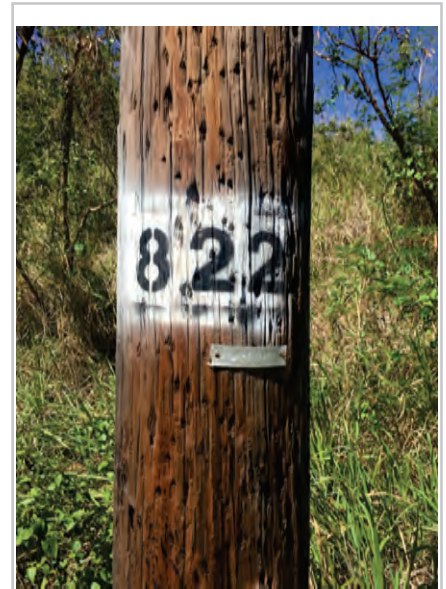
Photo 1: Pole Identification
