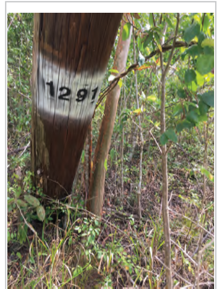
Photo 1: Pole Identification
