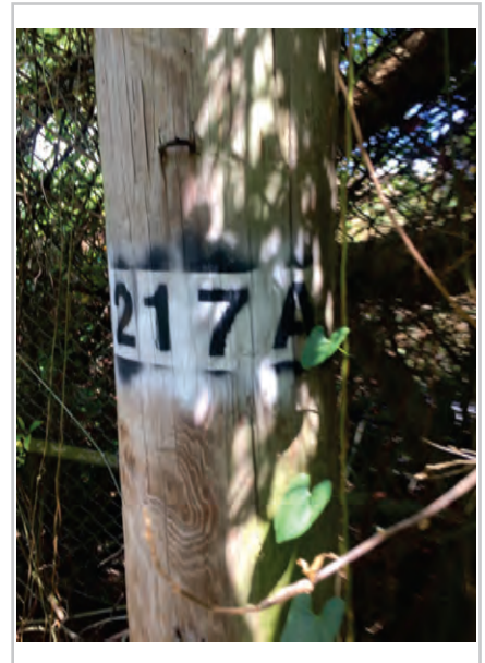
Photo 1: Pole Identification
