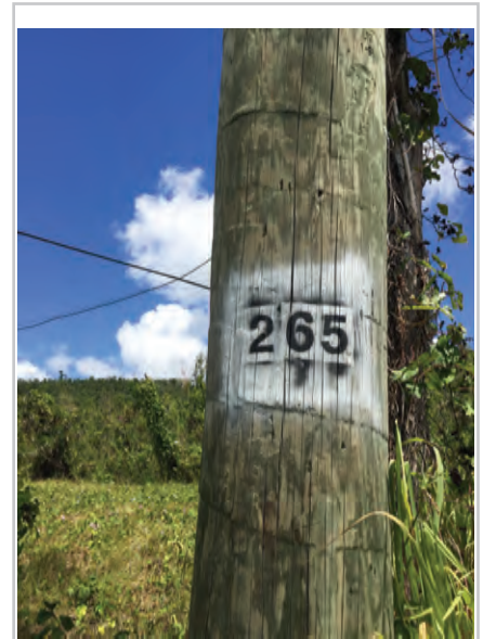
Photo 1: Pole Identification
