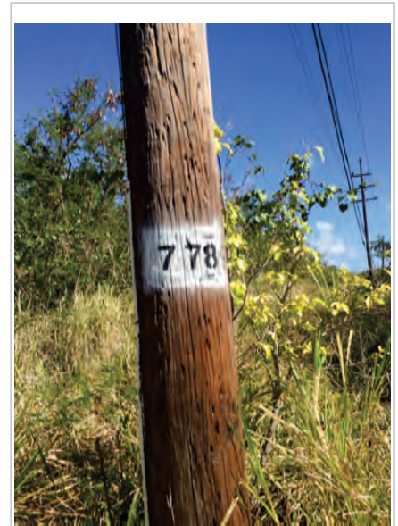
Photo 1: Pole Identification
