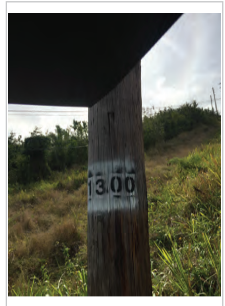
Photo 1: Pole Identification
