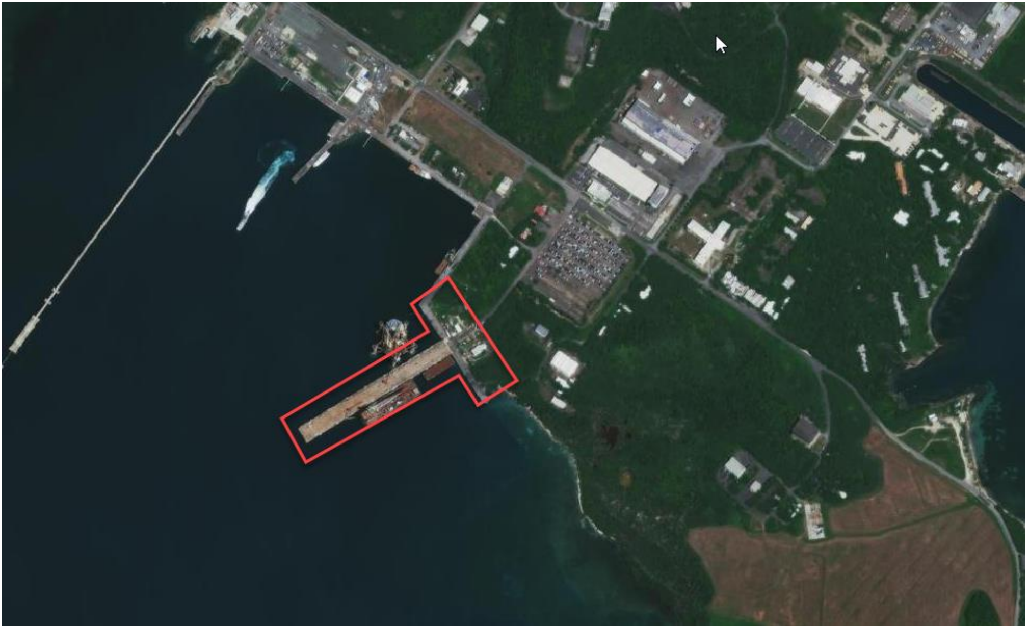
Exhibit B-3 - Pier 3 & Bulkhead D 1 of 2 Roosevelt Roads
