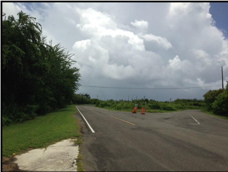
View of access roads within NSRR.
