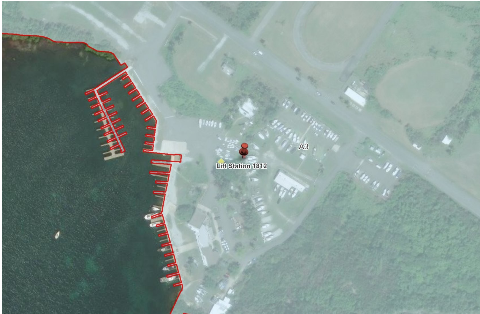
Figure 3. Lift Station 1812 – Parcel FOSL – SWMU 60 (U.S. Government), Subzone A3
