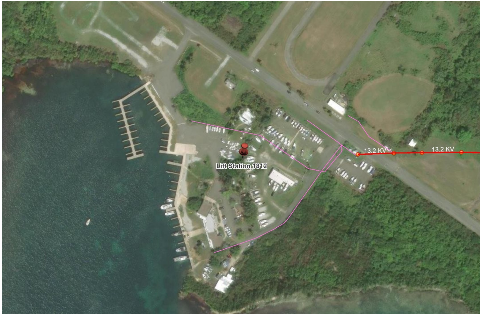
Figure 2. Lift Station 1812 – Electric Power Lines (for reference only)
